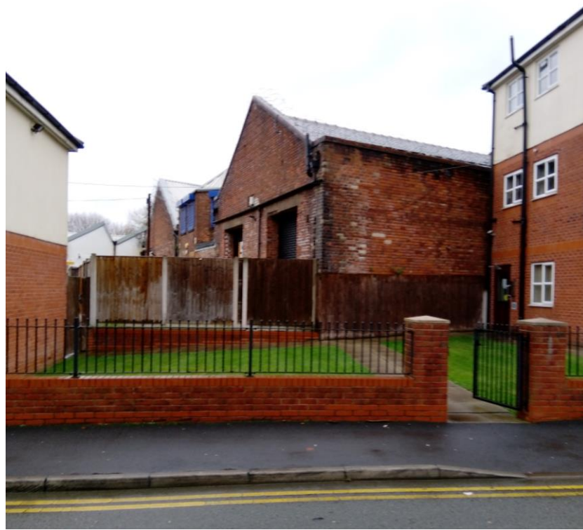
Fig. 2 – Views of the site from Hamsell Road.
