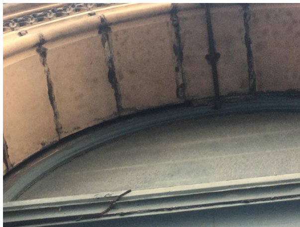
PLATE 2 SHOWING POTENTIAL ROOST FEATURE ON NORTHERN ASPECT OF B1
