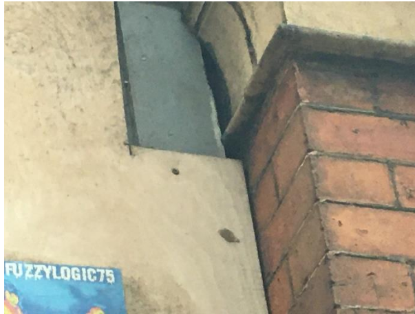
PLATE 3 SHOWING POTENTIAL ROOST FEATURE ON EAST ASPECT OF B1
