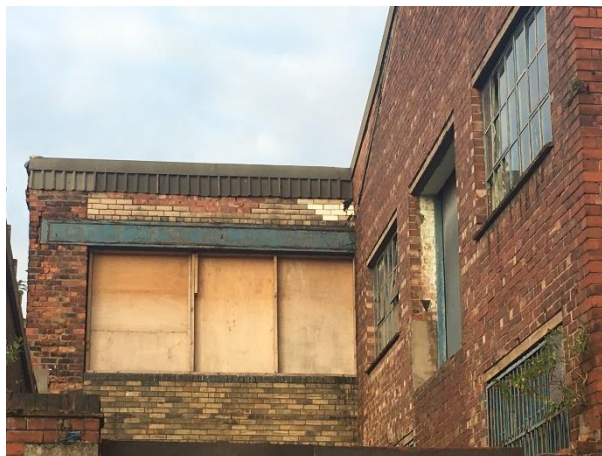
PLATE 4 SHOWING HANGING TILES AND FACIAS
