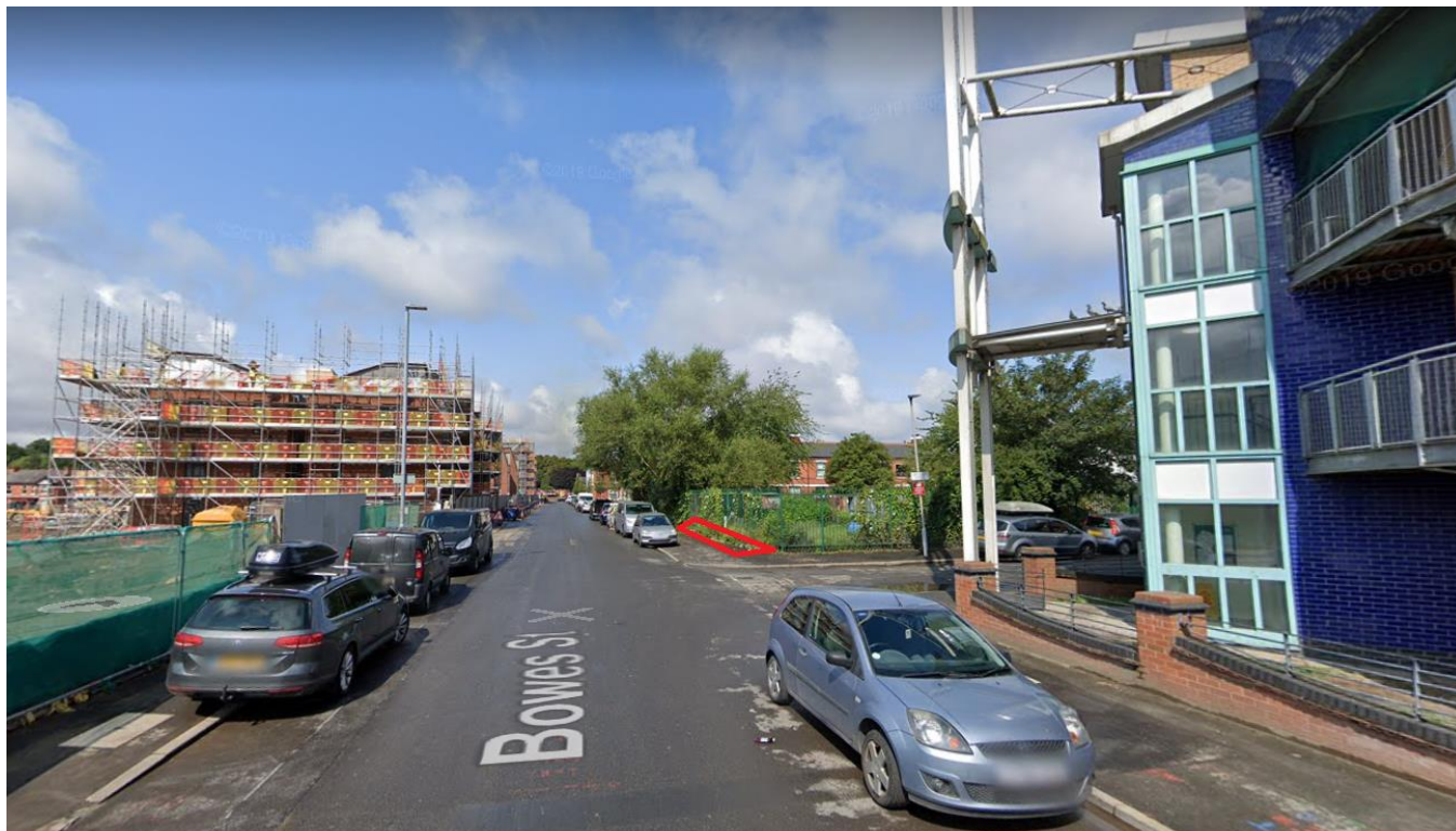
View west along Bowes Street with application site edged red
