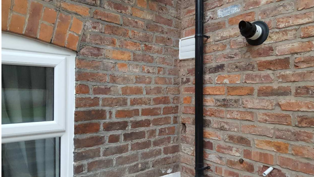
Original rear elevation/new rear extension brickwork junction (above)
