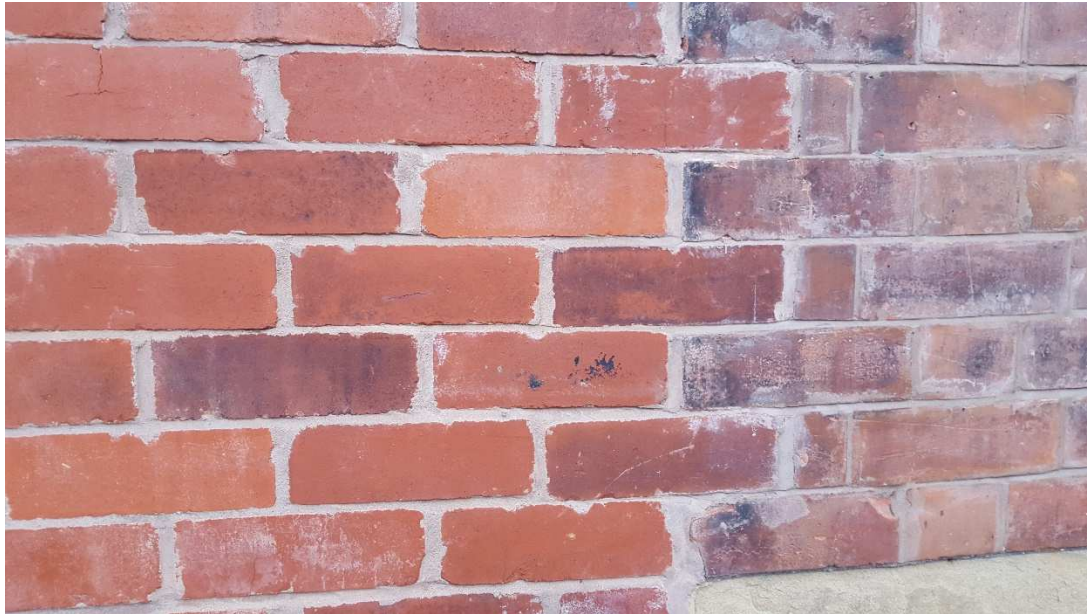
Front elevation junction between new and existing construction
