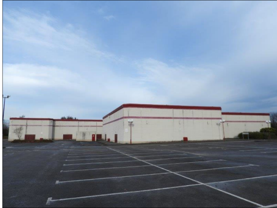
Plate 17. Showcase Cinema (southern elevation)
