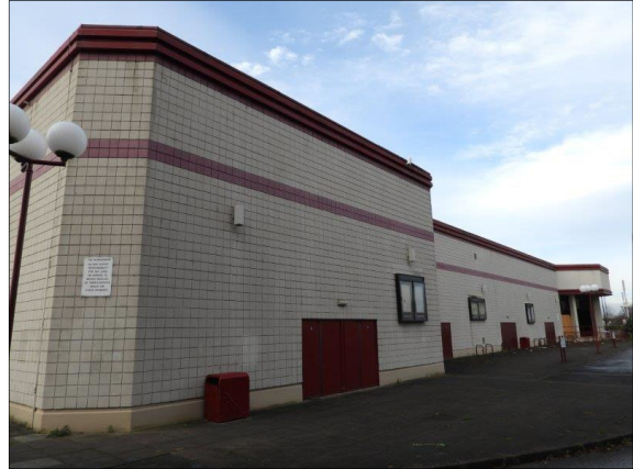
Plate 18. Showcase Cinema (north-east elevation)
