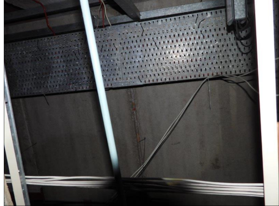
Plate 34. Showcase Cinema (concrete roof)
