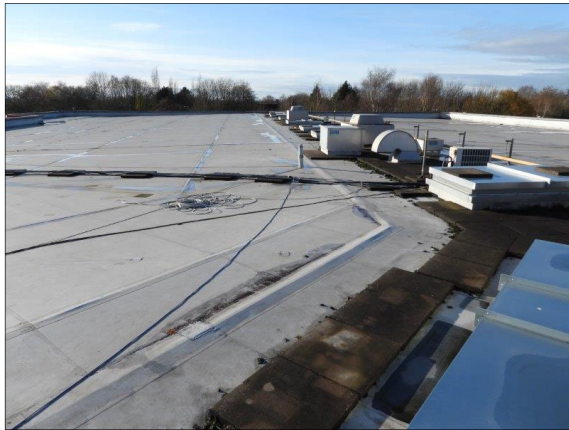
Plate 27. Showcase Cinema (metal gutter-boxing)
