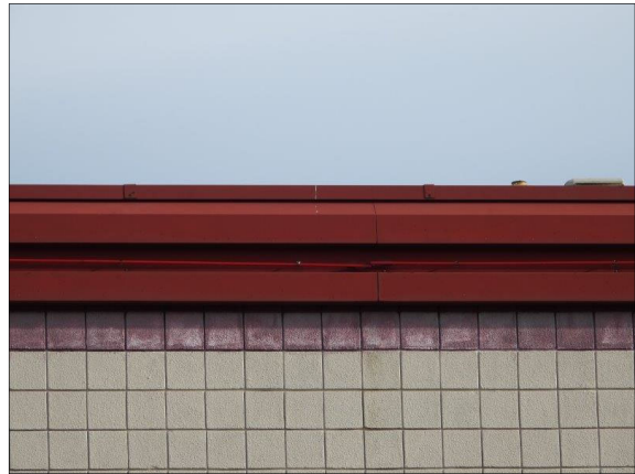
Plate 28. Showcase Cinema (metal gutter-boxing)
