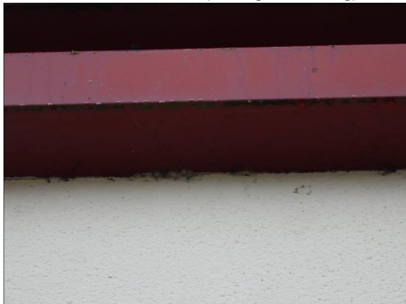
Plate 27. Showcase Cinema (metal gutter-boxing)
