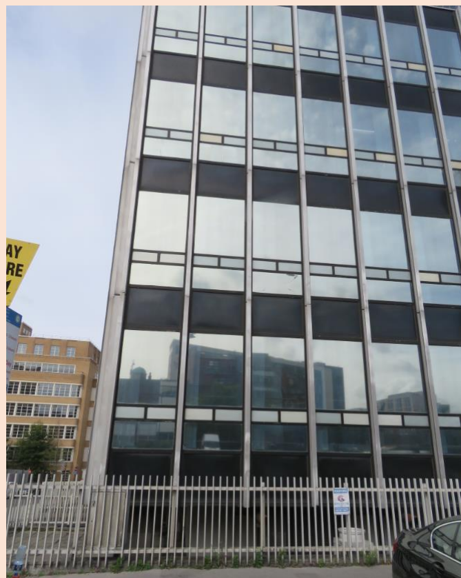
RS-08 Looking west showing the corner of the Riga Street podium elevation.
