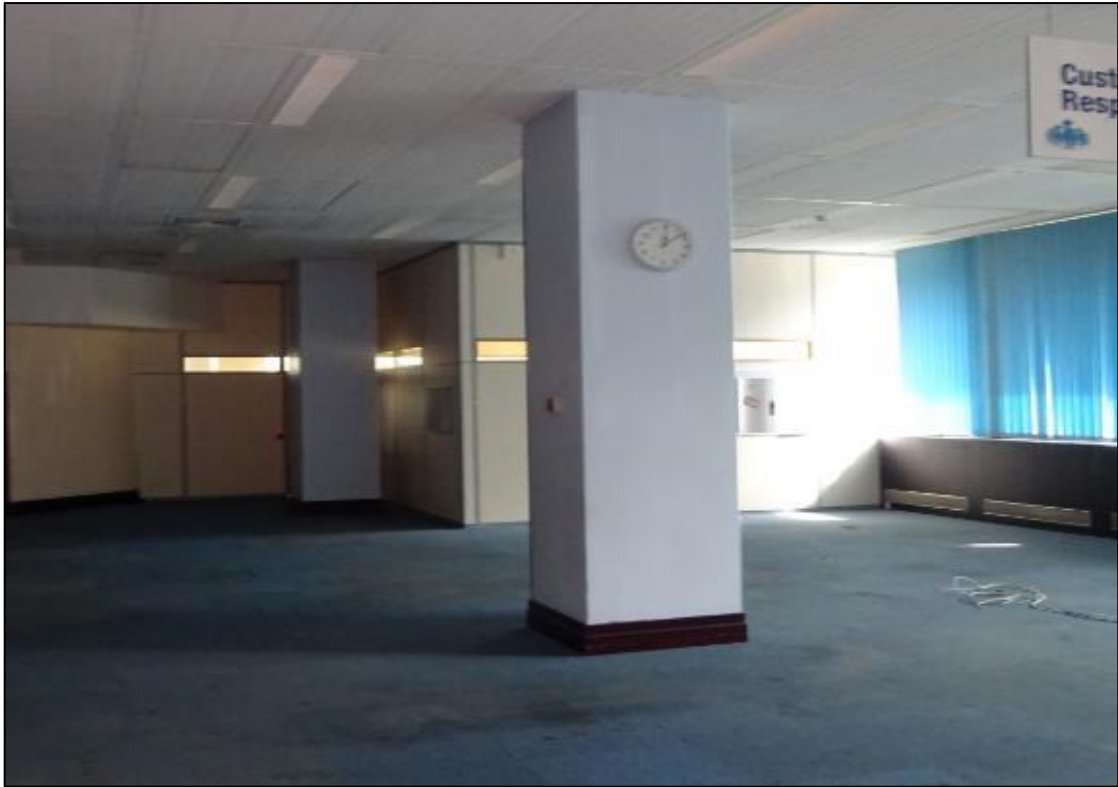
Figure 20. Typical Podium floor office space (Level 04 – Appendix 10 ) all fabric components shown (ceilings, floors, cladding to columns) are non-original.
