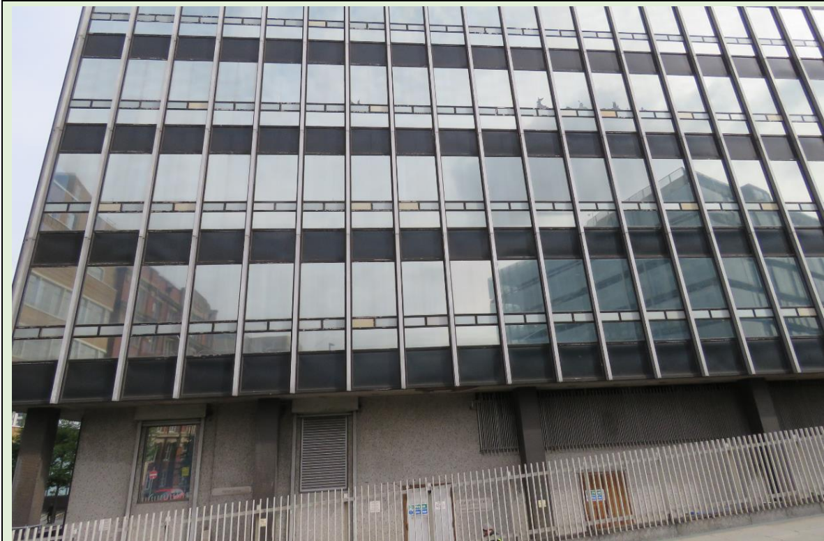
HS-03 Details showing the over-hang, service area, railings and the eastward rise of Hanover Street.
