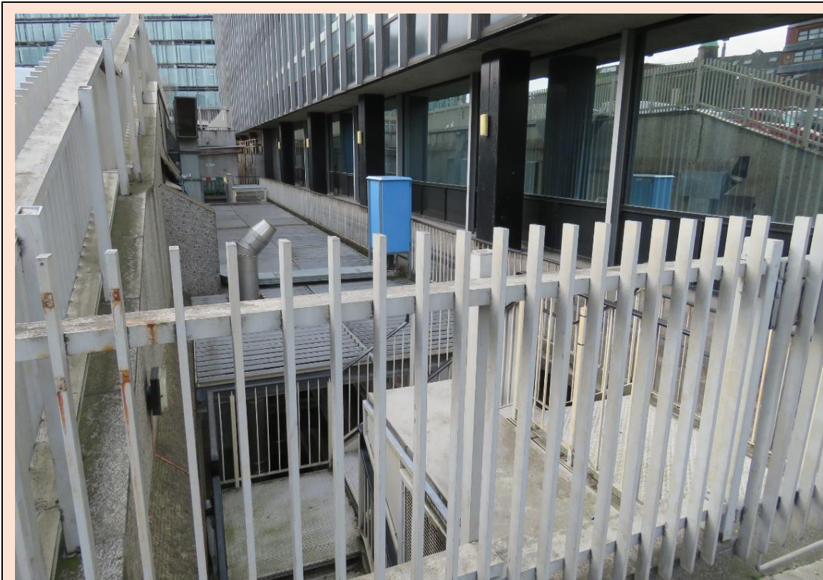
RS-03 Looking south into the plant basement, showing the square-section railings and retaining walls.
