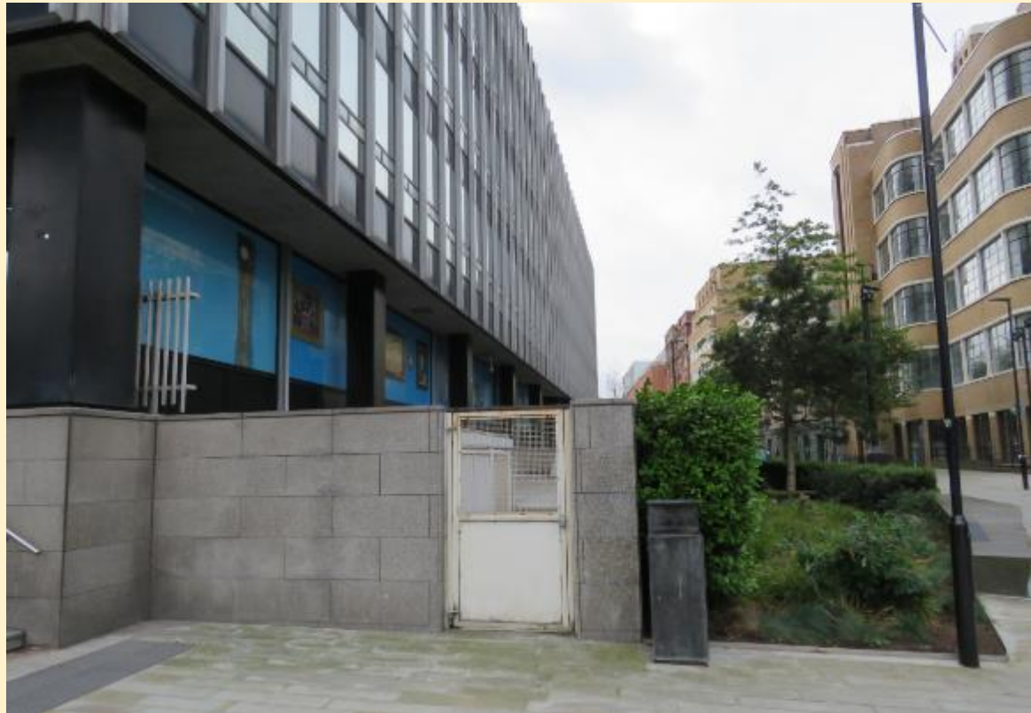
DS-09 Looking south along Dantzic Street toward the north-west fire escape
