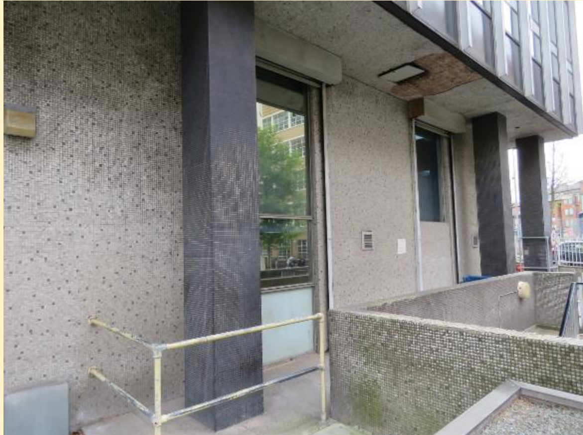
DS-05 Detail of the elevation and soffit materials, showing the south-west fire escape.
