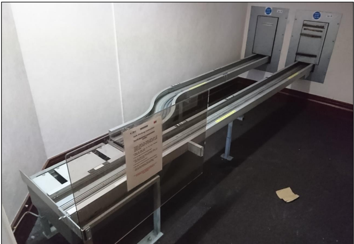
Figure 37. An example of the office-side dual track system on the 2 nd tower and podium floor, showing the entrance to the riser and vertical distribution.
