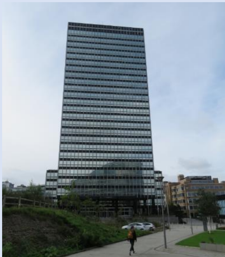
MS-02 View looking south-west showing the reflective result of the film applied to the glazing.
