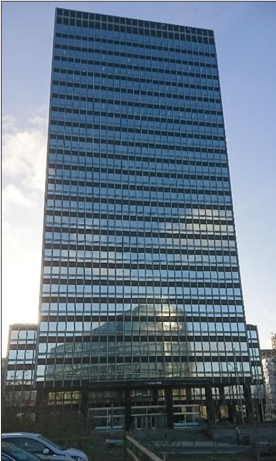
Figure 6. Miller Street elevation (Jan 2020), showing the result of the application of the reflective film on the glazing.
