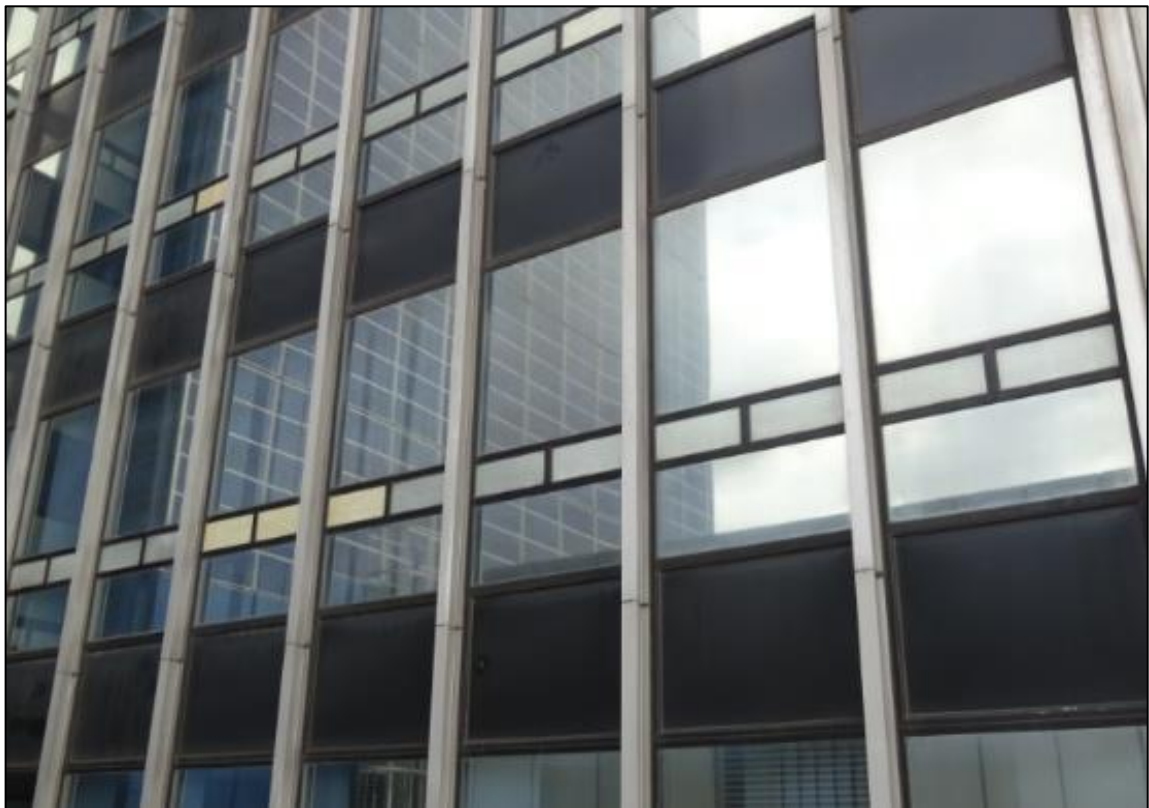
Figure 3. View of Miller Street frontage comprising black vitreous enamelled steel spandrel panels supported by the hiduminium mullions. The glazing panels are fitted internally and are supported by a mixture of timber and some replacement aluminium beads. The opaque horizontal glazing is formed of a encased asbestos/glass fibre sheet.
