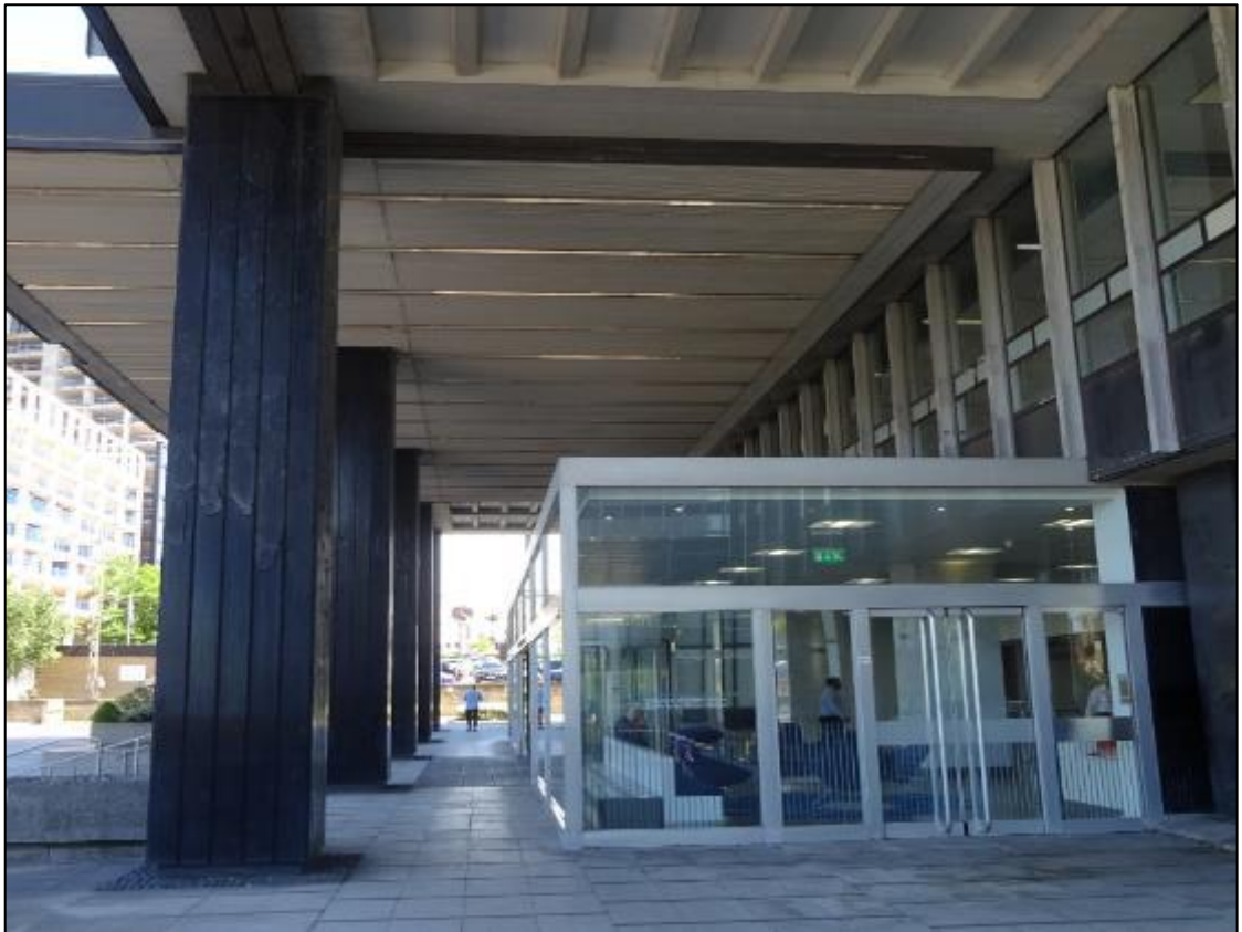
Figure 4. View of the main entrance onto Miller Street frontage (January 2020), showing the main soffit clad in metallic ceiling panels.
