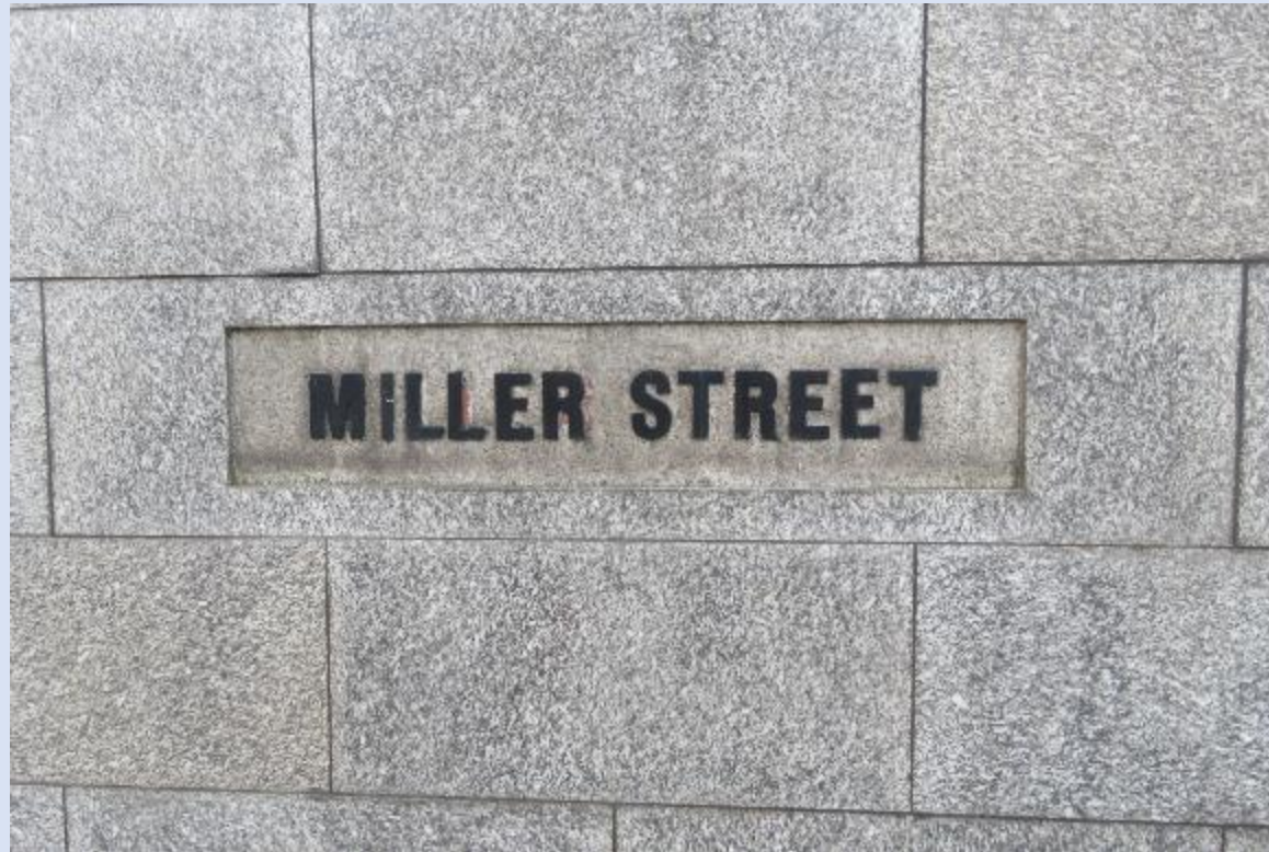
MS -09 Integral signage on retaining wall and planter.
