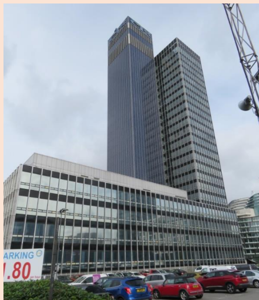
RS-02 Looking north-west from Hanover Street across the Riga Street car-park.
