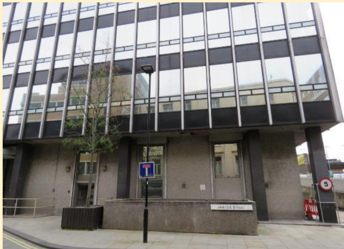
DS-04 Detail of the Dantzc Street elevation showing foreground south-west fire escape exit.
