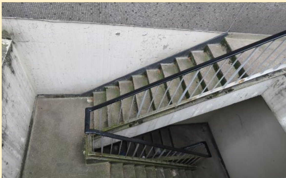
DS-06 View looking into the Dantzig Street south-west fire escape.
