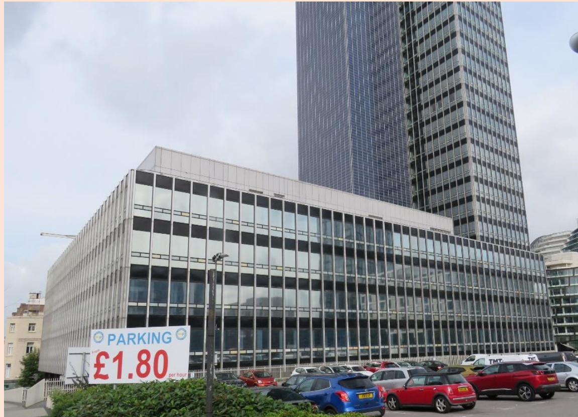
RS-09 Detail of the Riga Street podium elevation, looking north-west, showing the plant room and expressing the four main blocks to the building.
