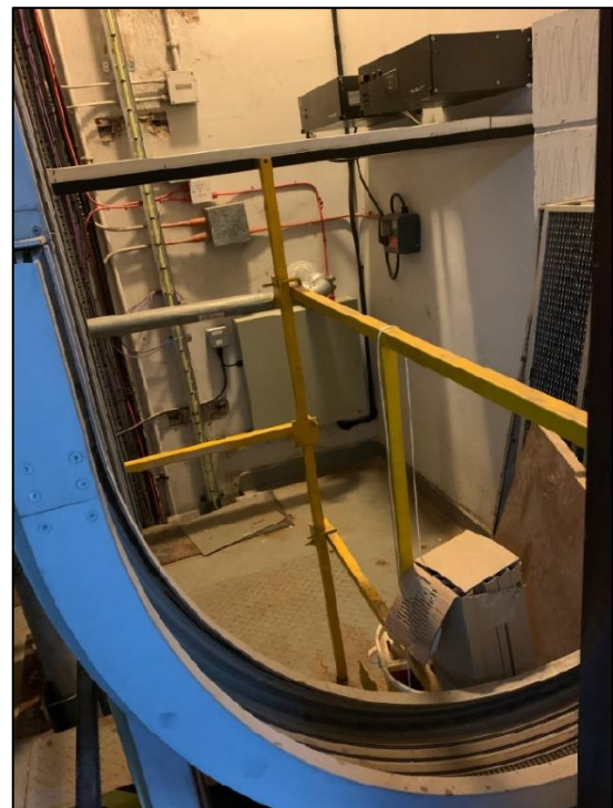
Figure 39. Views inside the vertical riser. Left-hand shows the track and door opening to the office and right-hand shows the curving track and the safety barriers.
