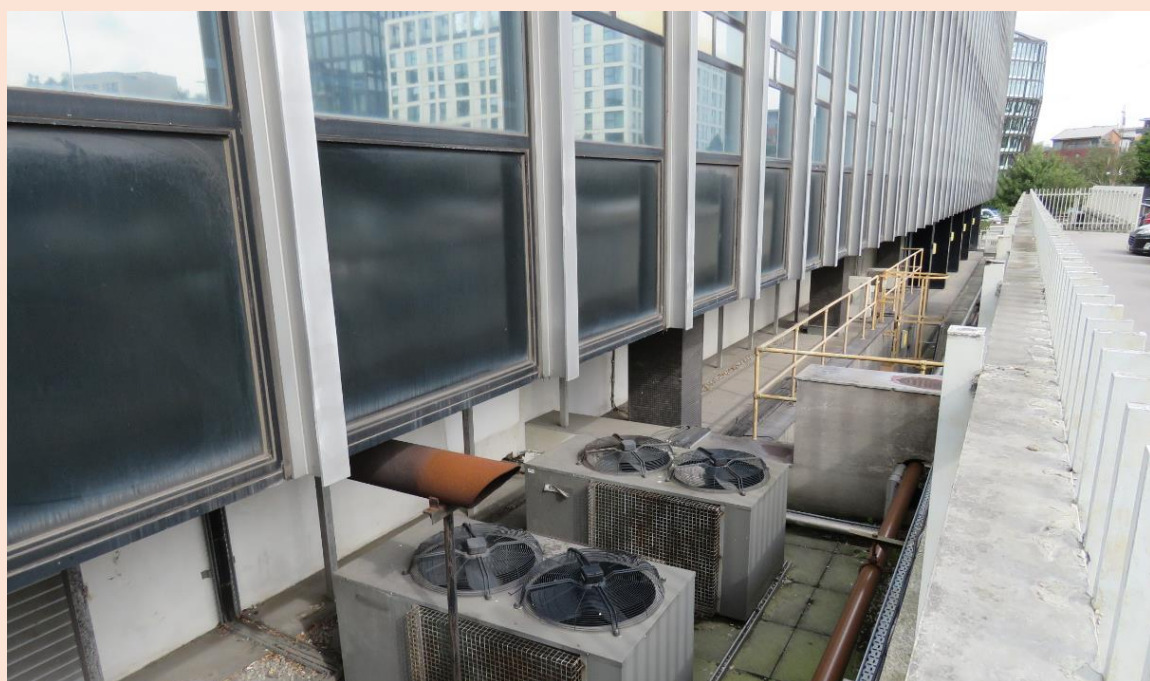
RS-06 Detail of the north end of the Riga Street plant basement abutting the carpark.
