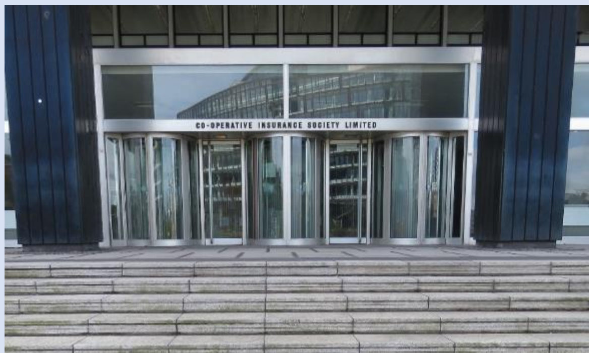
MS-04 Details of the concrete steps and non-original revolving doors and metal-sheet clad columns.
