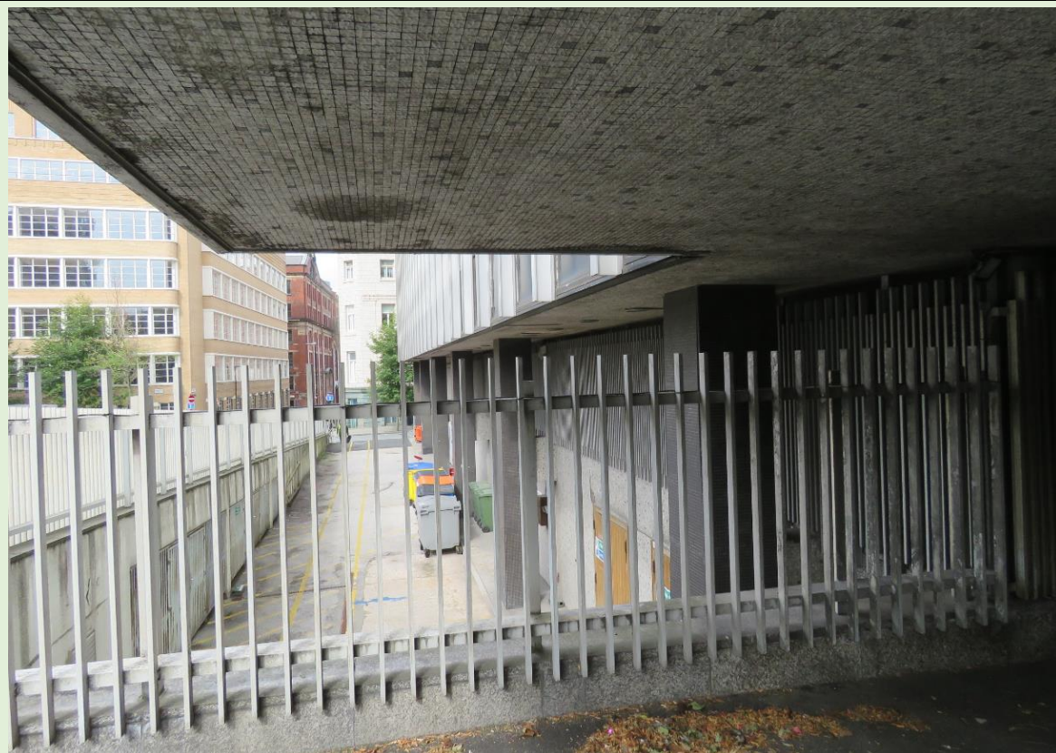
HS-06 Looking west from the car-park access bridge along the service yard, showing the tiled soffit of the canopy and detail of the square-section, grey painted railings.
