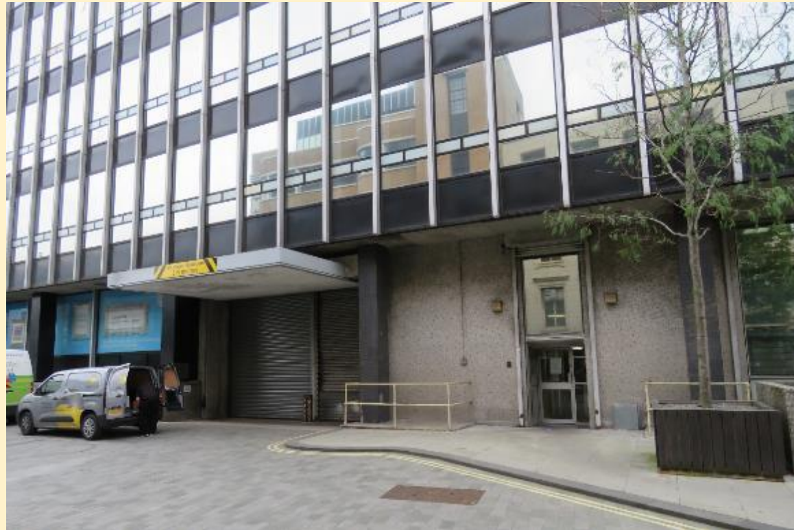
DS-03 Detail of the Dabtzc Street service entrances, showing the tiled elevations below the soffit and the reflective film to the glazing.
