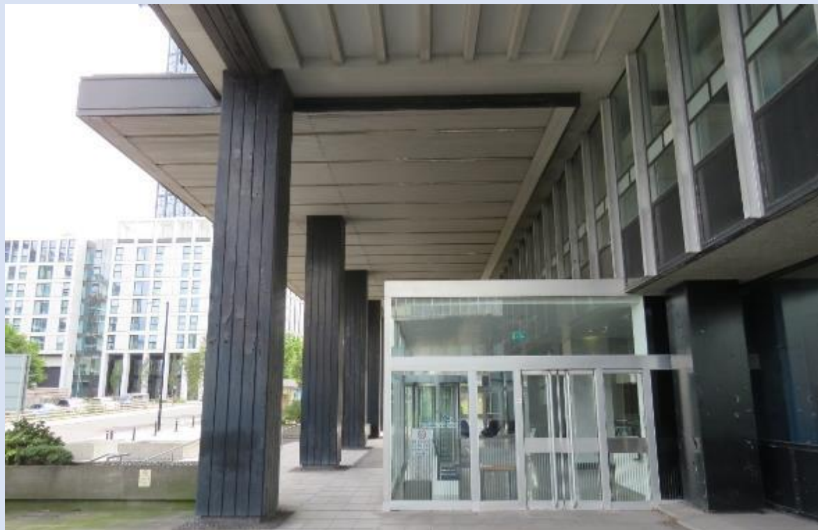
MS-06 View looking east into the entrance canopy and porch showing the concrete and metal panels and tiling to the main soffit of the porch.
