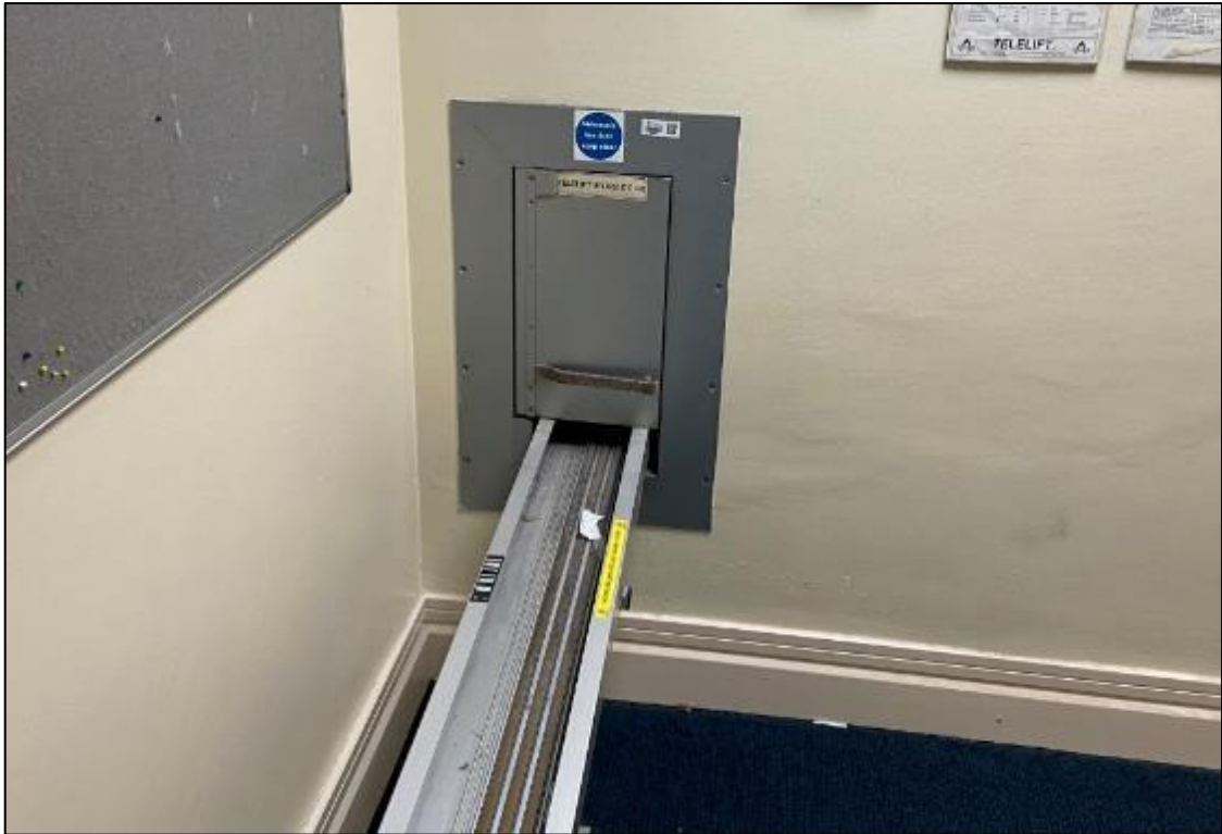
Figure 38. Example detail of the door to vertical riser and track bed.
