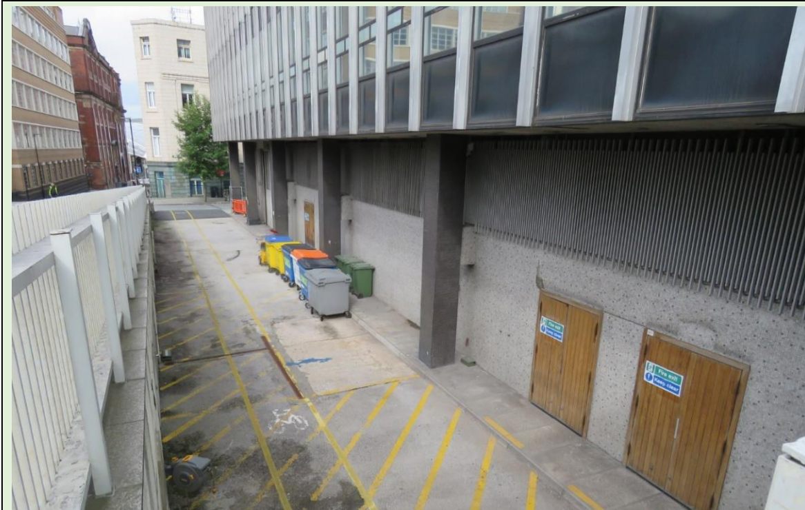
HS-07 Looking west along the Hanover Street service yard, showing the tile-clad elevations and columns.
