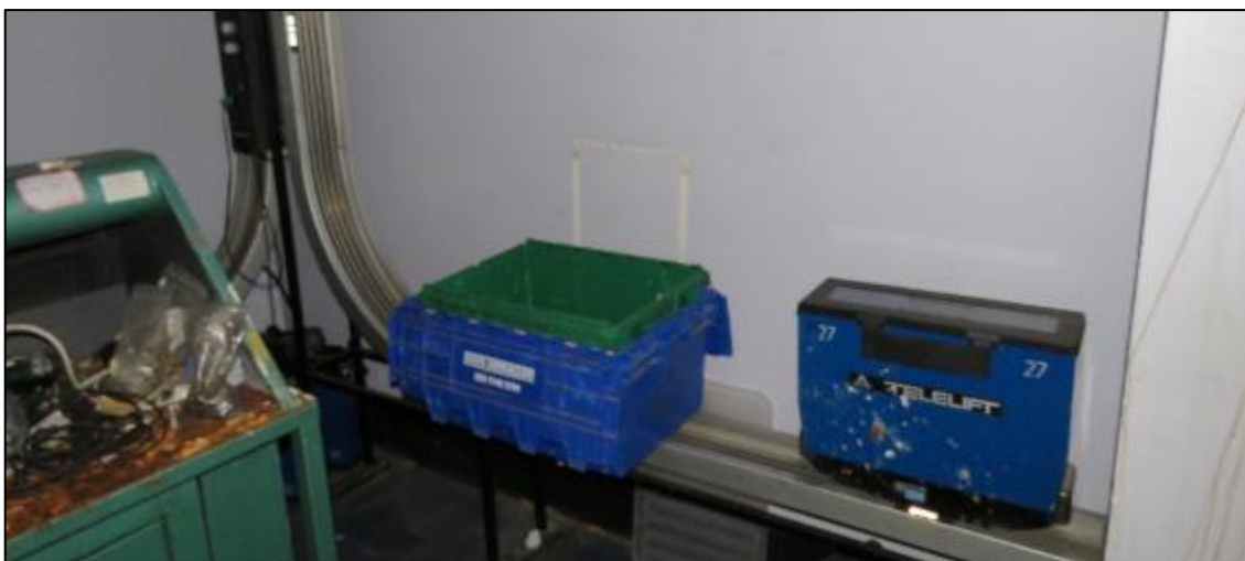
Figure 33. The end of the track and the document transportation units in the former postal services room (Level 00 – north-west).
