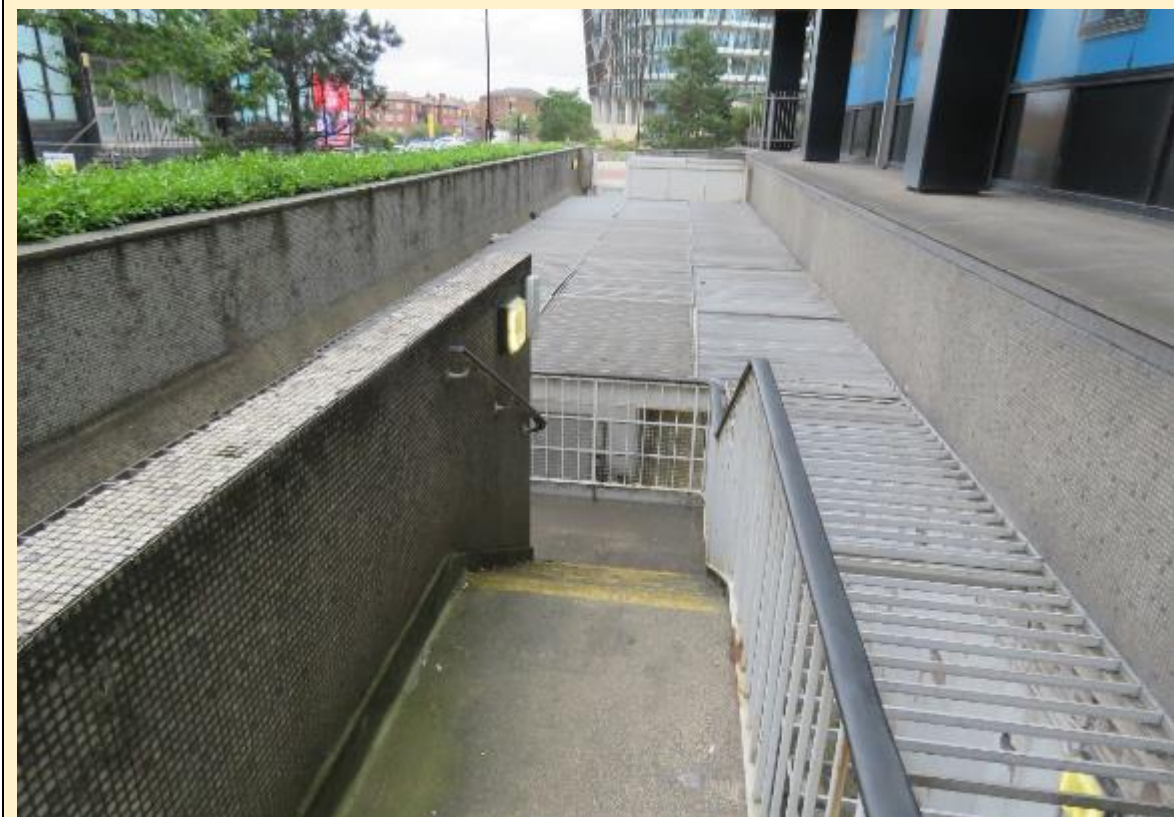
DS-08 Detail of the Dantzic Street north-west fire escape entrance and gas plant ventilation..
