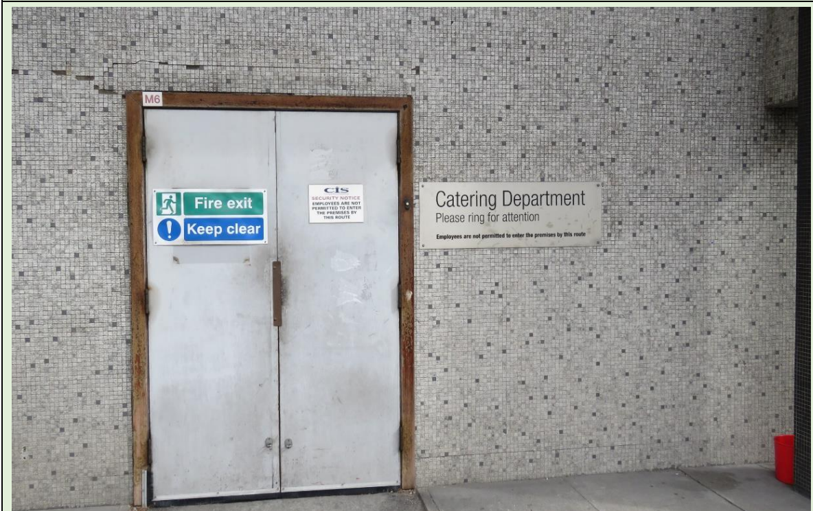
HS-10 Details of the tiling to the Hanover Street service yard and the kitchen delivery entrance.
