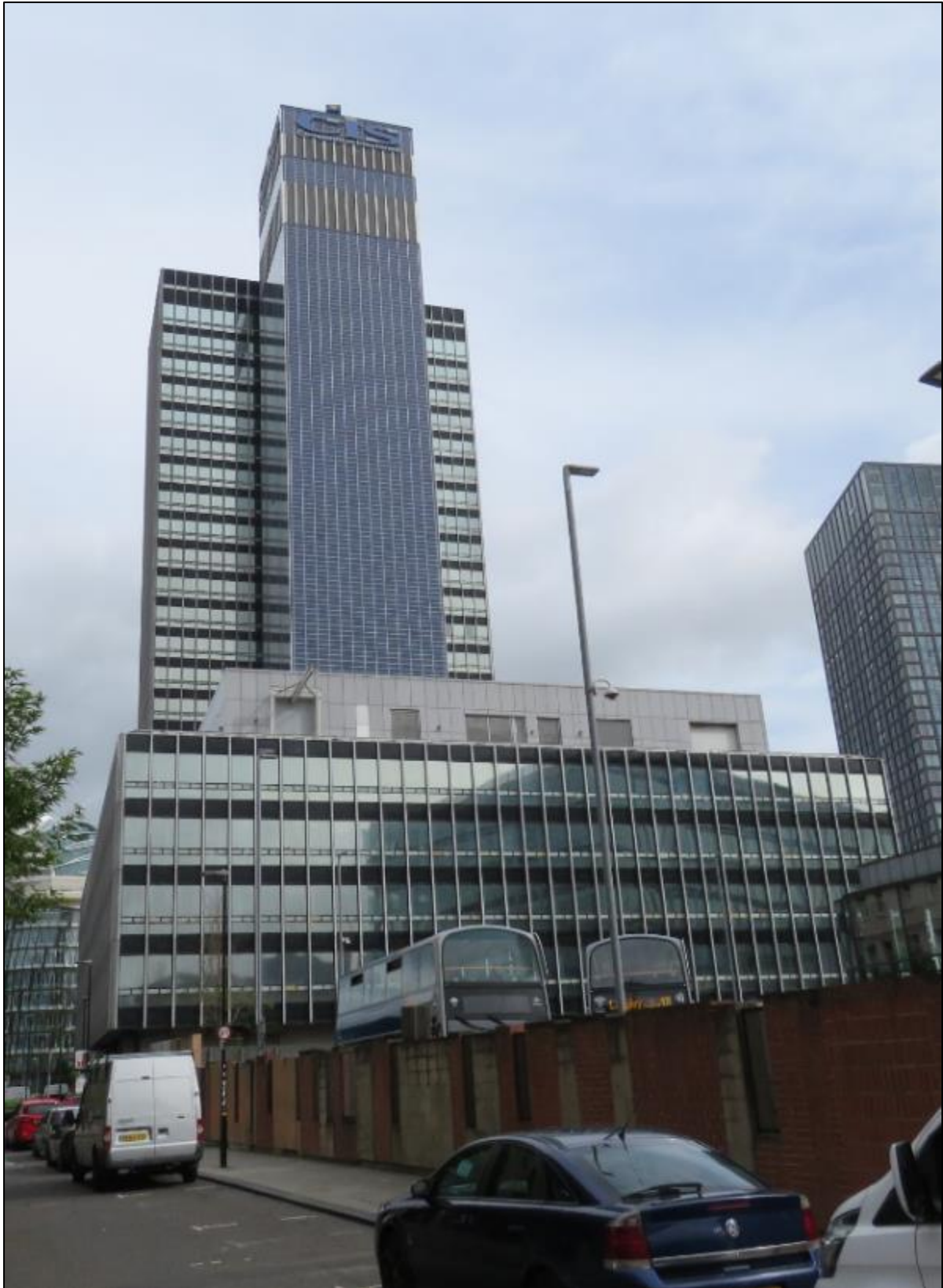
Figure 12. View of the Hanover Street frontage from the junction of Dantzic Street and Balloon Street, showing the exposed rear elevation of the podium following the redevelopment of the former warehouse to accommodate the bus station.
