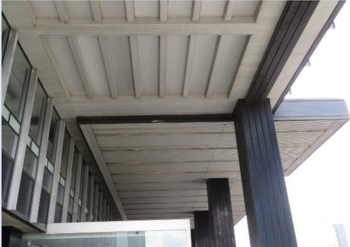
MS-07 Detail of the soffit to the entrance canopy showing the glazing to the mezzanine floor and columns.
