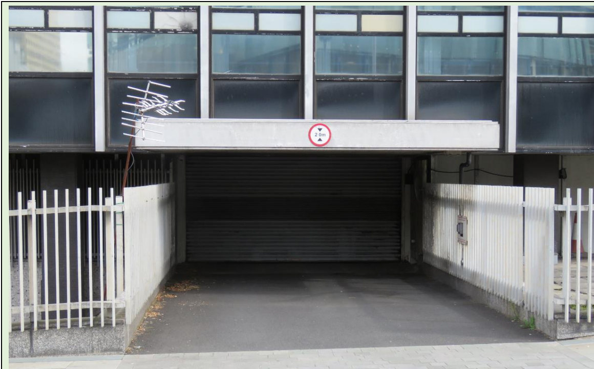
HS-05 Detail of the bridge and car-park entrance, showing the railings, canopy and roller-shutter door.
