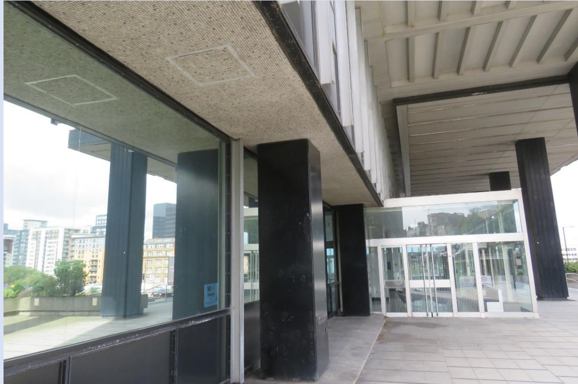
MS-05 View looking west into the entrance canopy and porch, showing the use of concrete, metal panels and tiling to the soffit.
