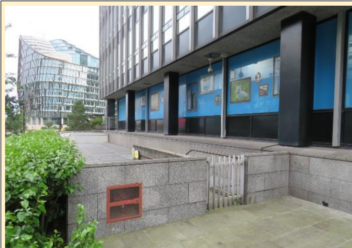
DS-07 Detail of the former Postal Dept elevation and north fire escape exit and plant room.
