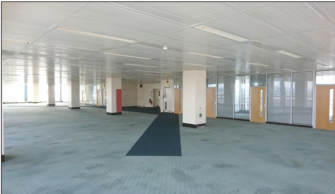
Figure 19. Typical office floor (August 2020), Level 16 (see Appendix 22 ). The partitioned offices are non-original, as is the floor covering, ceilings and decorative finish.
