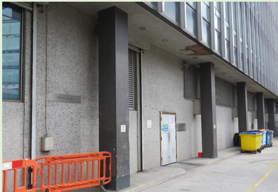
HS-08. Looking east along the Hanover Street service yard, showing the tile-clad soffit and access for kitchen deliveries and bin stores.
