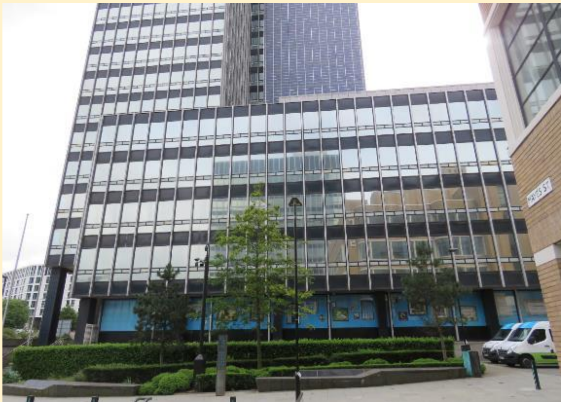
DS-02 Partial elevation from the steps to Sadlers Yard, showing the former ground-floor Postal Department rooms and the reflective nature of the applied glazing film. The hedge screens the north-west fire escape and gas-plant room.
