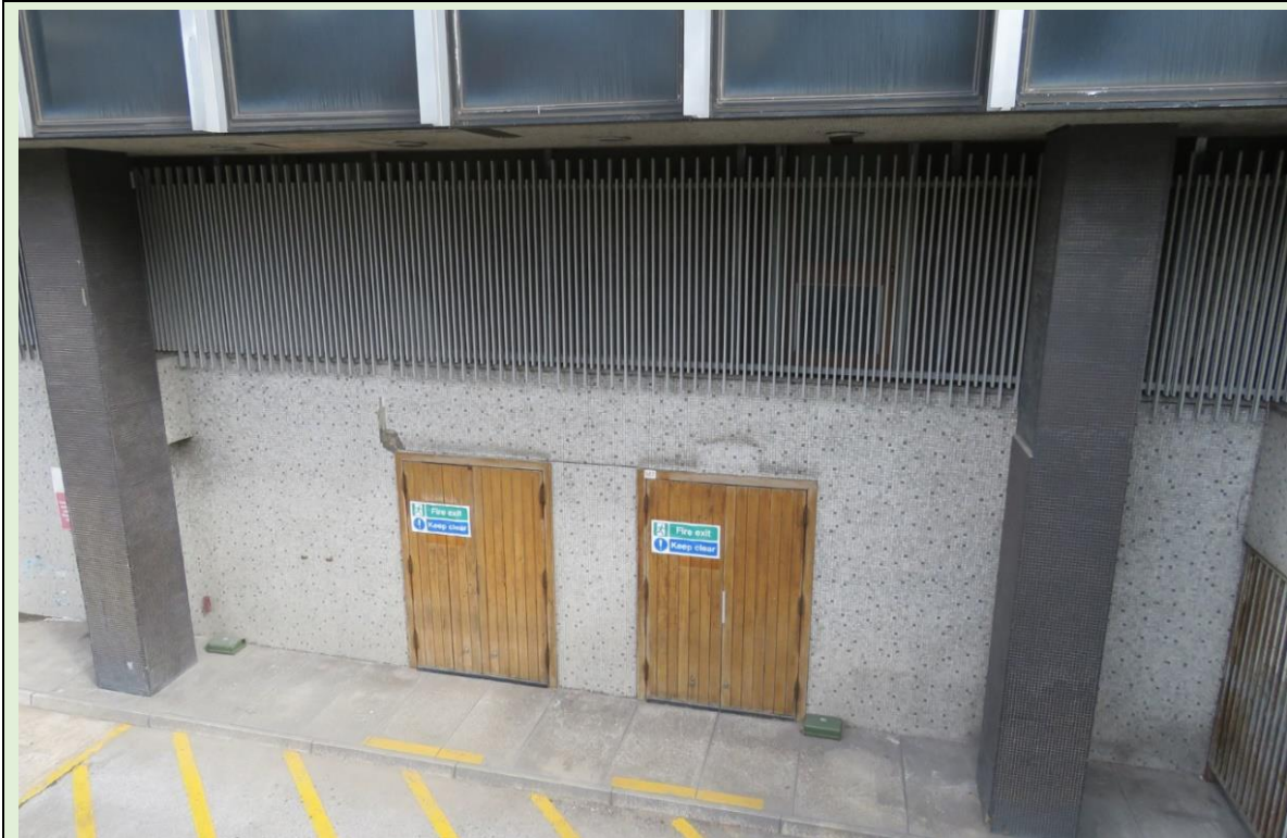
HS-09 Detail of the Hanover Street service yard elevation and fire-escape doors. The railings to the elevation screen the executive garage. Showing the tile-clad elevations, soffit and columns.
