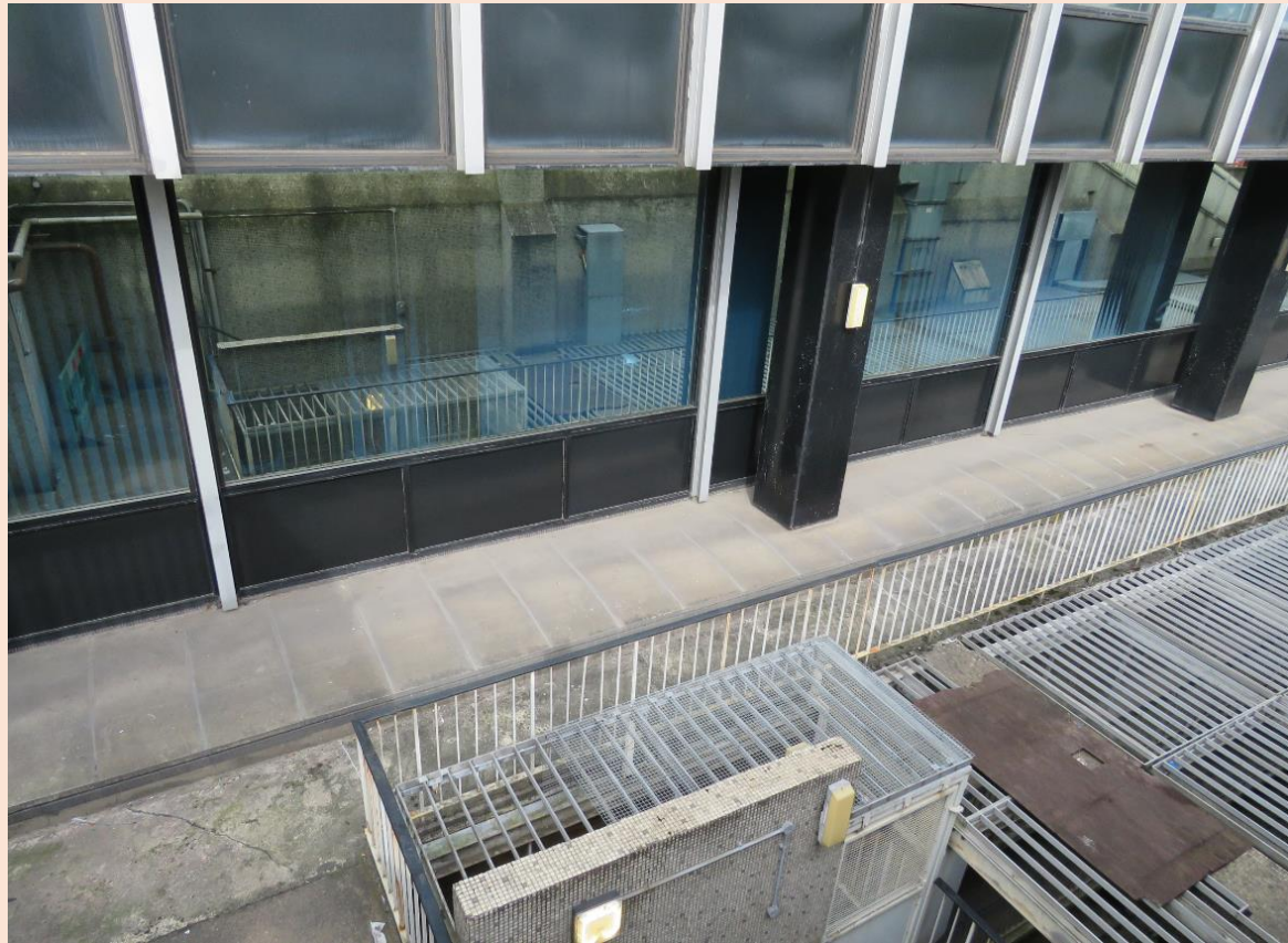
RS-05 Detail of the central section of the Riga Street ground floor elevation and plant basement, showing the reflective nature of the film applied to the glazing.
