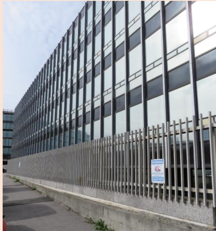
RS-07 Looking south showing detail of the Riga Street podium elevation and railings.
