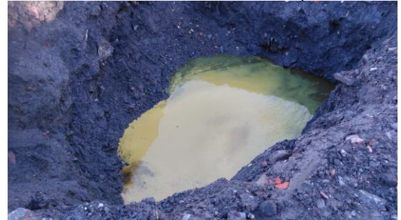
View of the oil contaminated excavation
