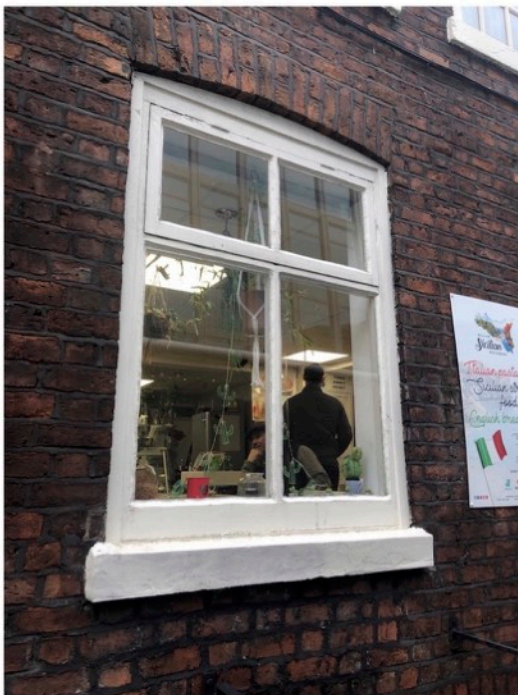
WINDOW W.02 REPLACEMENT TOP HUNG OPENING LIGHT AND FIXED WINDOW NOT ORIGINAL
