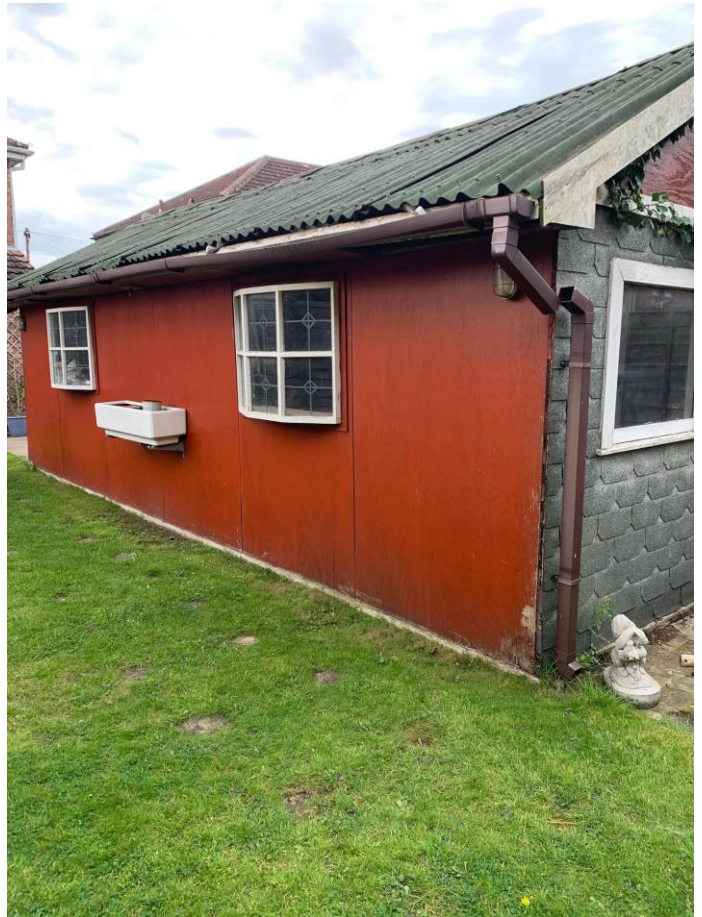
Timber garage / workshop in the garden which is in a poor state of repair and to be demolished. Photo taken 23.09.2020
