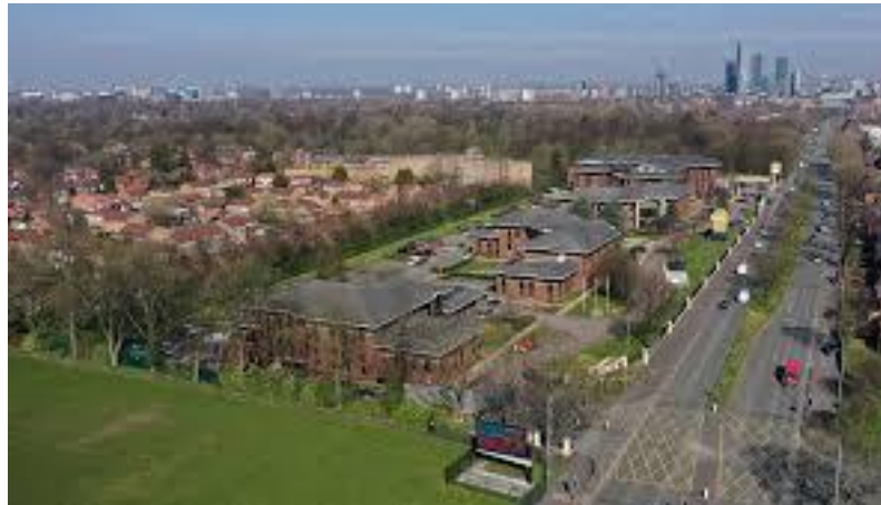
Parkway Business Park: Not fully let since construction
