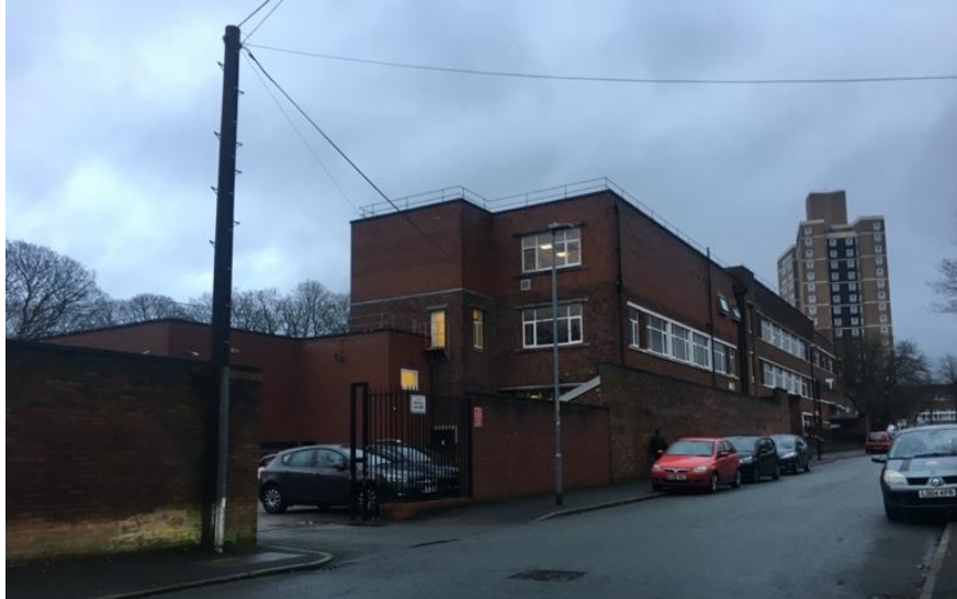
View of 1980's extension from Langley Rd.
