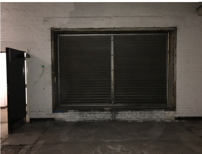
Current condition of back of louvre area
