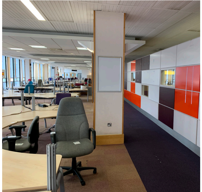
Level 3 (highlighting metal wall panelling and column trims)
