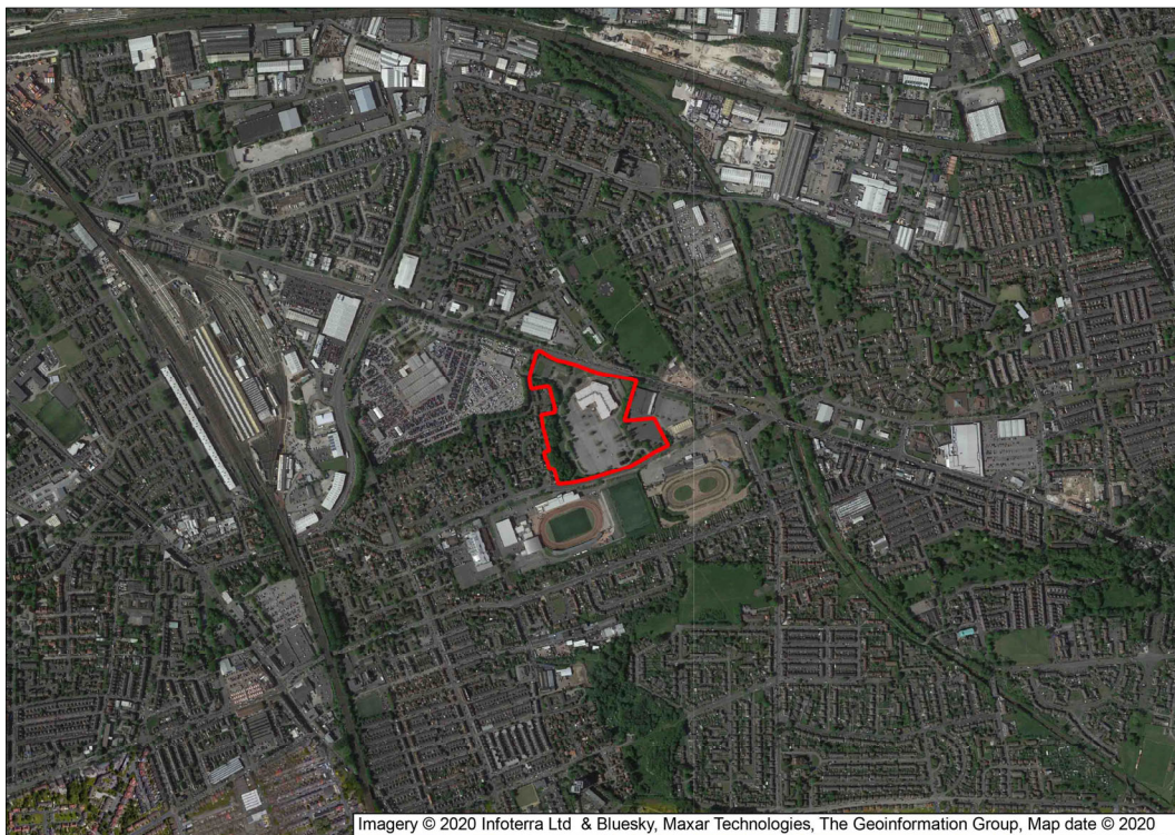
Figure 1. The Hyde Road School site
