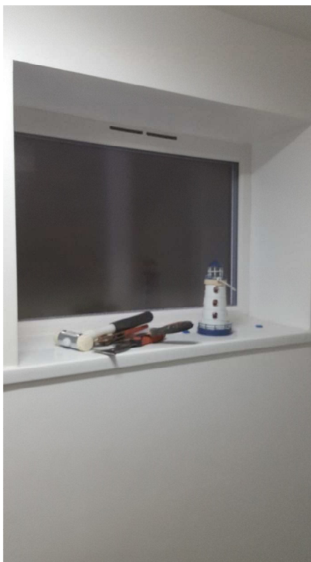
Basement communal hall
