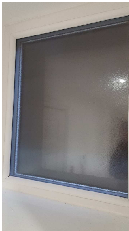
Basement rear flat hall
