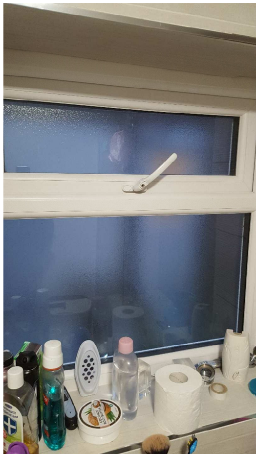
First floor flat bathroom
