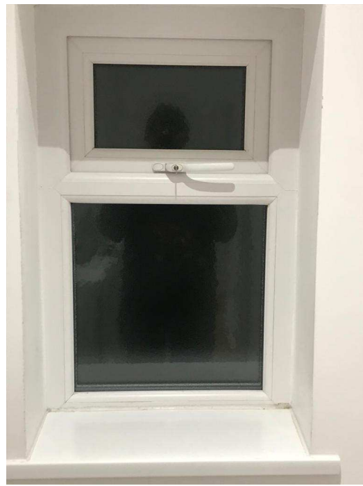
First floor flat hall
