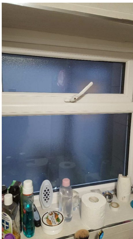
Ground floor flat bathroom
