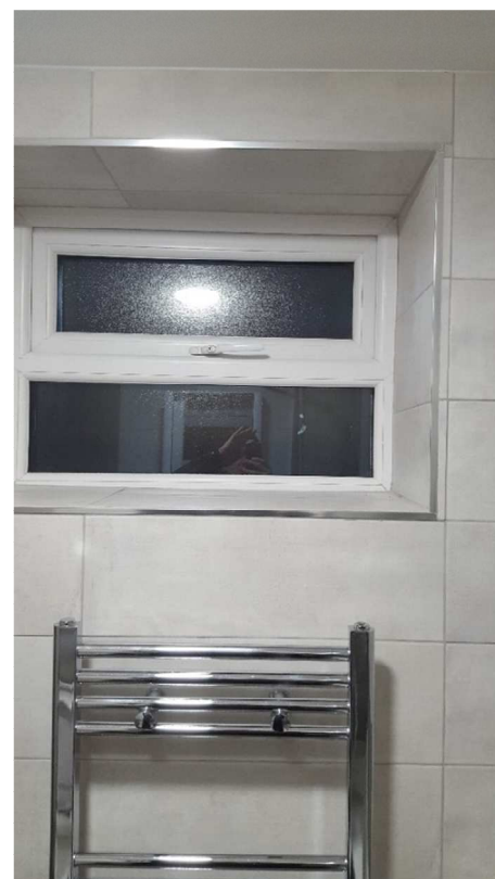
Basement rear flat bathroom
