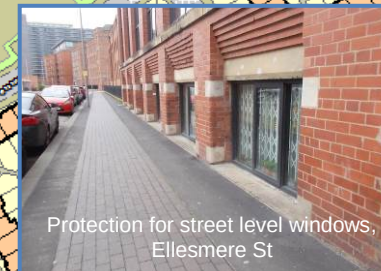
Ellesmere St looking northeast towards Phoenix House
