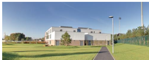
Existing school building viewed from the East boundary
