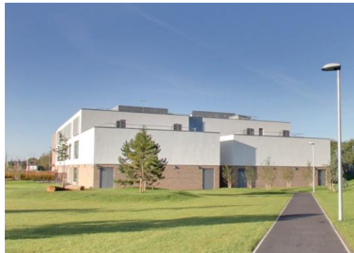
Existing Rear Elevation – The existing building is a mix of brick and render. This has been incorporated in the designs of the new building
