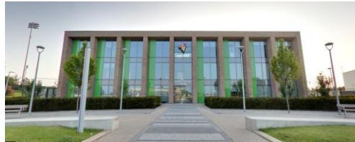
Existing college main entrance
