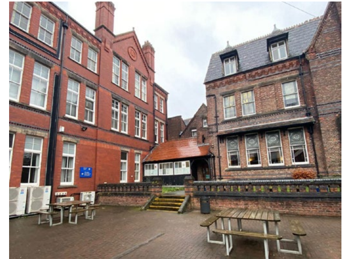
3 - retaining wall in courtyard corner
