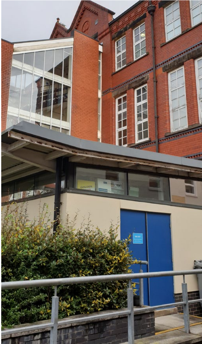
1 - existing single storey element with fire escape stair above
