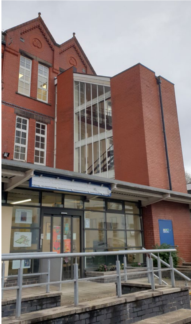
1 - fire escape stair
