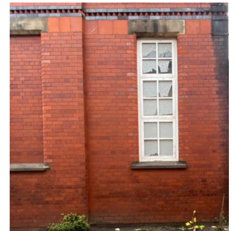
Timber window, multi-paned glass (made opaque through dilapidated vinyl) - location of new fire escape stair door.
