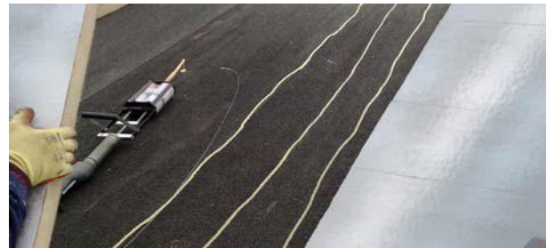
New insulation provided. Adhesive or mechanical fix.
