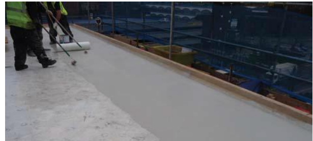
Application of waterproofing direct to primed insulation.
