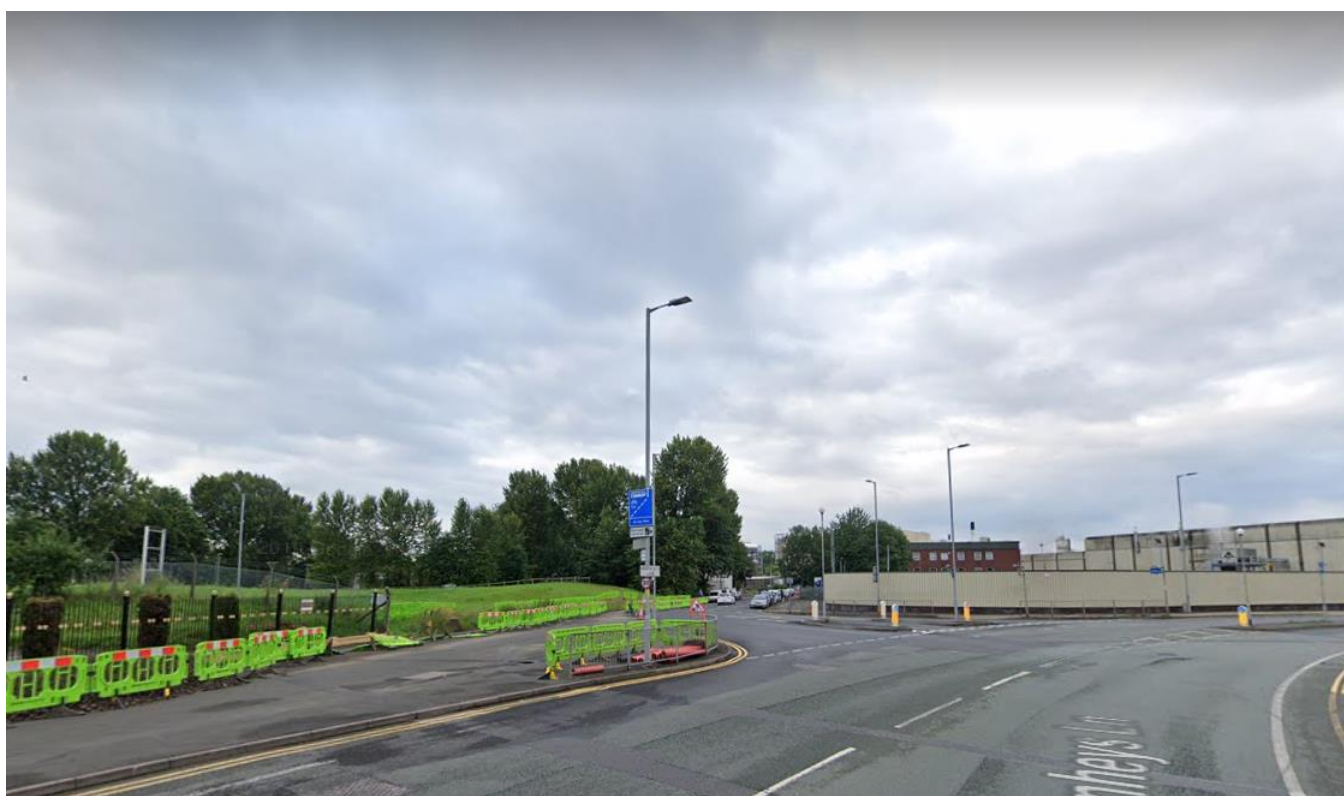
View south west towards site from Greenheys Lane/Charles Halle Road
