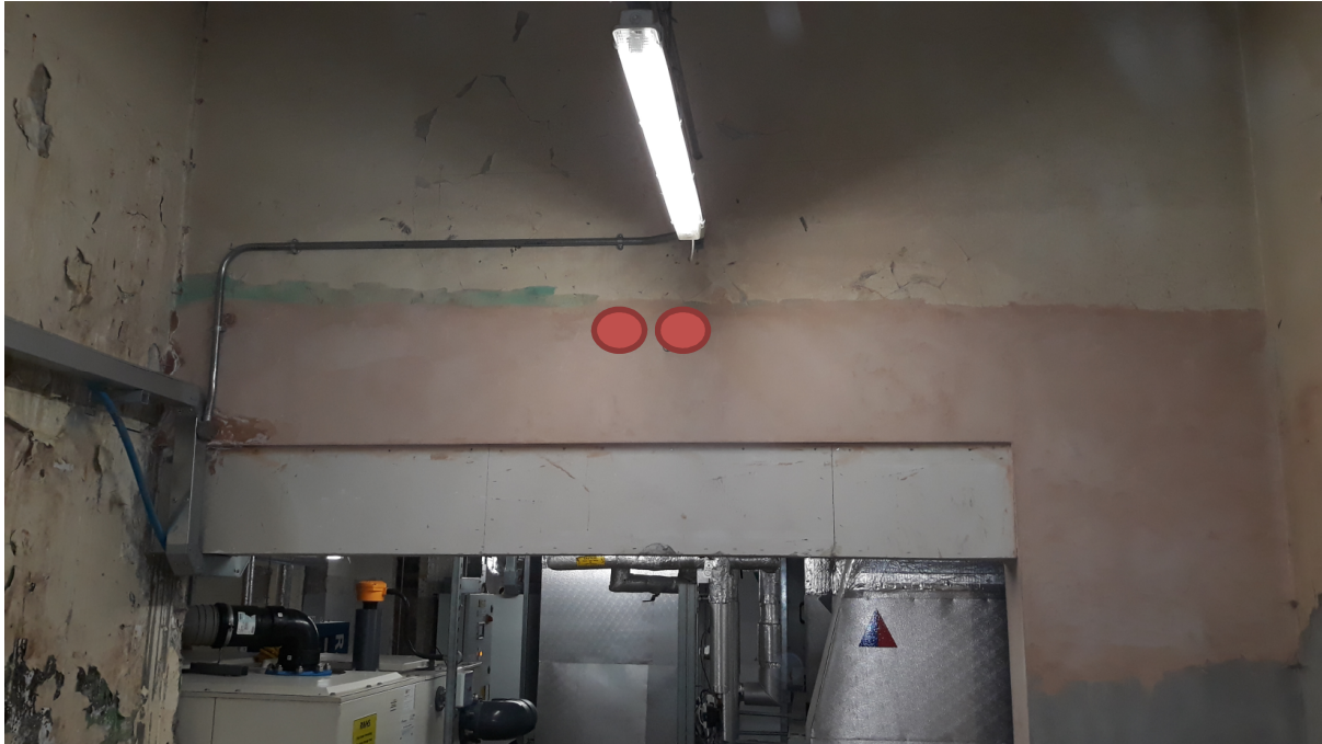
Basement plantroom HV cable ladder route through existing blockwork wall
