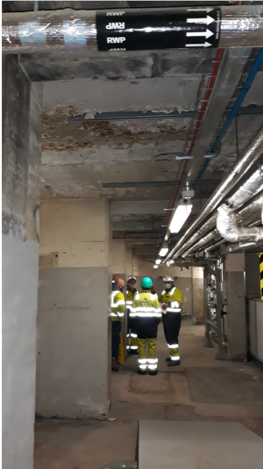
Basement plantroom HV cable ladder route adjacent existing services
