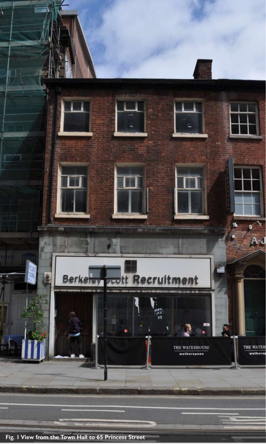
Fig. 1 View from the Town Hall to 65 Princess Street
