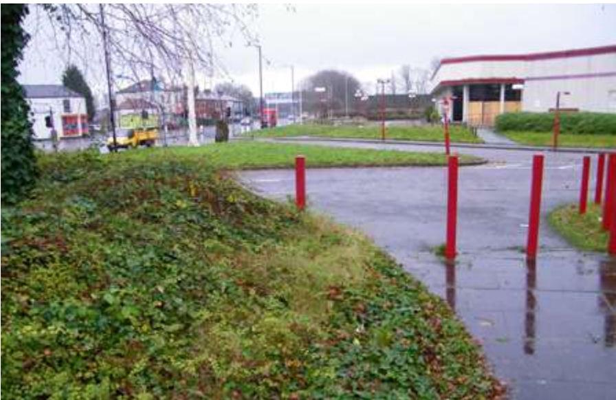
View of existing site entrance
