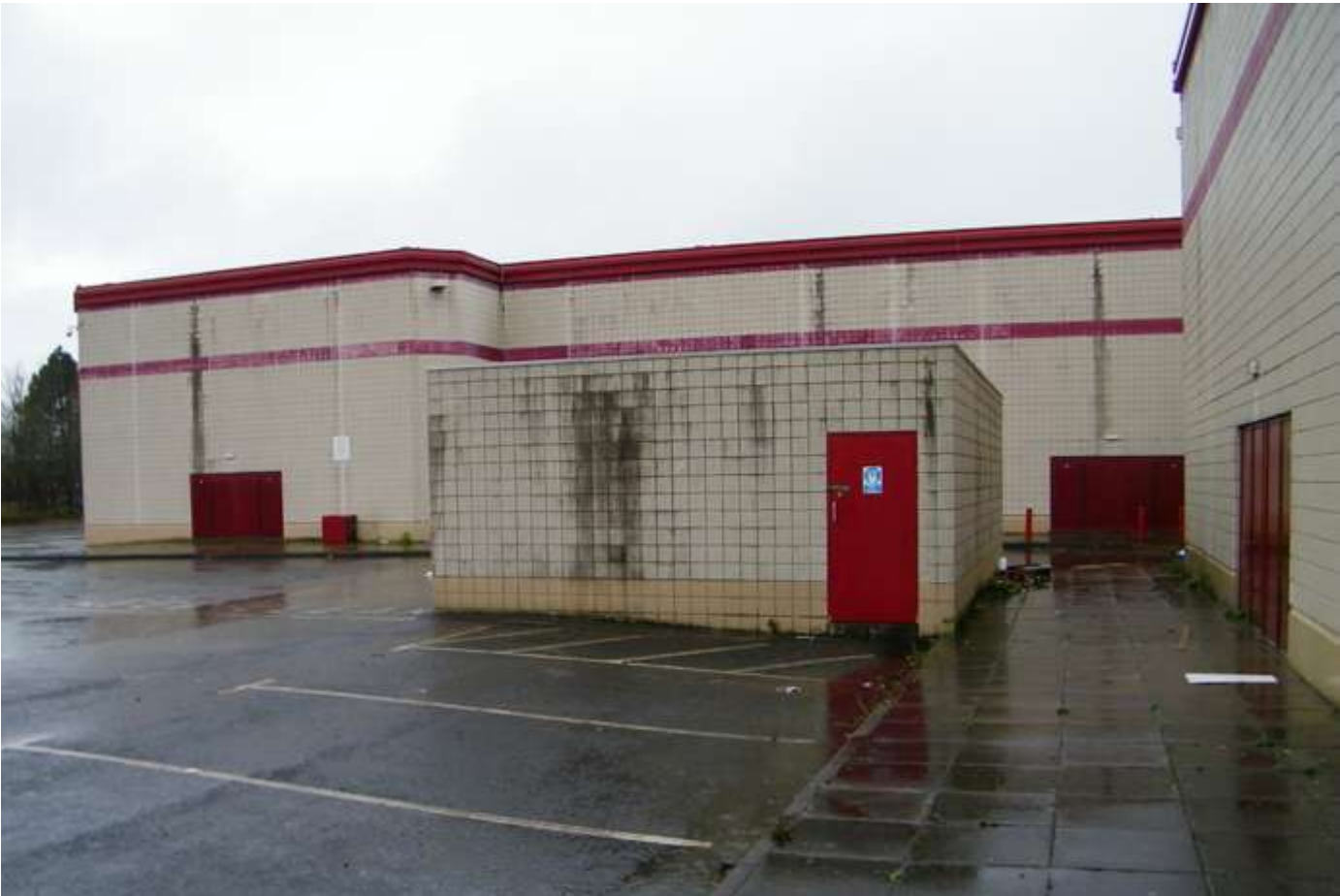
View of existing building from Rear
