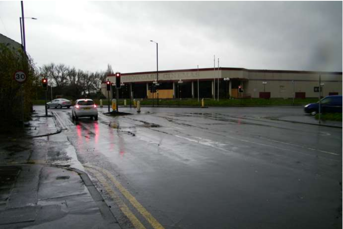
View of existing building from Hyde Road
