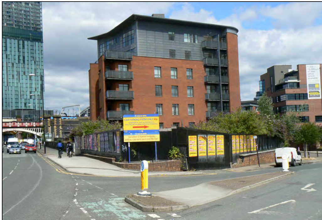
Plate 9: View of the Site Area from the west, showing the Bridgewater Viaduct to the right
