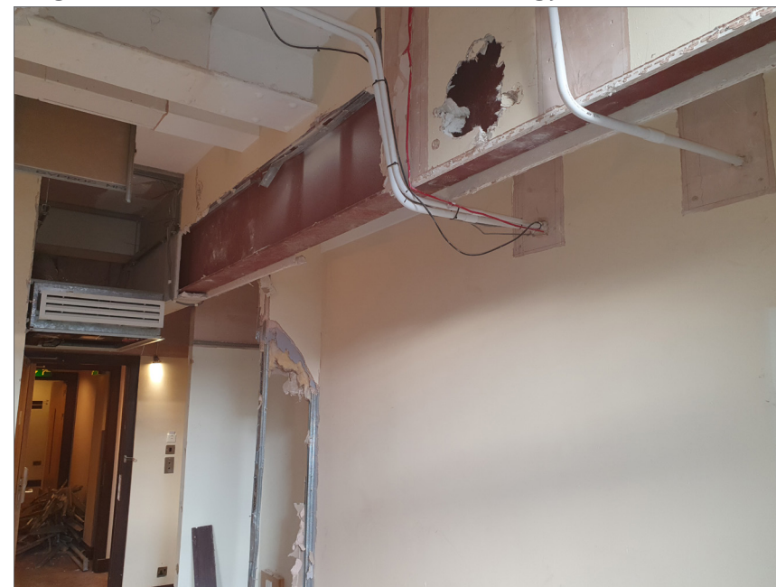
Guestroom beam lining removed to expose modern steel beam.
