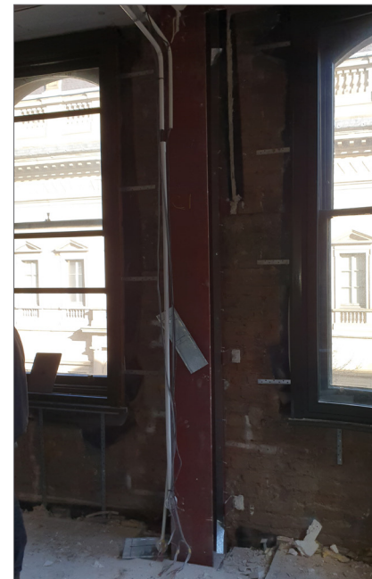
Guestroom Wall with liner wall & column lining removed
