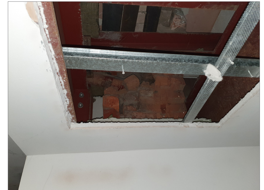
Opening through fire boarded bulkhead to reveal modern steelwork forming opening through original masonry wall in basement.
