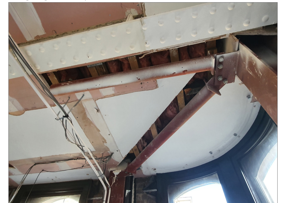
Existing fire boarding to beams removed to reveal modern beams.
