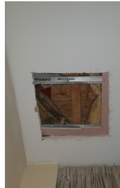
Opening through fire boarded soffit to reveal existing joisted floor & floor boards
