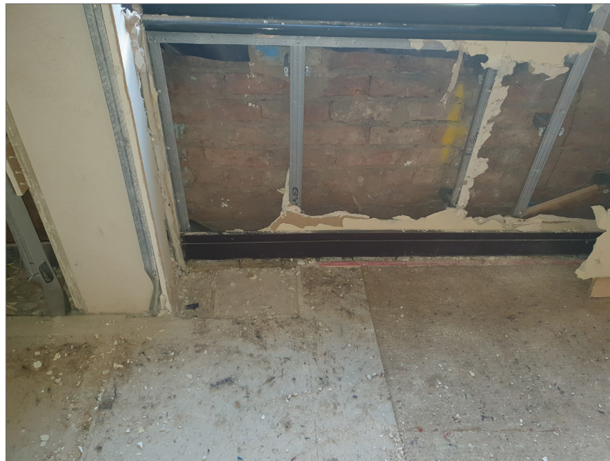
Guestroom Wall with liner wall removed
