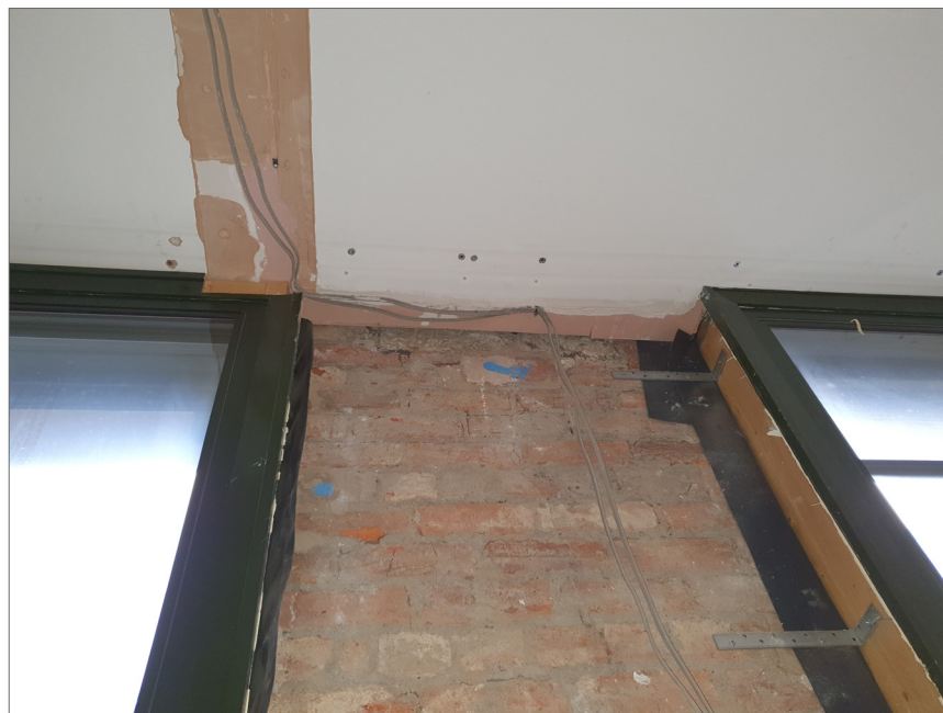
Guestroom soffit with liner wall removed
