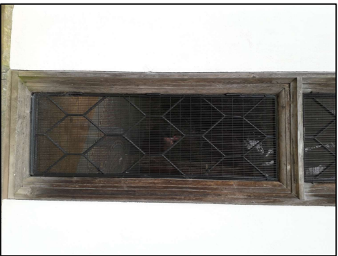
P84 - View of adjacent window fitted with mesh protective grille to external face.
