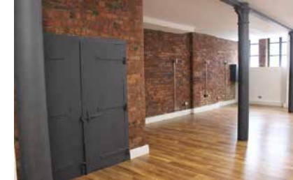
Existing painted iron columns and 1hr plasterboard ceiling works done under previously approved application 101365/LO/2013/C2 to be retained as part of proposed works [Photo taken 02.02.20]
