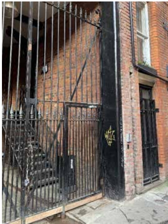
Existing loading bay gates with access control under previously approved application 101365/LO/2013/C2. [Photo taken 15.11.19]
