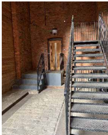
Existing loading bay works under previously approved application 101365/LO/2013/C2. Non-original steel staircase to be removed to accommodate DDA loading bay lift [Photo taken 15.11.19]
