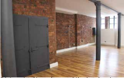
Existing painted iron columns and 1hr plasterboard ceiling works done under previously approved application 101365/LO/2013/C2 to be retained as part of proposed works [Photo taken 02.02.20]
