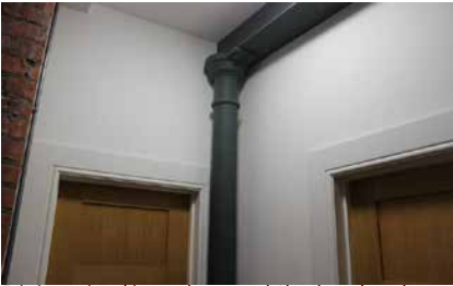
Existing painted iron columns and 1hr plasterboard ceiling works done under previously approved application 101365/LO/2013/C2 to be retained as part of proposed. Previous non-original partition works to be amended to suit proposed layout [Photo taken 02.02.20]
