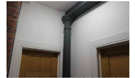
Existing painted iron columns and 1hr plasterboard ceiling works done under previously approved application 101365/LO/2013/C2 to be retained as part of proposed. Previous non-original partition works to be amended to suit proposed layout [Photo taken 02.02.20]
