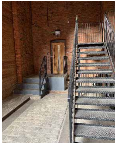
Existing loading bay works under previously approved application 101365/LO/2013/C2. Non-original steel staircase to be removed to accommodate DDA loading bay lift [Photo taken 15.11.19]
