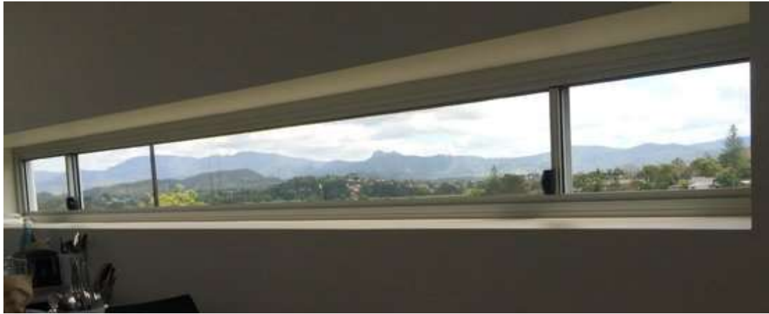
Slot window will allow light but offer 2 way privacy.
