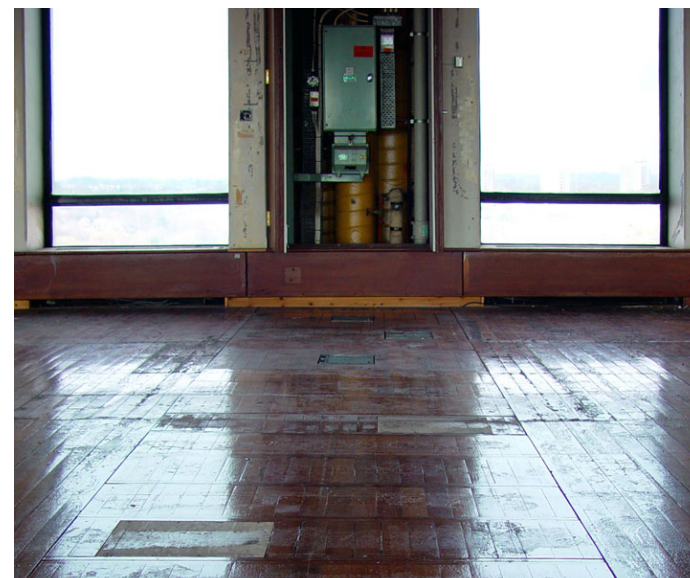
Historic Photograph: Original floor fucts and services located within facade voids
