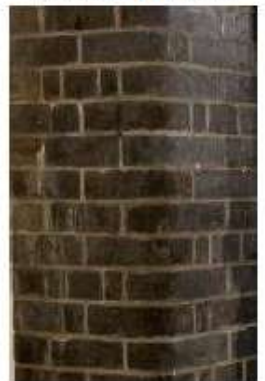
EXISTING BRICK EXPOSED IN PARTS
