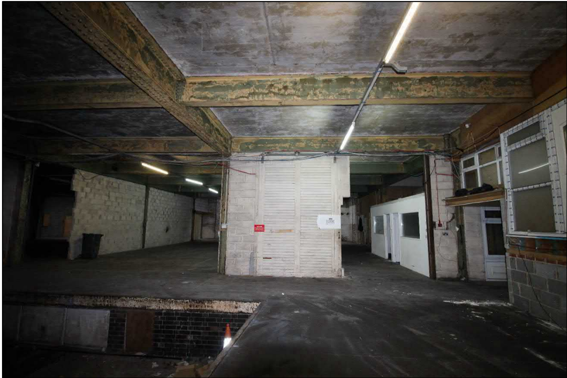
Plate 33: The partition wall between the loading-bay and the storage area to the south-west
