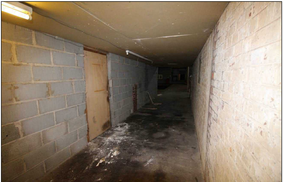
Plate 29: The narrow corridor giving internal access between the later office block and the earlier warehouse
