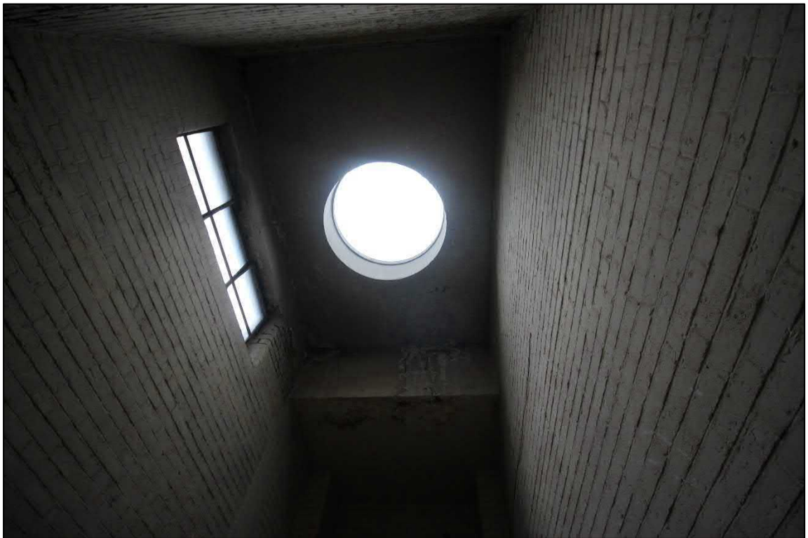
Plate 40: Detail of the round skylight and the single window within the southern stairwell
