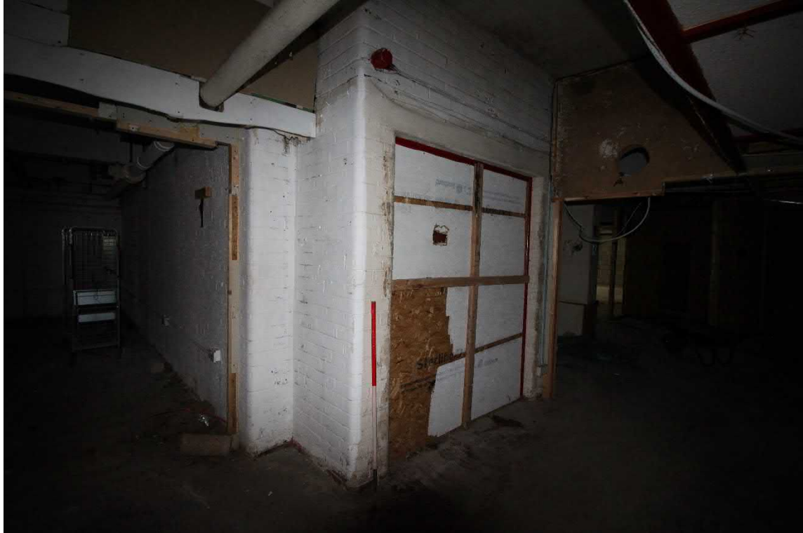
Plate 76: The blocked entrance into the north-eastern staircase
