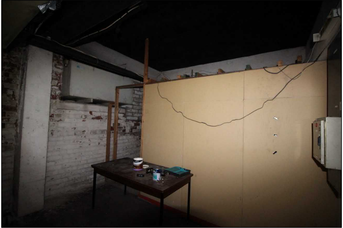
Plate 81: The toilet at the northern end of the basement
