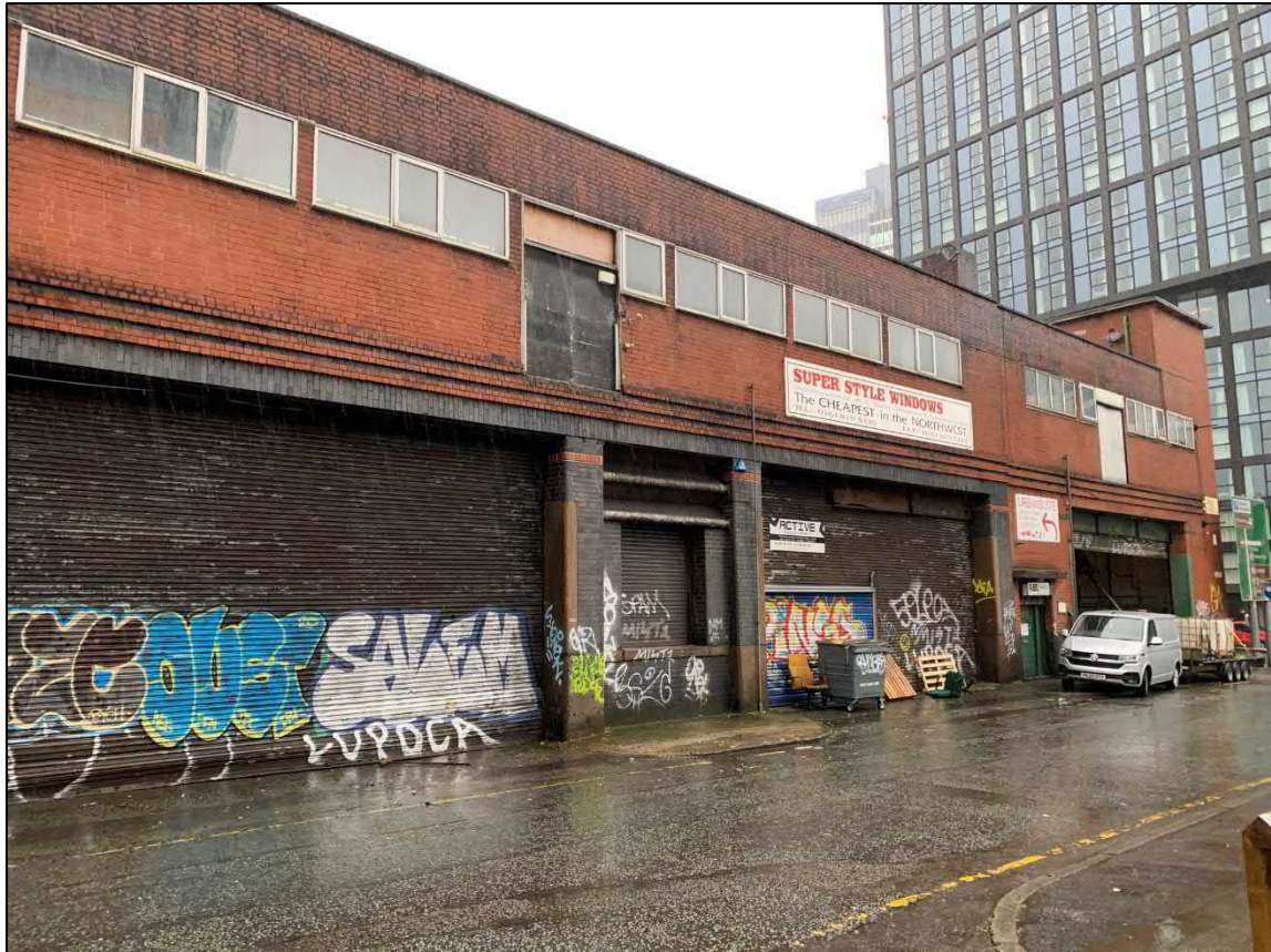
Plate 14: The north-western end of the north-eastern elevation
