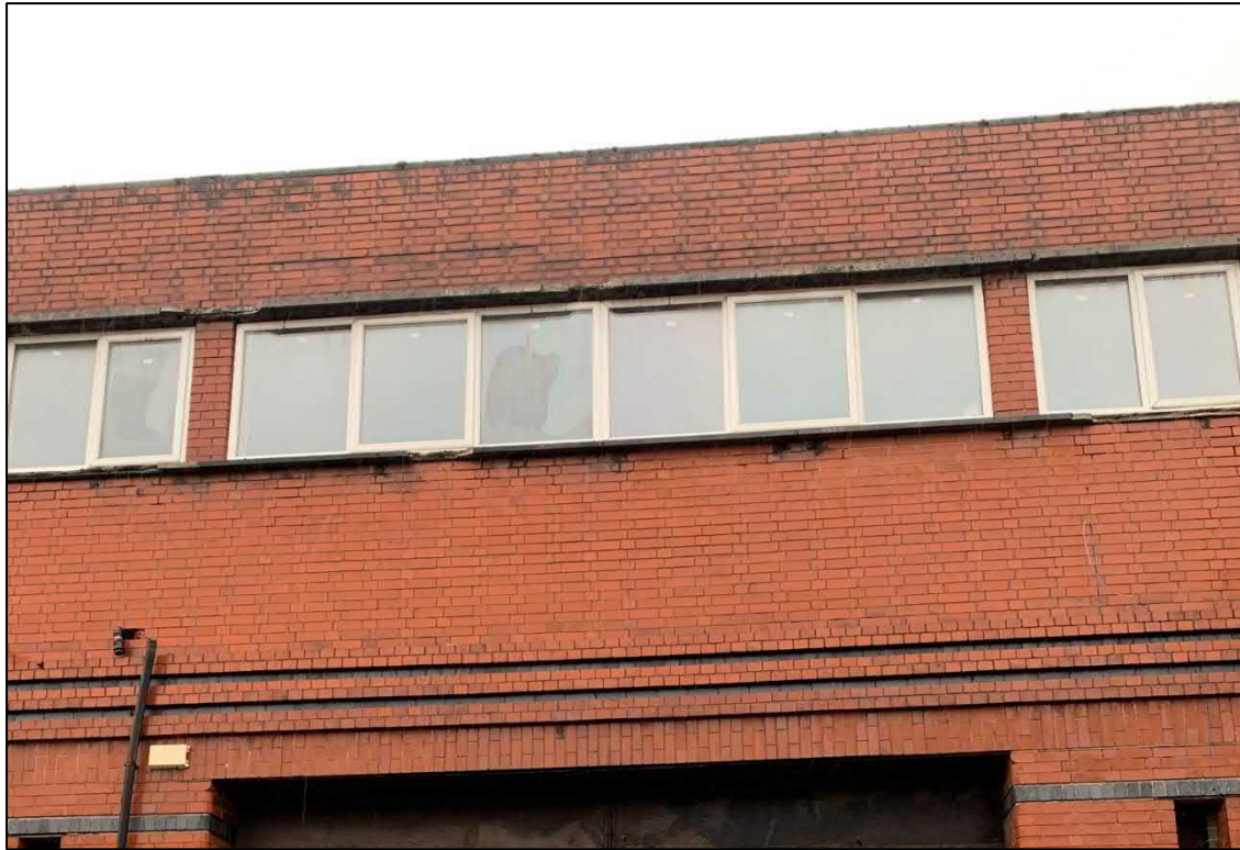
Plate 19: Detail of the first-floor windows on the south-eastern elevation
