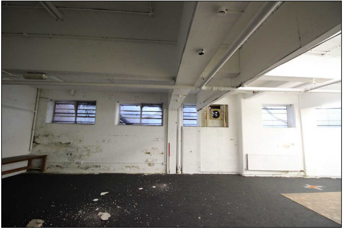
Plate 79: The windows within the south-west wall
