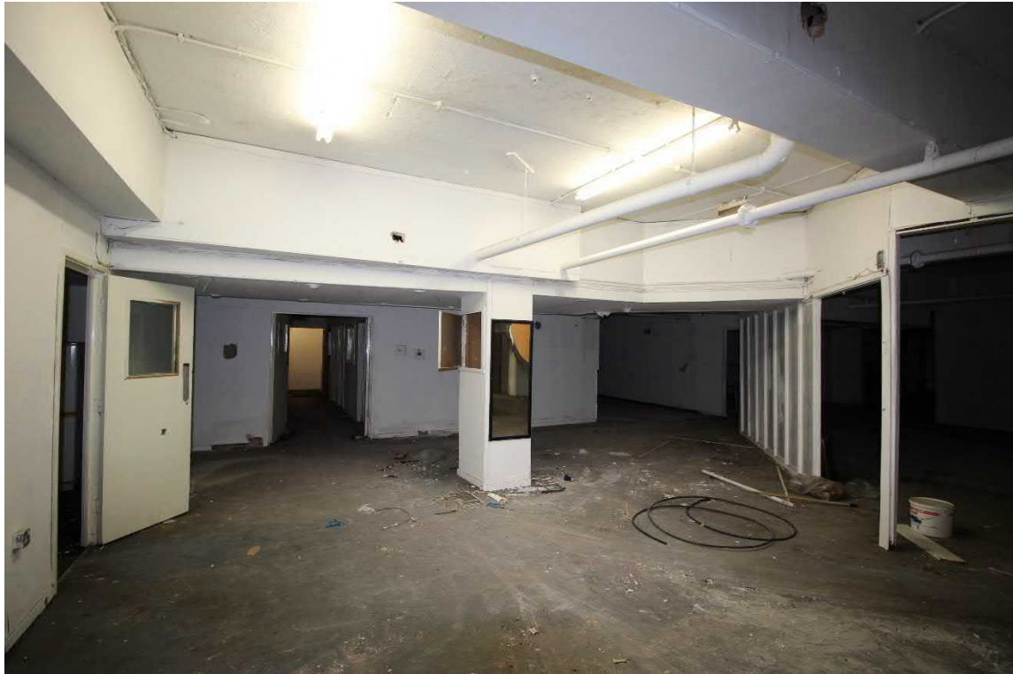
Plate 77: General view of the central room of the office block basement
