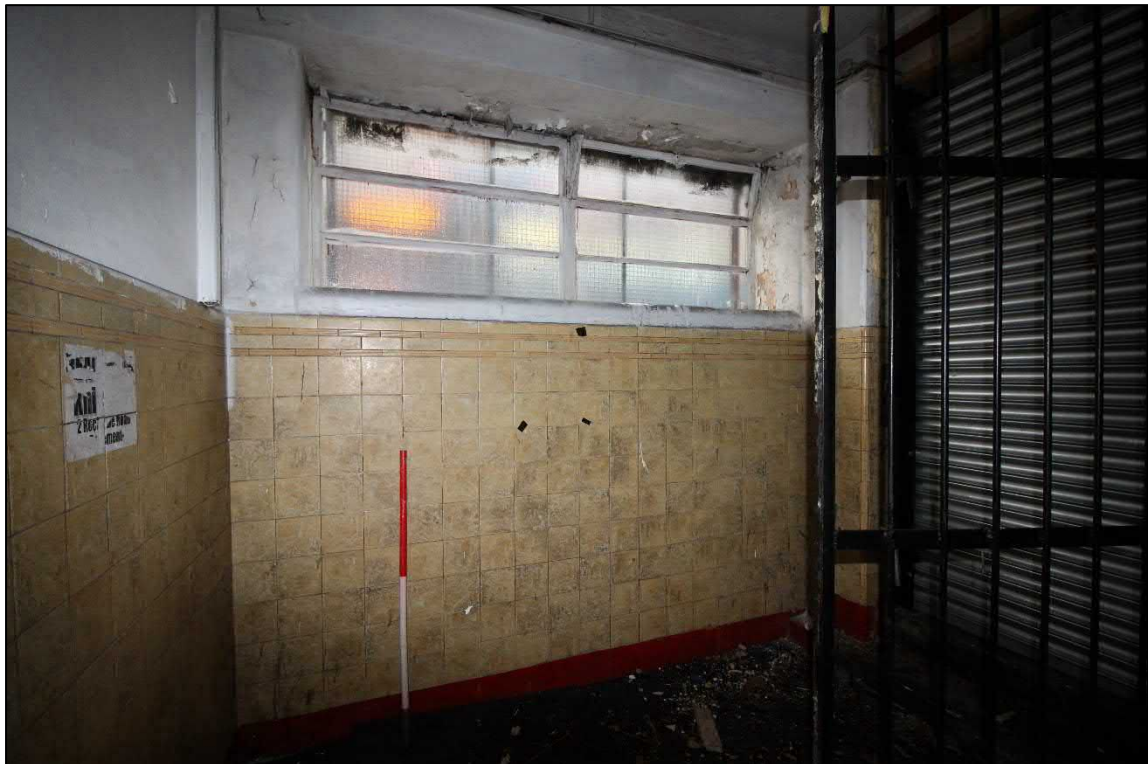
Plate 84: The basement landing of the northern stairwell
