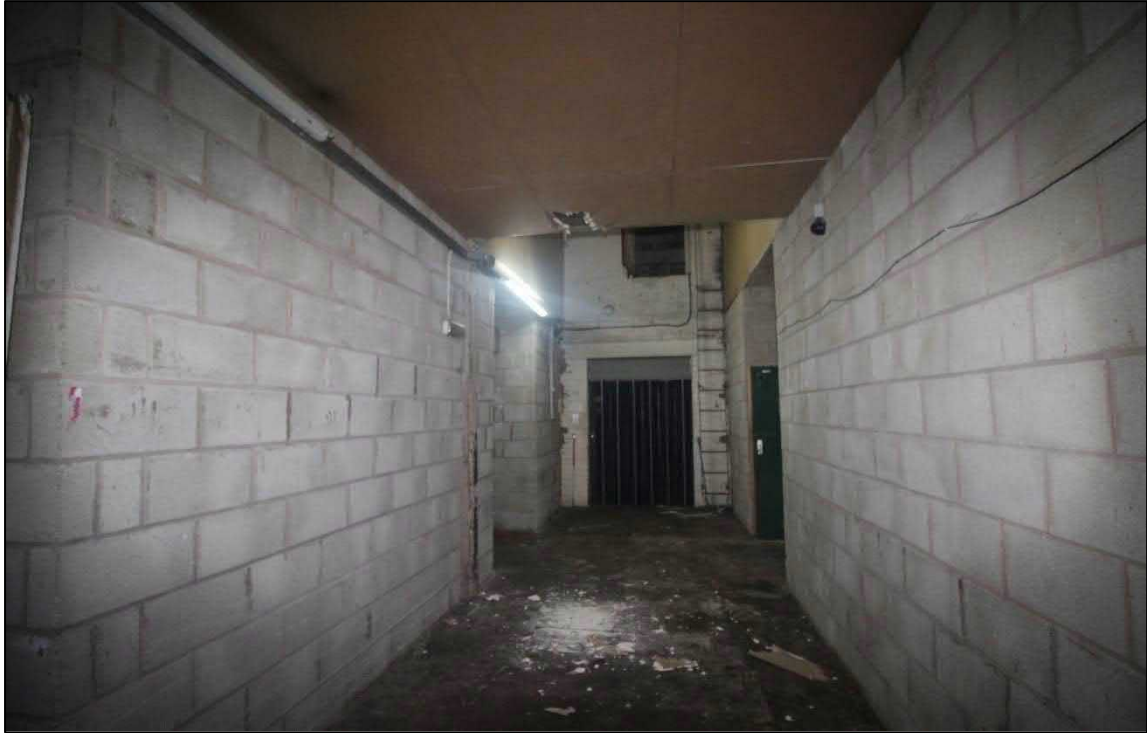
Plate 46: The corridor within southern staircase first-floor landing
