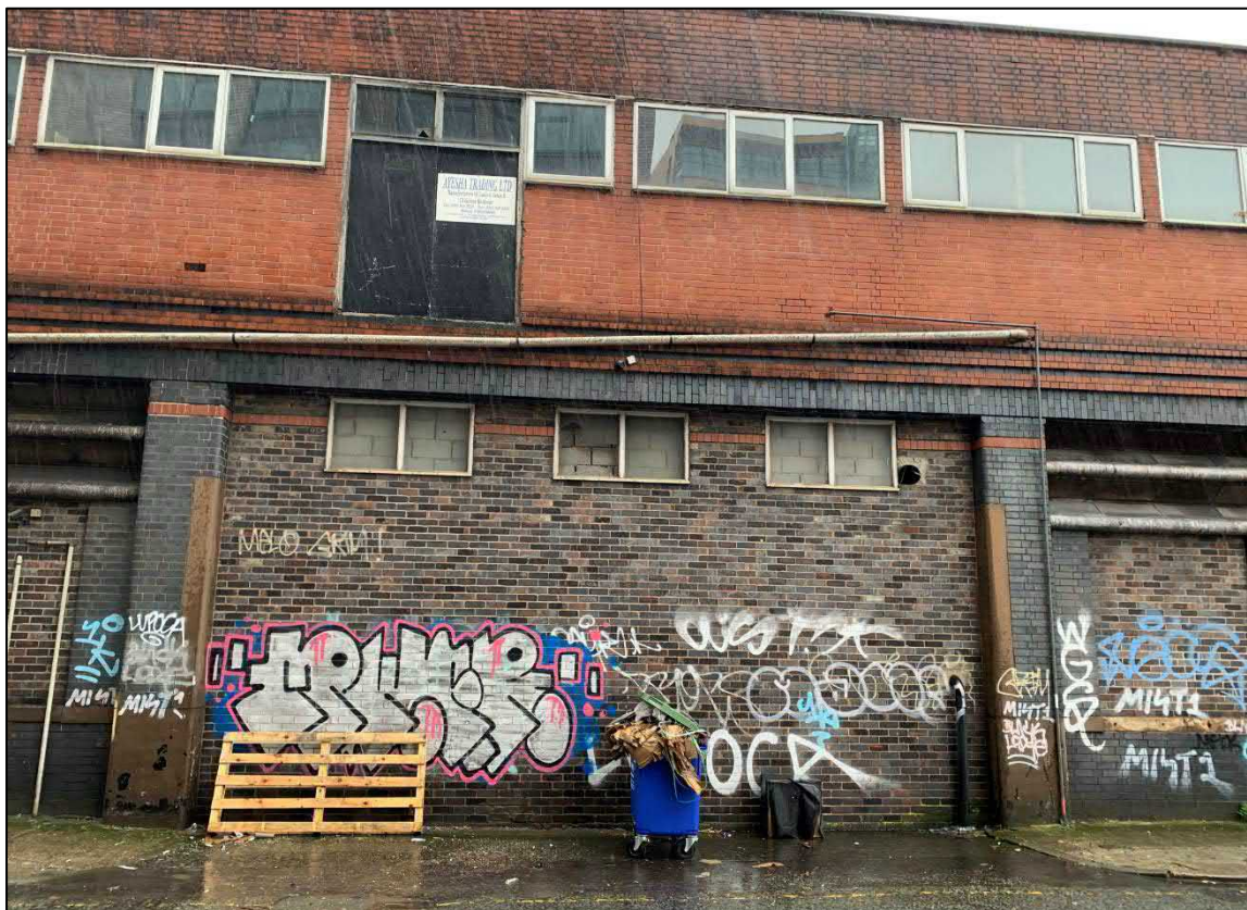
Plate 15: The central doorway within the north-eastern elevation
