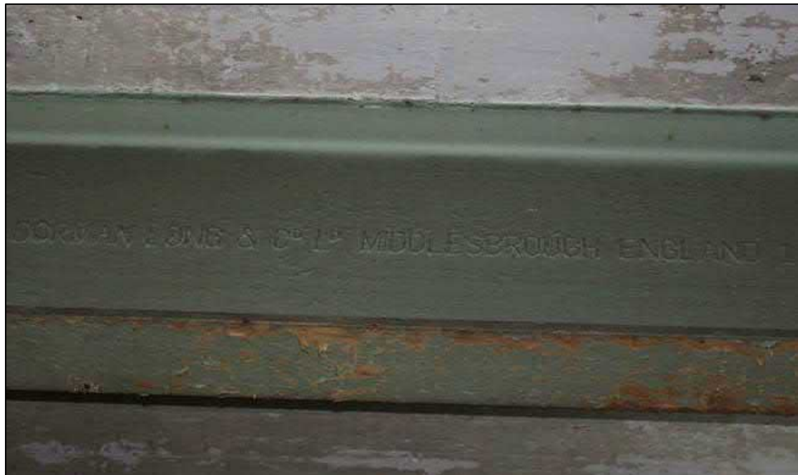
Plate 86: Detail of the roll stamp 'Dorman Long & Co Ltd Middlesbrough England'
