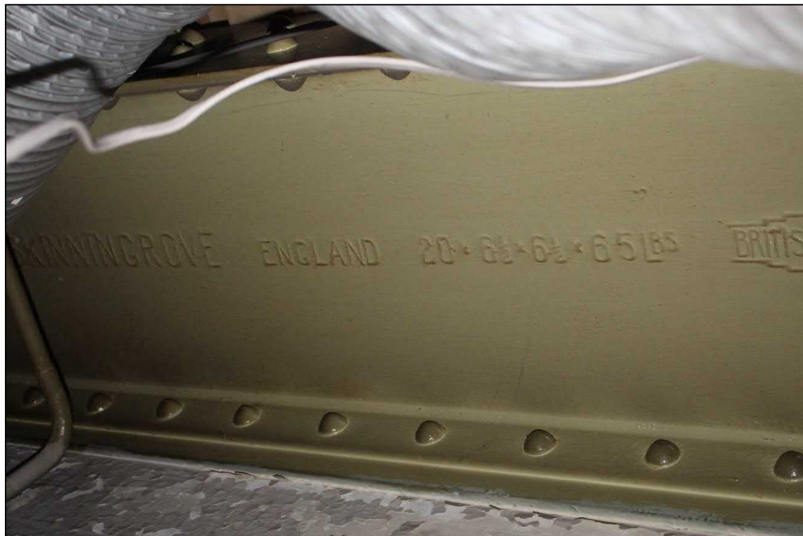
Plate 78: The rolling stamp of Skinningrove on the steel beams used in the later office block
