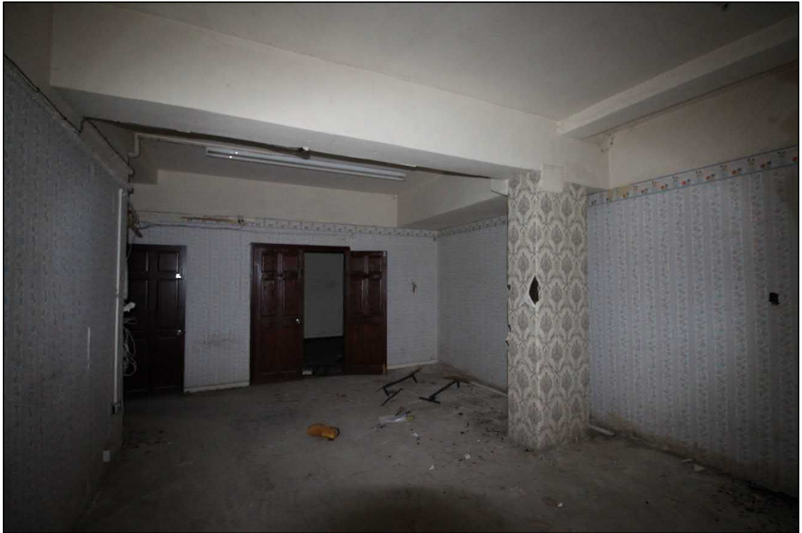
Plate 68: One of the northern offices within the basement of the office/warehouse block
