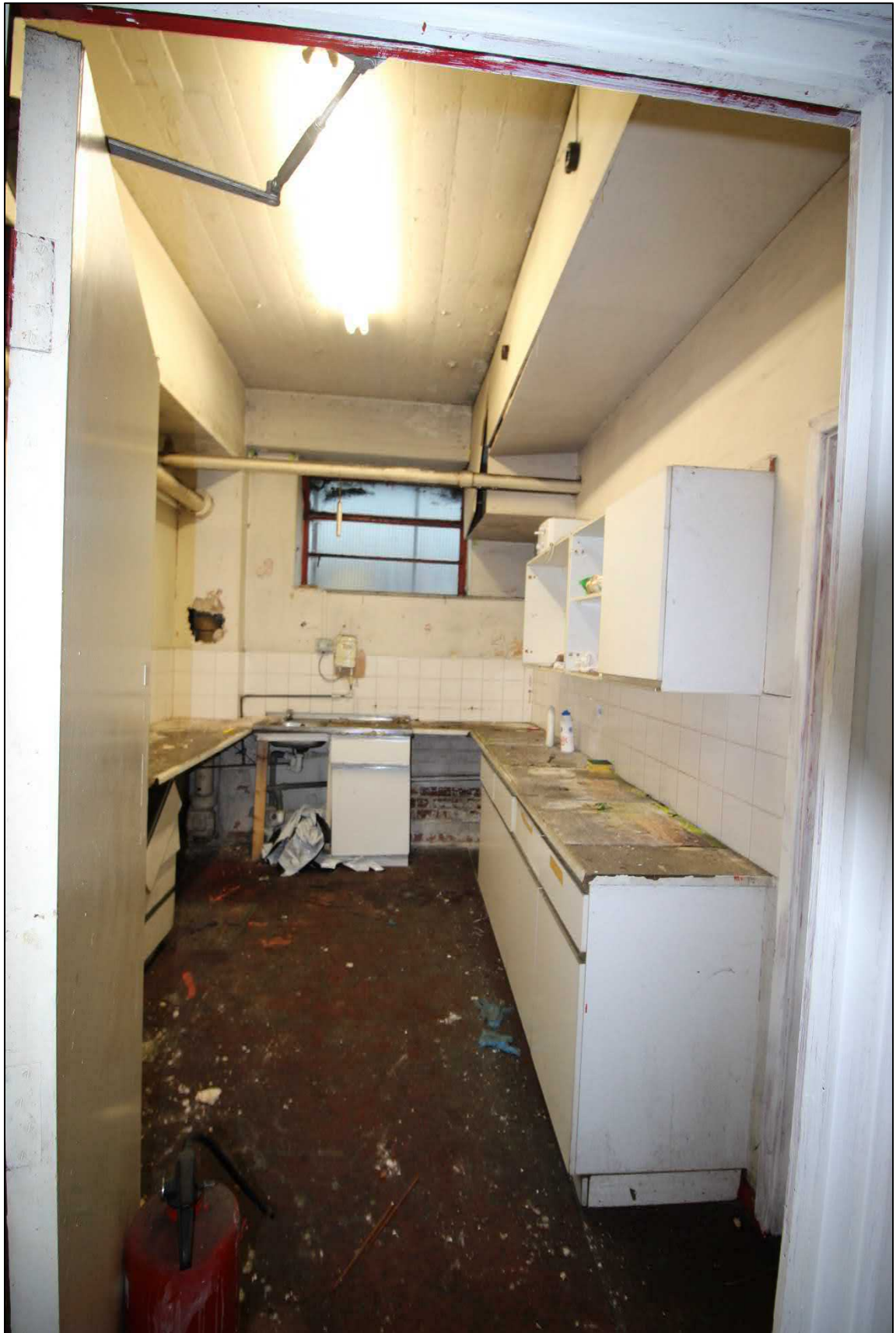
Plate 80: The kitchen at the northern end of the basement
