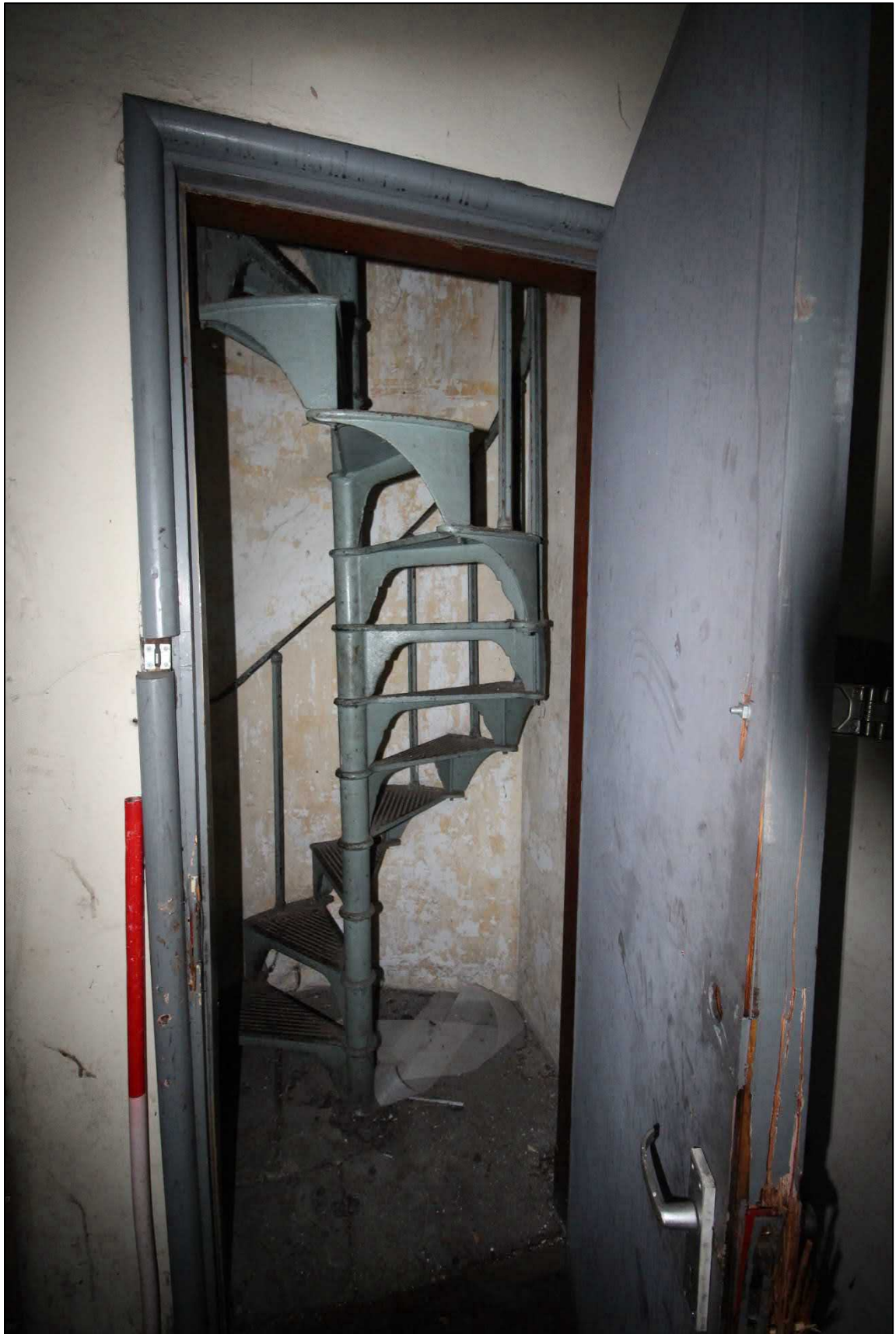
Plate 61: The spiral staircase leading to the roof space of the later office block
