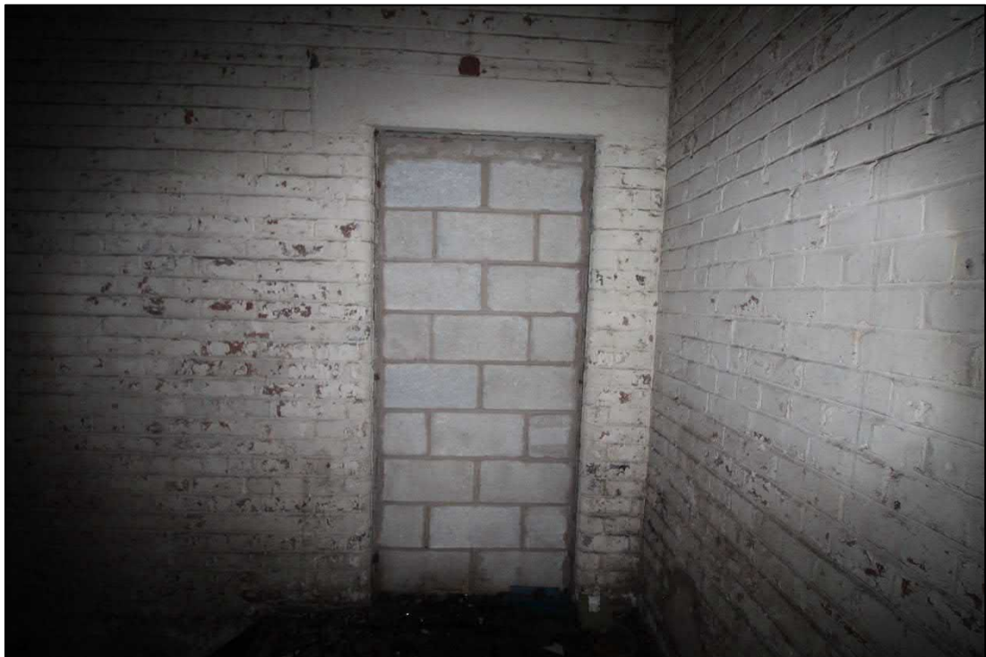
Plate 66: The doorway within the central stairwell originally giving access into the first-floor of the warehouse
