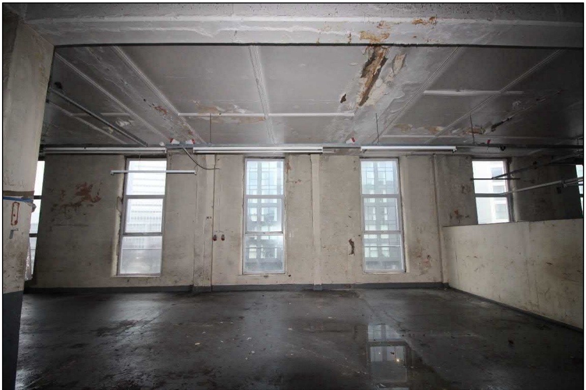
Plate 64: The north-western wall of the later office block
