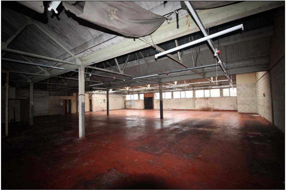
Plate 50: General view of the northern compartment on the first-floor of the warehouse
