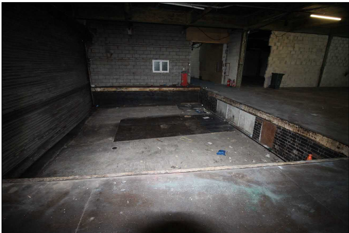
Plate 32: The loading-bay at the north-western end of the warehouse
