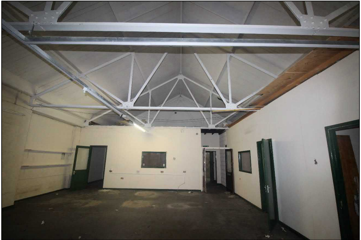
Plate 44: The northern end of the office showing the exposed fan trusses of the warehouse
