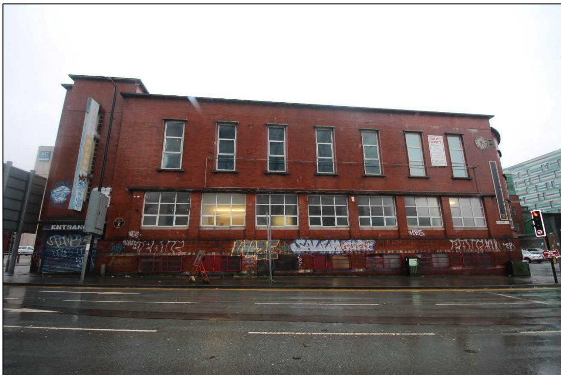
Plate 10: General view of the north-western elevation
