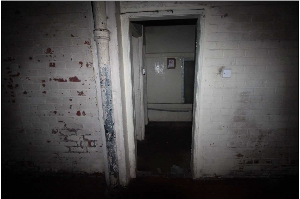
Plate 52: The doorway leading into the toilets within the north-western wall
