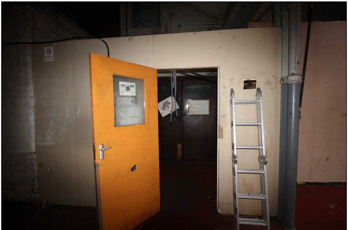
Plate 53: The doorway and partition wall of the northern lift lobby
