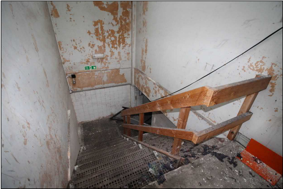
Plate 65: The southern stairwell of the later office block
