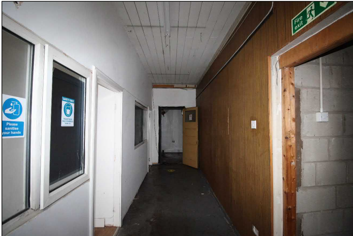
Plate 58: The northern corridor at the north-western end of the warehouse
