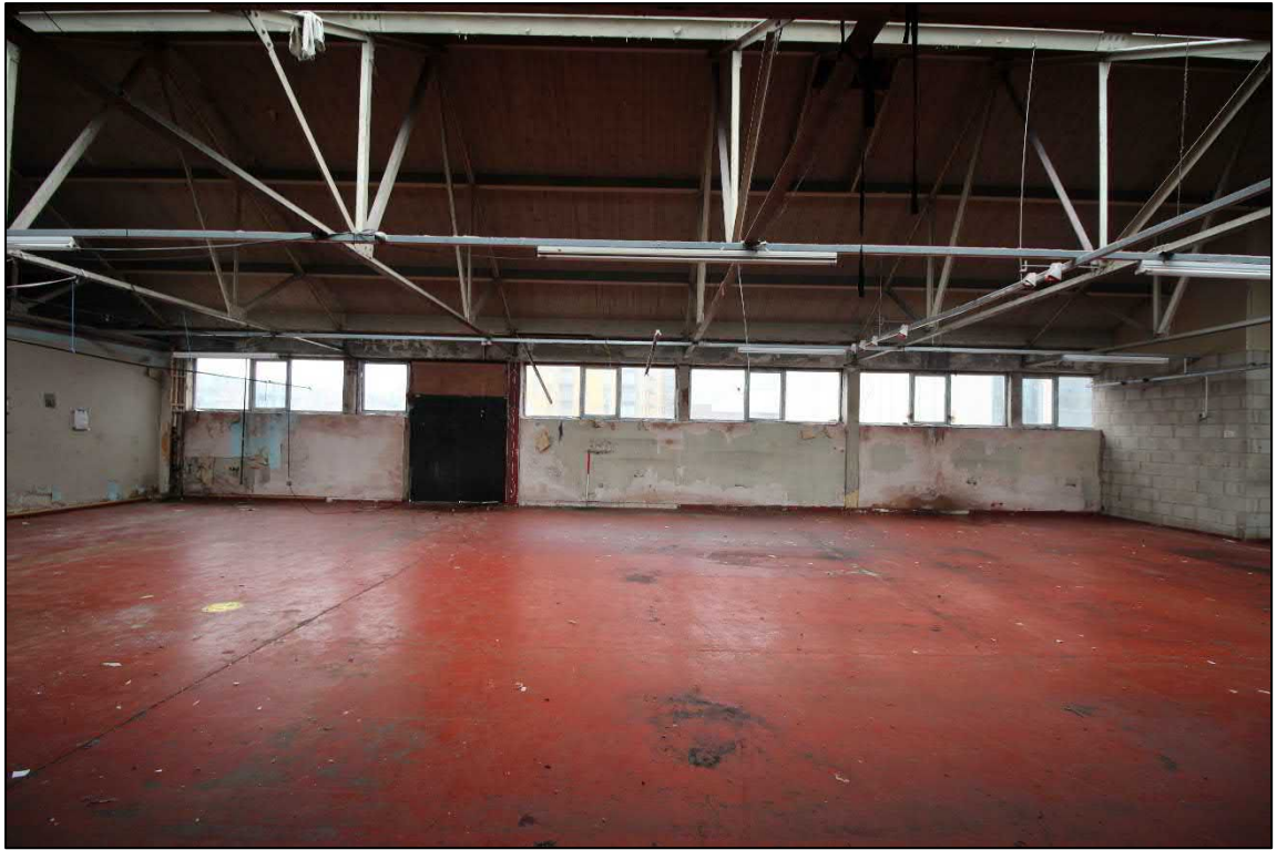
Plate 51: The north-eastern wall of the warehouse
