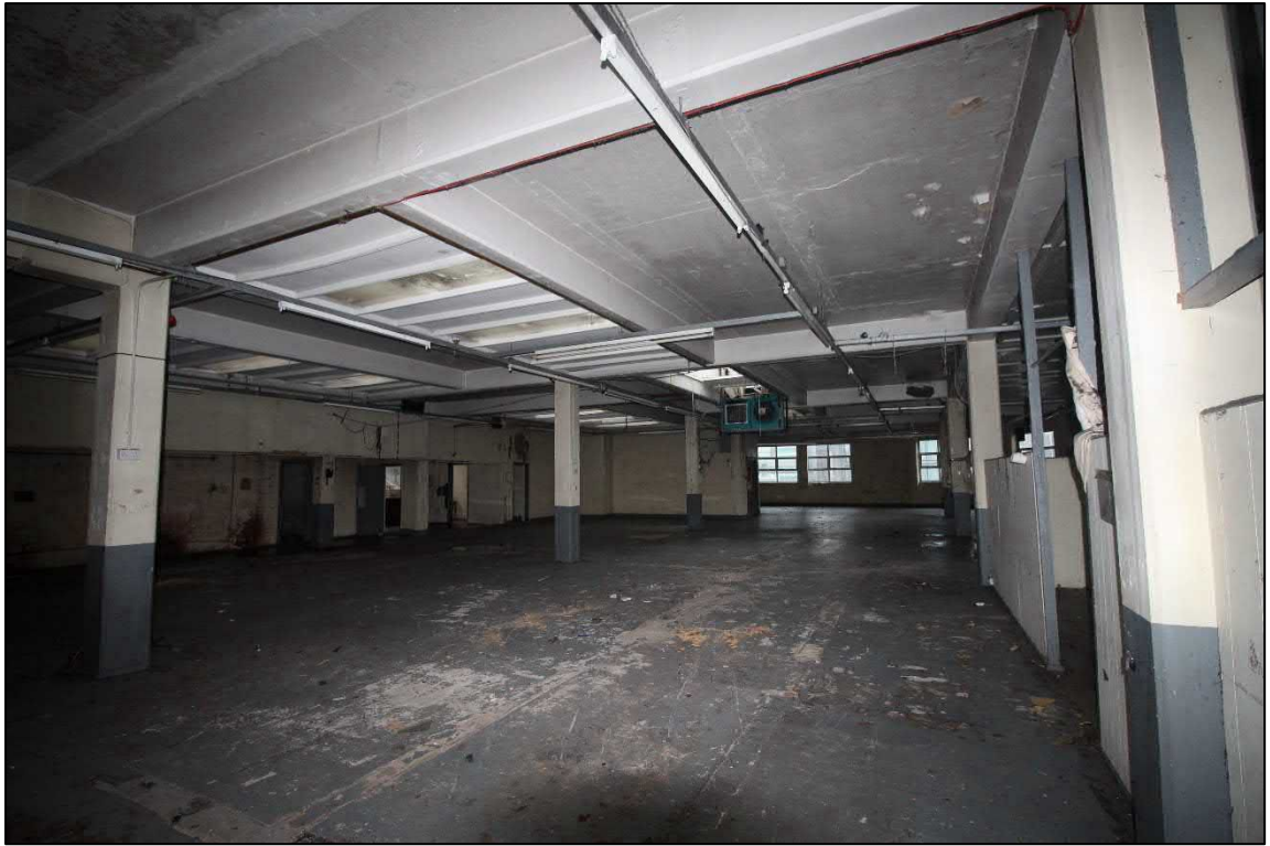
Plate 63: General view of the central room of the later office block
