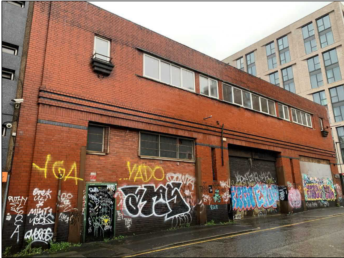
Plate 17: General view of the south-eastern elevation
