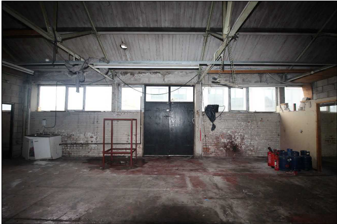
Plate 49: The north-eastern wall of the warehouse
