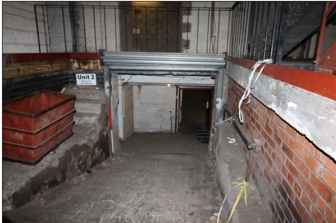
Plate 67: The doorway leading into the warehouse basement
