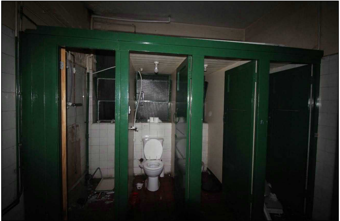
Plate 28: Detail of the timber toilet stalls within the basement of the office block
