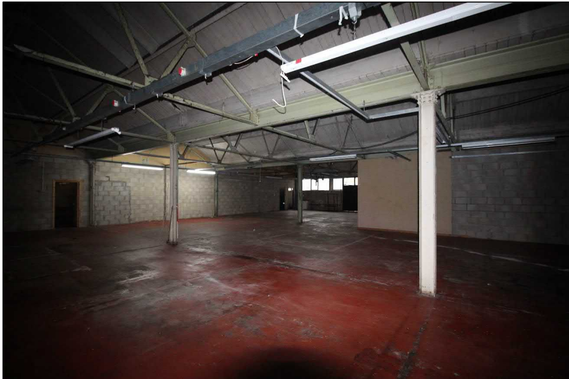
Plate 48: General view of the southern compartment on the first-floor of the warehouse
