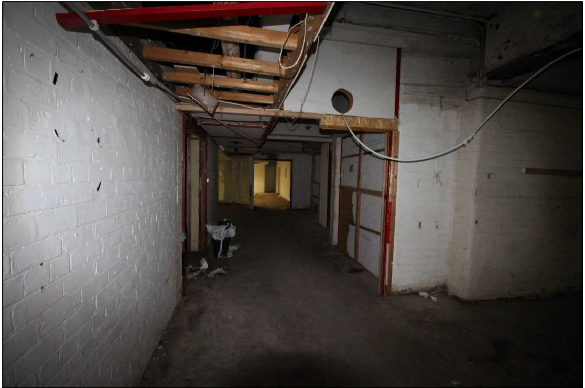
Plate 74: The doorway leading to the linking corridor between the buildings
