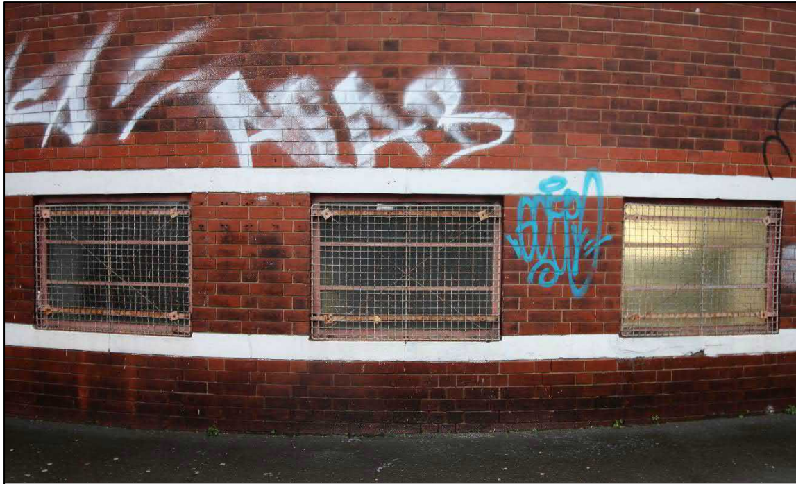
Plate 11: Detail of the basement windows on the north-eastern elevation
