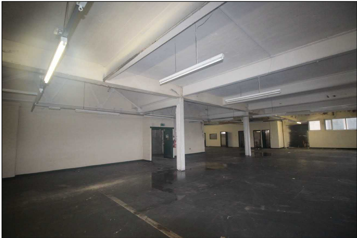
Plate 43: The first-floor of the office/warehouse block
