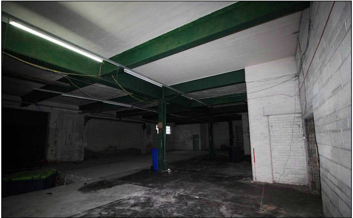
Plate 36: General view of the south-east compartment within the warehouse
