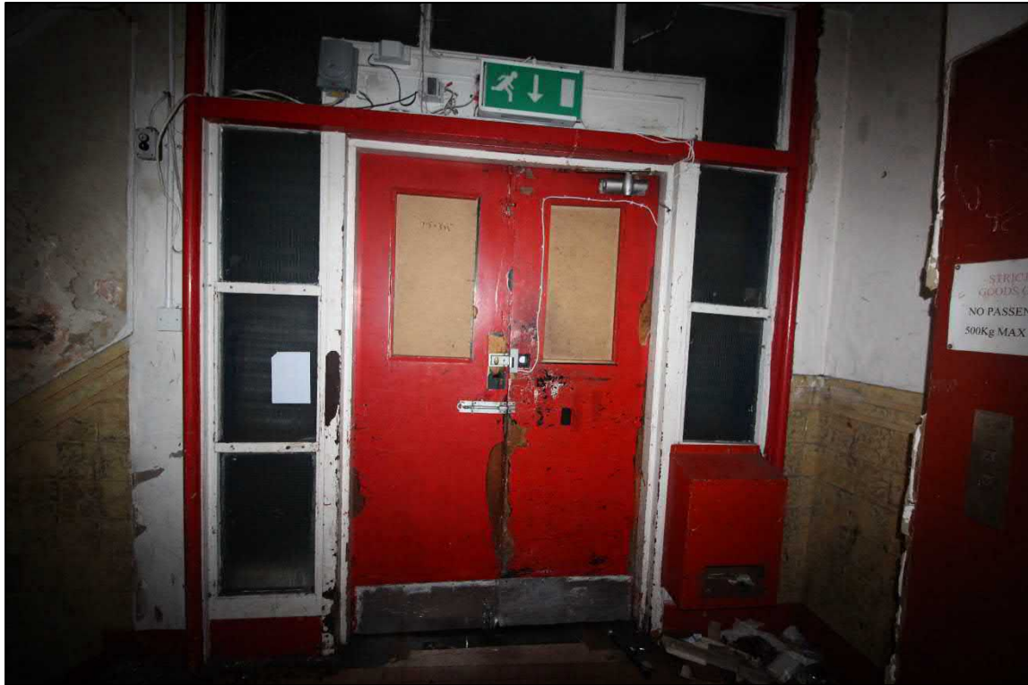
Plate 13: Detail of the timber doors behind the roller shutter
