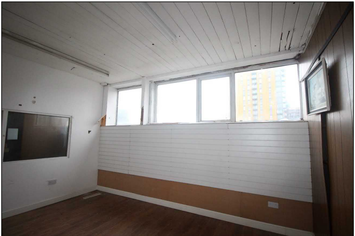
Plate 57: The north-eastern wall of the warehouse, detailing the altered windows
