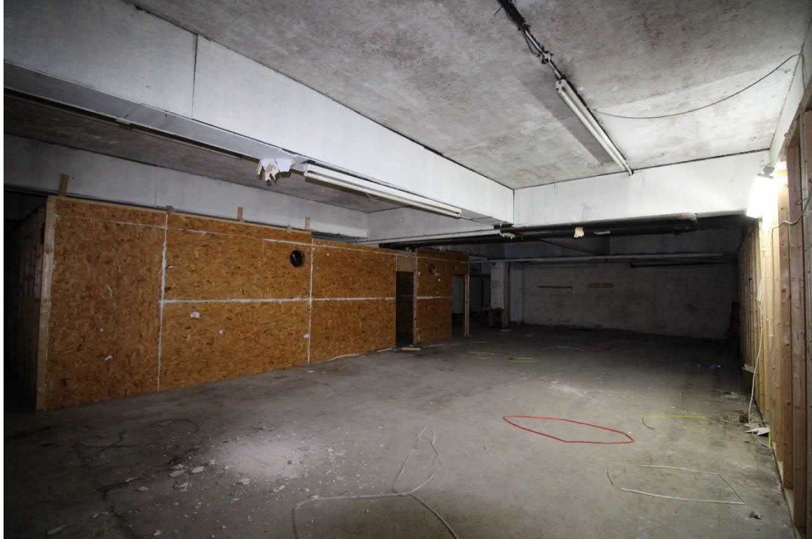
Plate 73: General view of the north-western room
