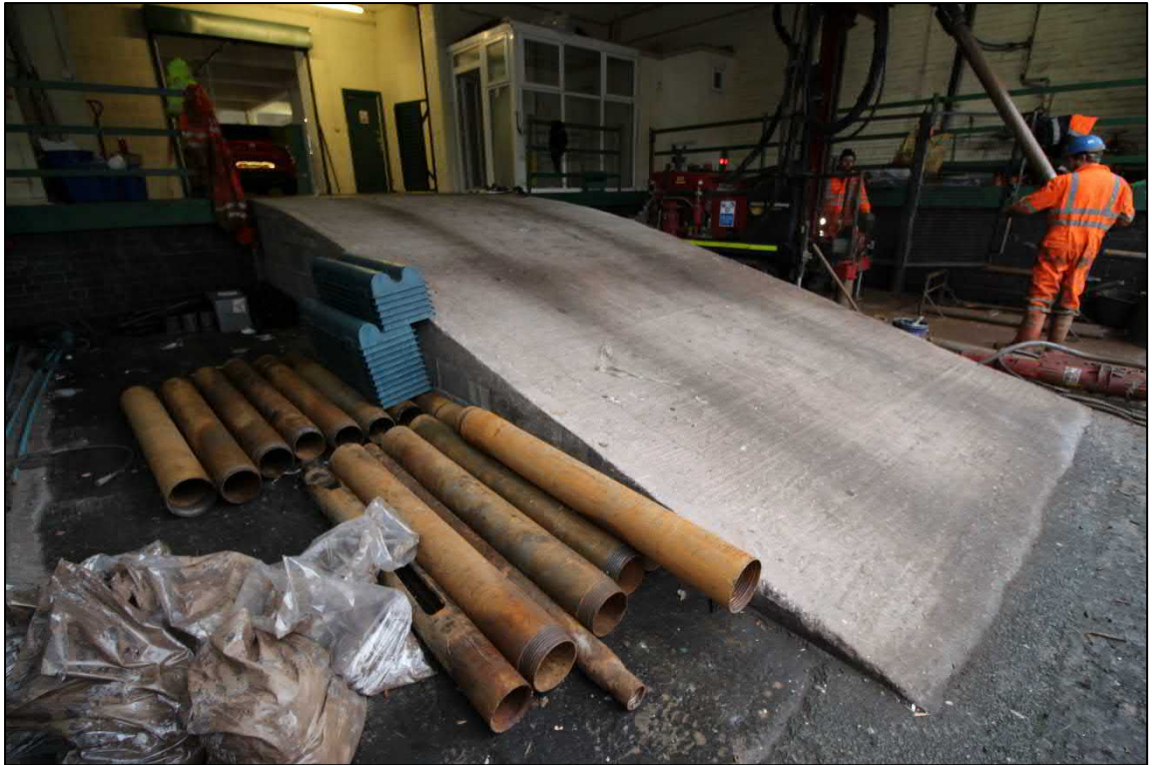
Plate 22: The concrete ramp at the centre of the north-western loading-bay
