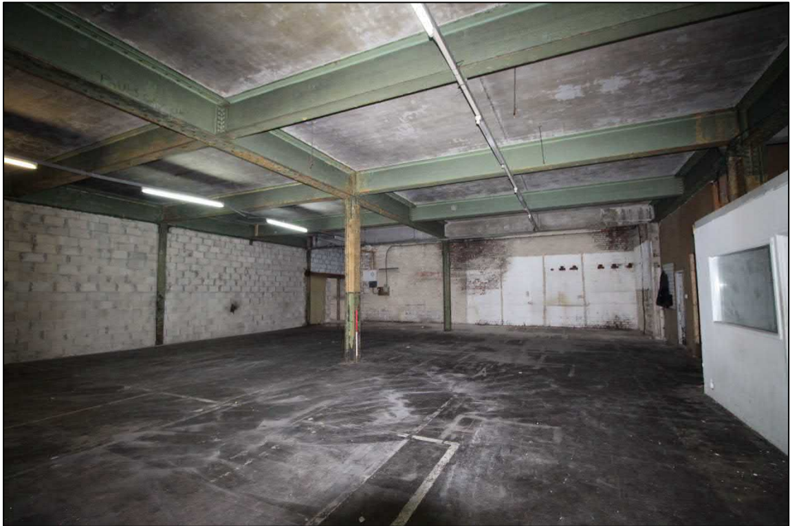
Plate 30: General view of the north-western end of the warehouse
