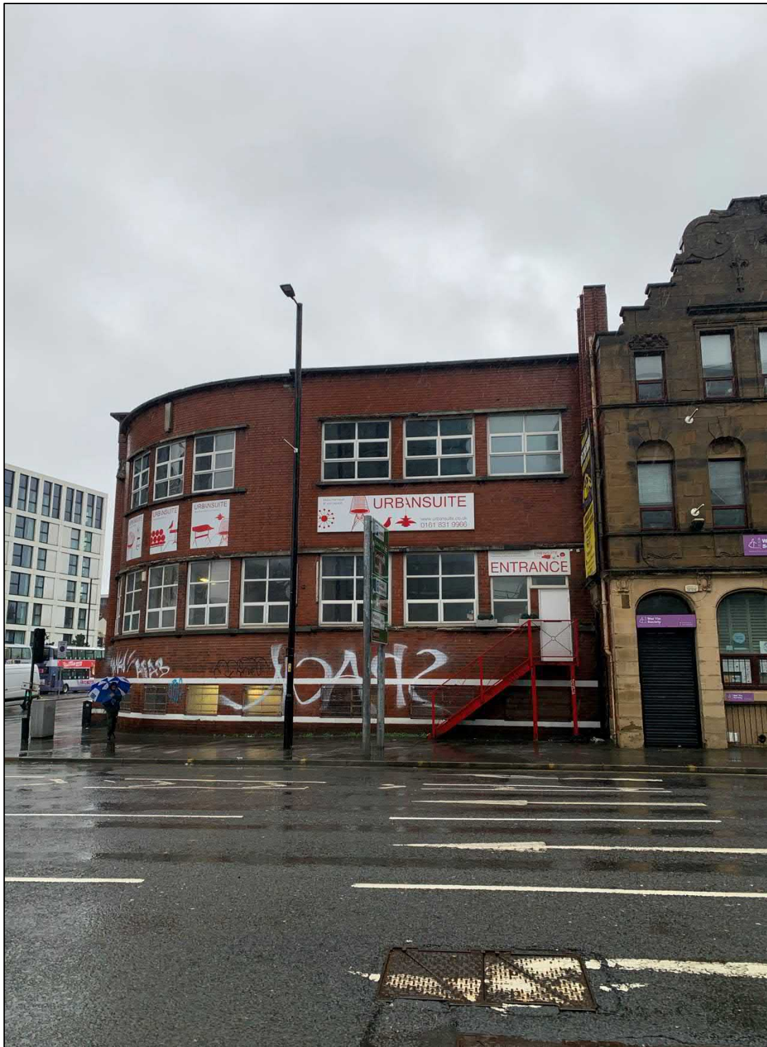
Plate 20: General view of the south-western elevation
