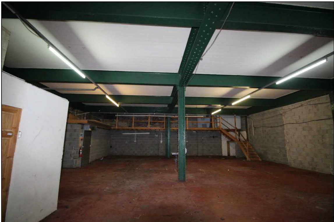
Plate 34: General view of the central compartment within the warehouse
