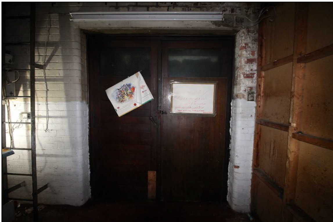
Plate 54: The lift doorway on the south-eastern wall of the lift shaft
