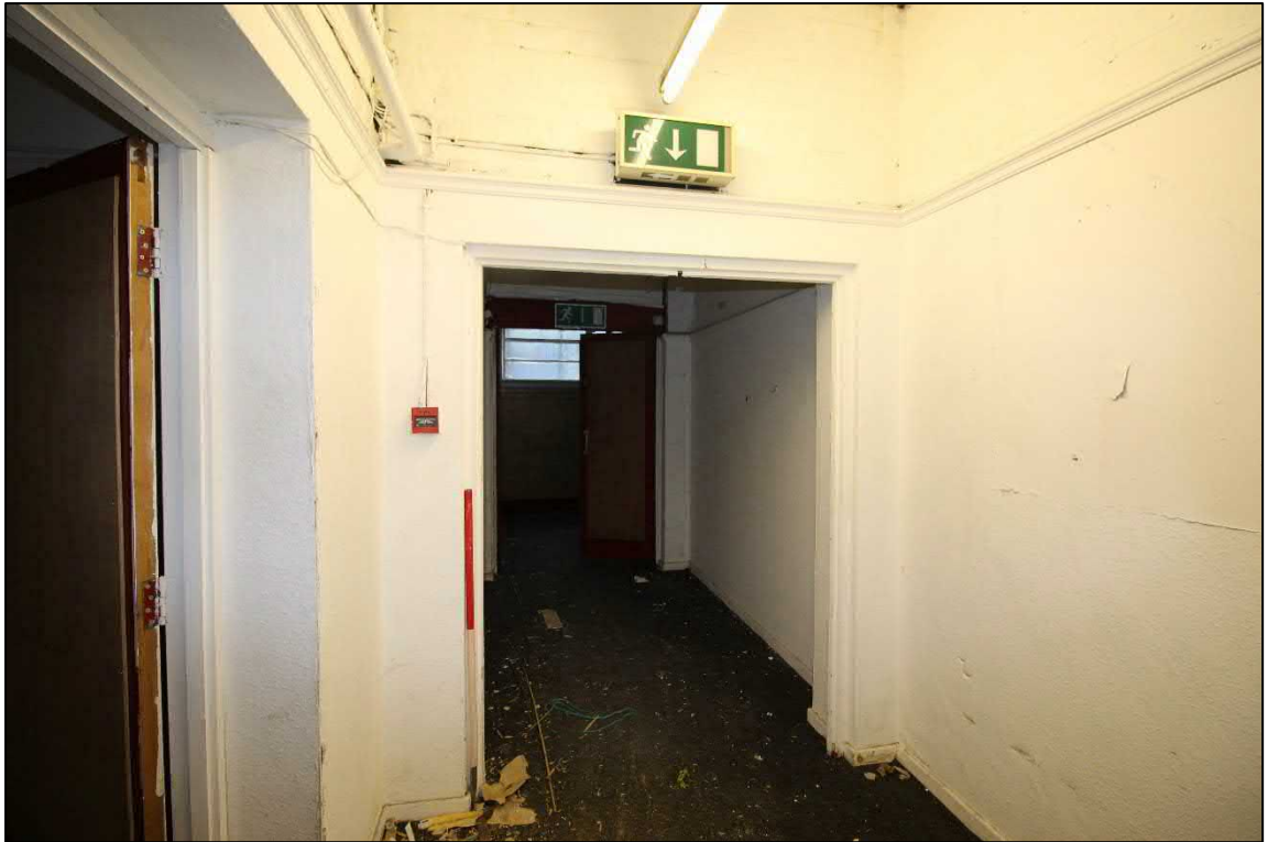
Plate 80: The north-east corridor of the basement
