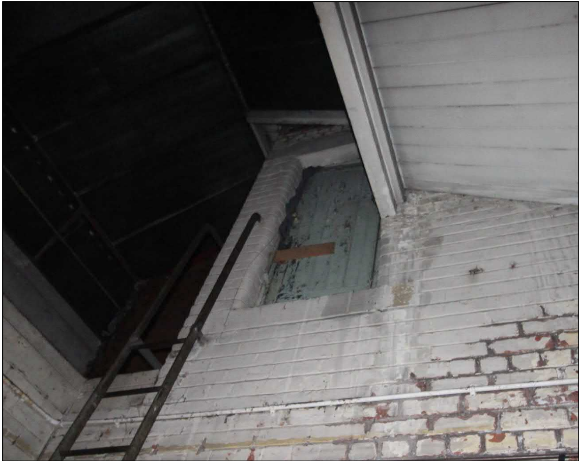
Plate 55: The doorway leading to the small room containing the lift winding gear
