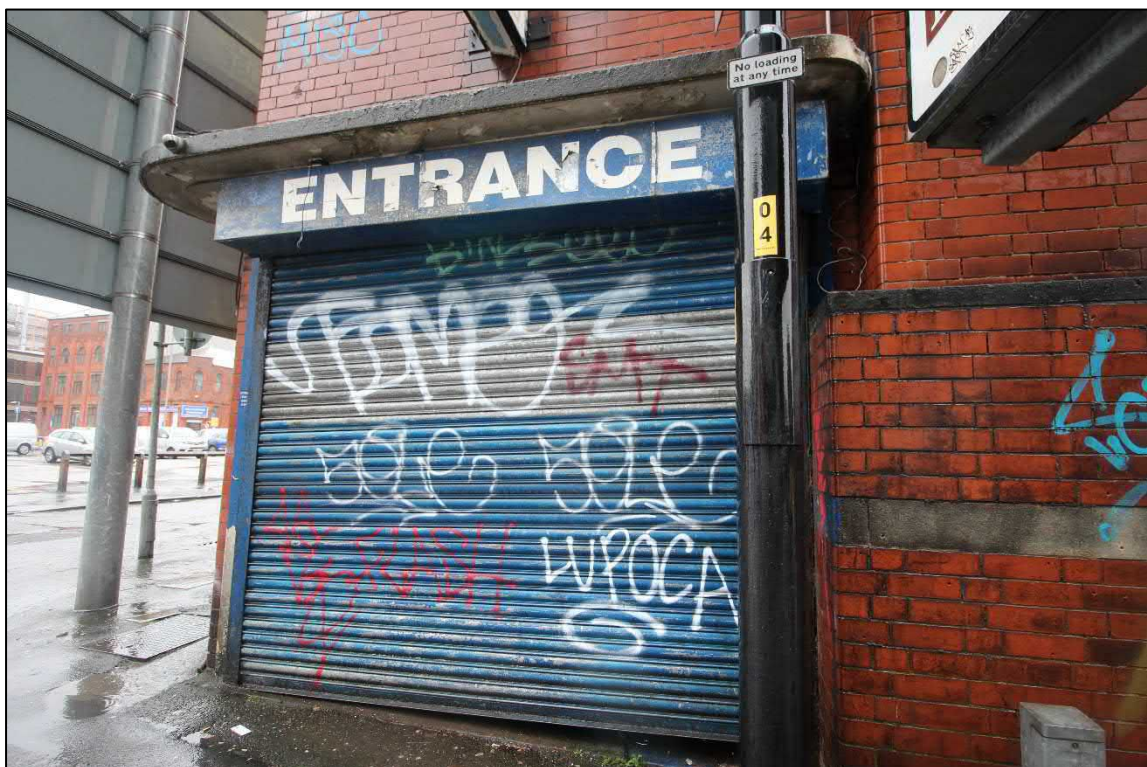
Plate 12: The roller shutter door at the north-eastern end of the elevation
