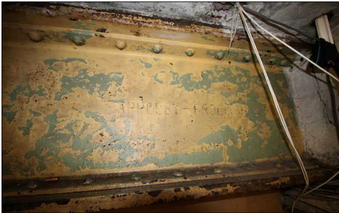
Plate 87: Detail of the roll stamp 'Appelby-Frodingham Iron & Steel Co. Ltd, England'
