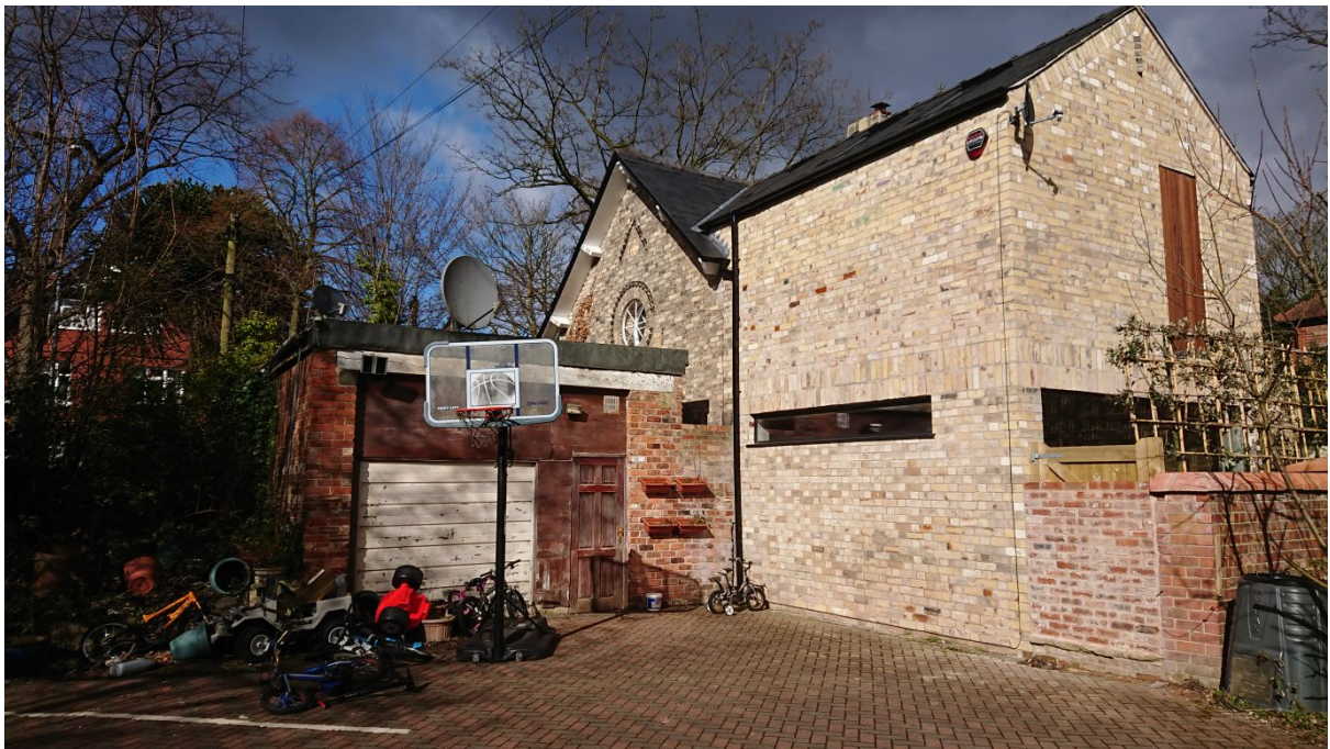
Figure 2. The garage in context of adjacent neighbour
