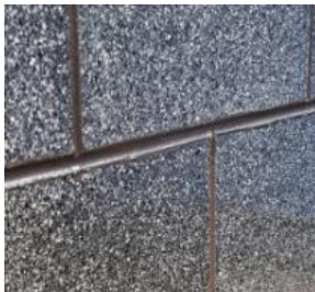
Pewter Block Mortar as mid grey and weather struck jointing quoin reveal and finished ends
