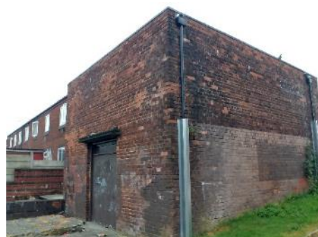
Figure 7: Substation on site
