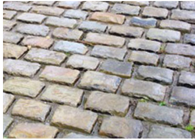
Lifted, cleaned and recycled cobbles
