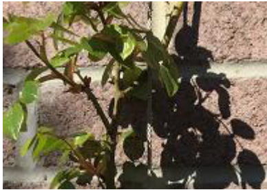
Trellis wire set in mortar joint
