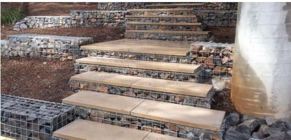
Retaining walls made from gabions
