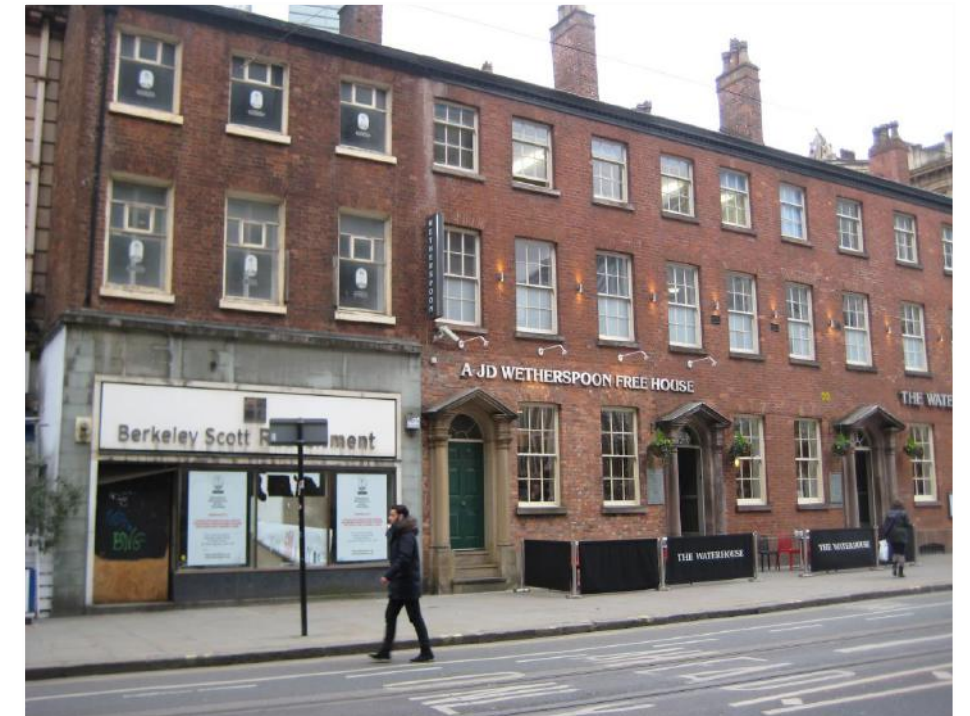
Fig. 04 Front elevation of the terrace of Georgian town houses from Manchester Town Hall.
