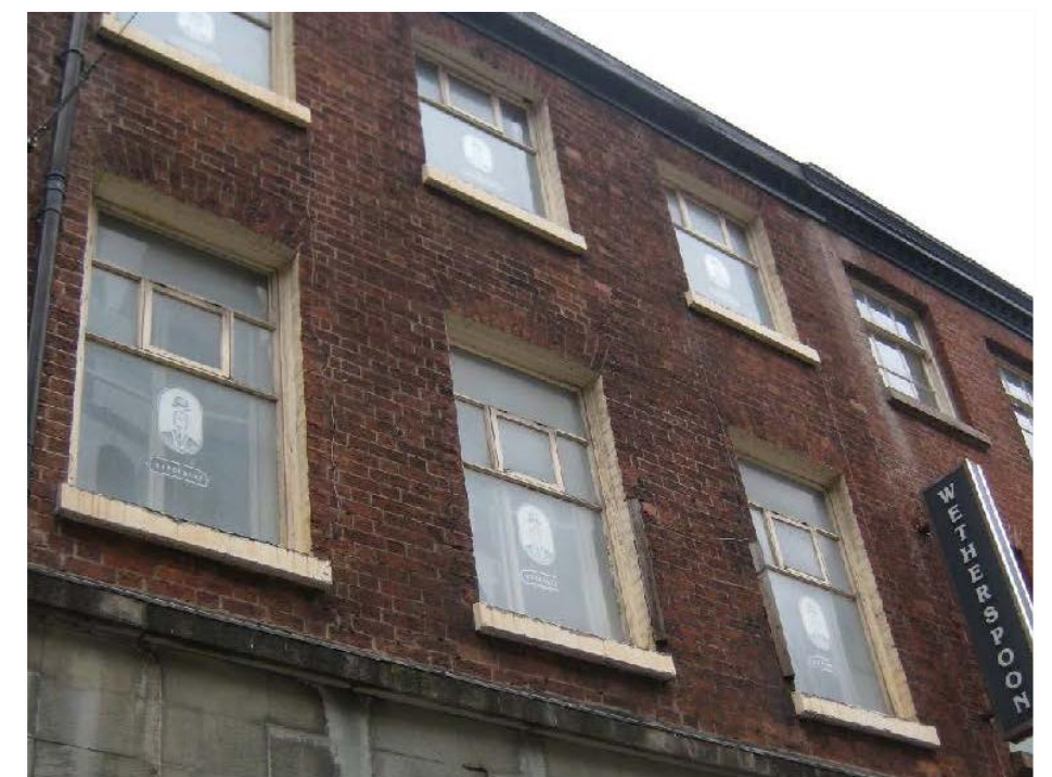
Fig. 06 Windows of 65 St Peter's Street.
