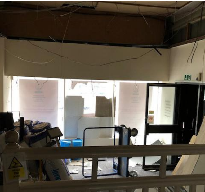
2: Floor to the front has been lowered with new steel and floor joists
