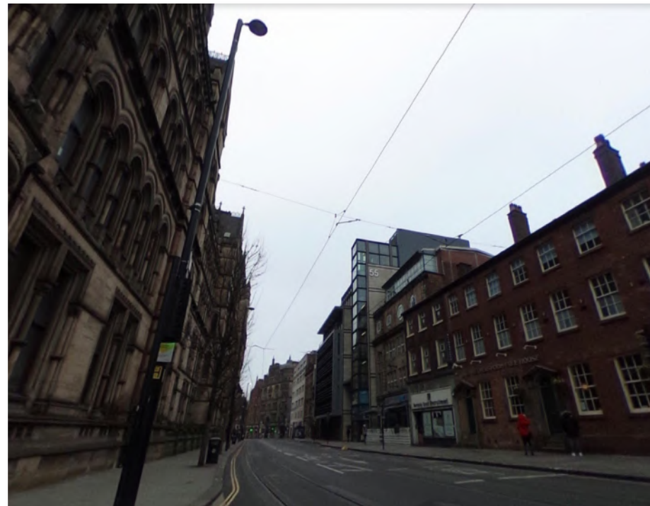
Fig. 03 Front elevation of the terrace of Georgian town houses from Manchester Town Hall.
