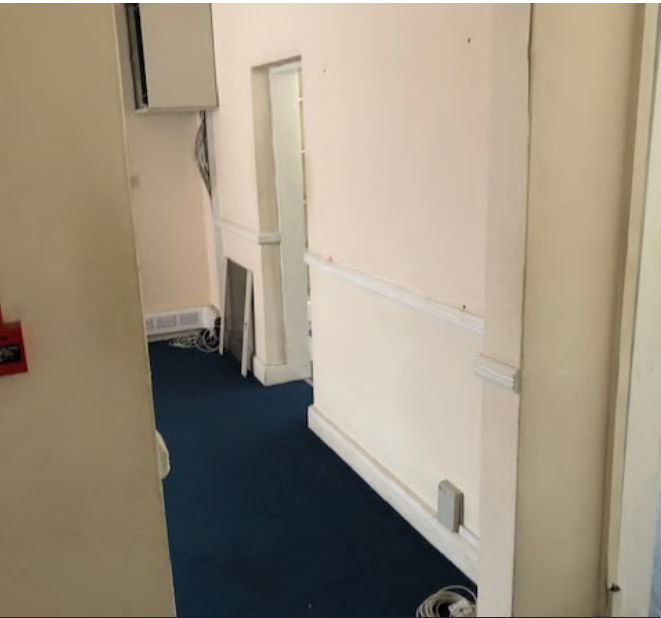
11: Original skirting and dado rail
