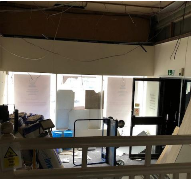
6: Balustrade not original
