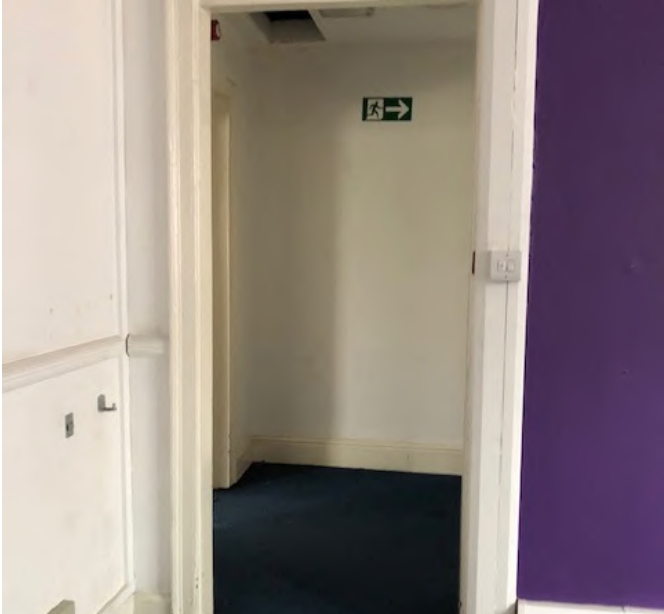
1: Original architrave dado and plain skirting, not original
