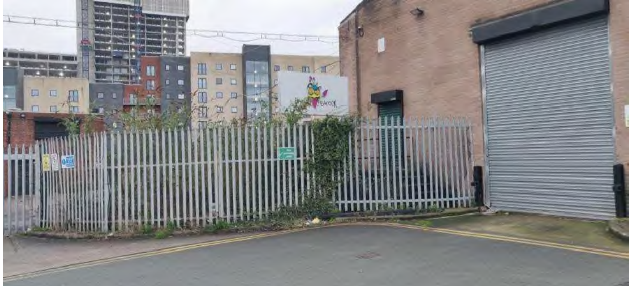
Fence on site boundary and overhead cabling. Note that the large building on the right is not included in the site boundary.
