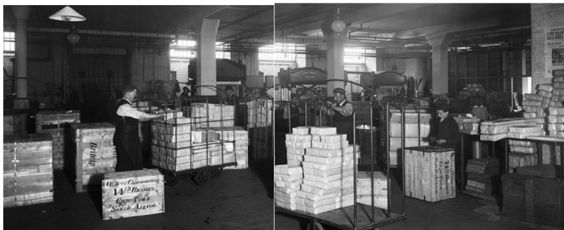
Figure 5: A photograph looking across the basement floor in 1900, illustrating the busy packing and shipping rooms, which predominantly occupied the basement area (this area does not form part of the current proposals).
