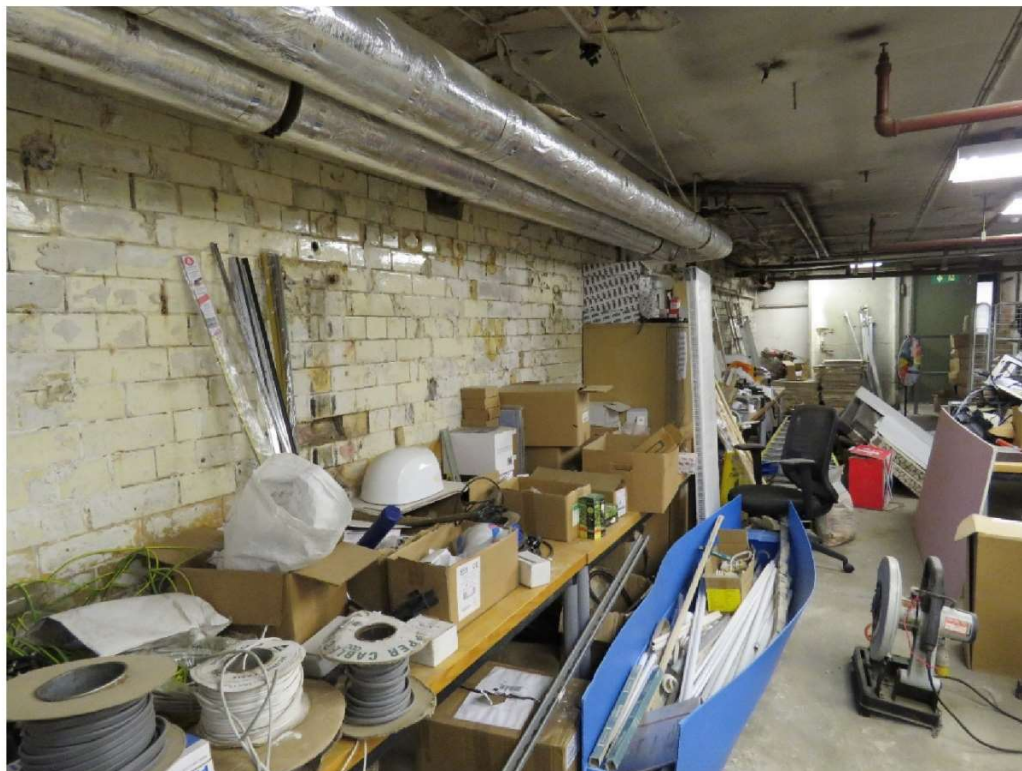
Figure 7: The now over-painted original tiling to the larger of the two store rooms.
