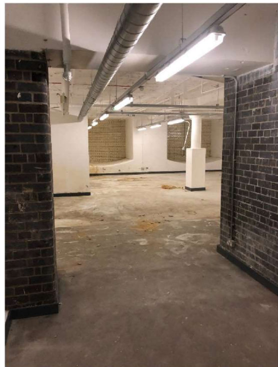
Figure 22: Looking into the sub basement level, showing the exposed and painted brick walls and central column.
