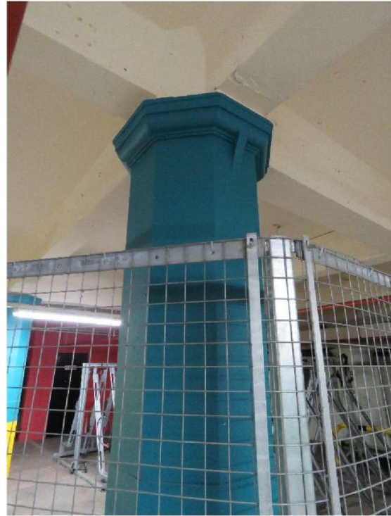
Figure 14: One of two designs of original concrete columns to the bike store area.
