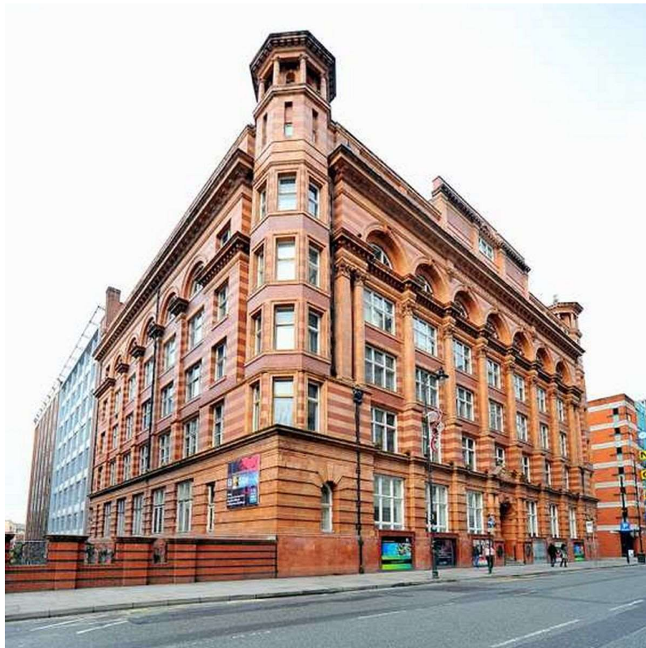
The Tootal Buildings from the corner of Oxford Road and Rochdale Canal.
