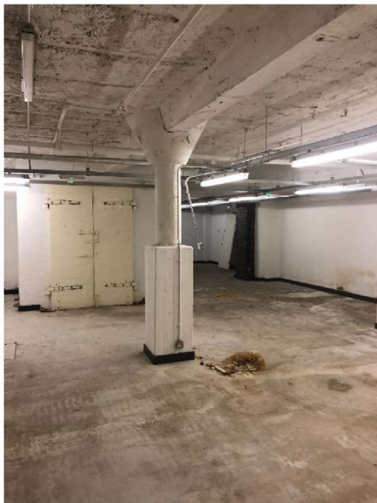
Figure 21: Another example of a structural concrete column and steel doors.
