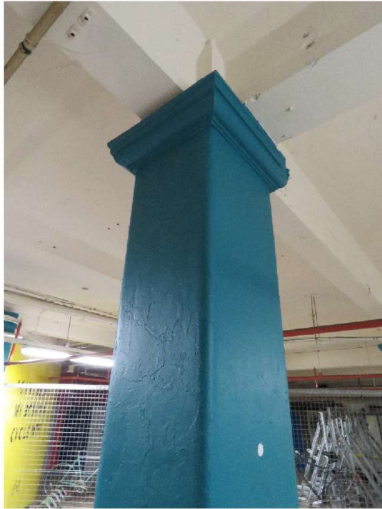
Figure 13: One of two designs of original concrete columns to the bike store area.
