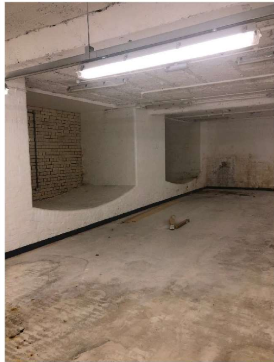
Figure 20: A corner of the sub basement illustrating the base of the former basement lightwells from the above basement floor. Note the exposed glazed brick.
