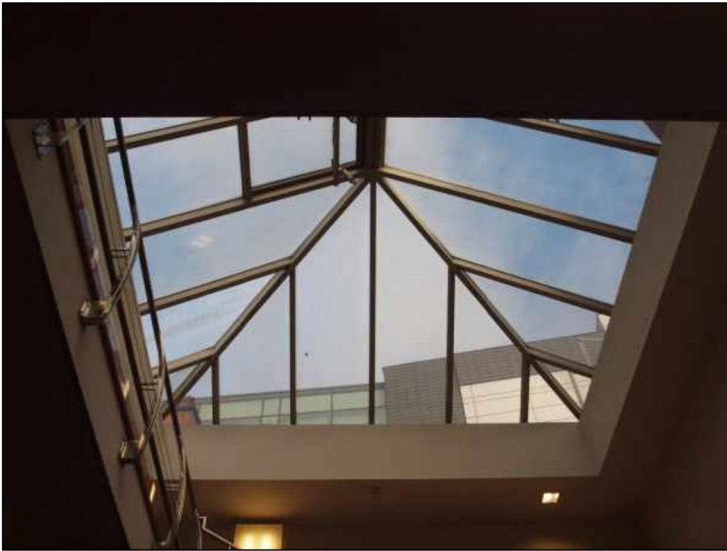
Plate 31: Modern skylight above main staircase
