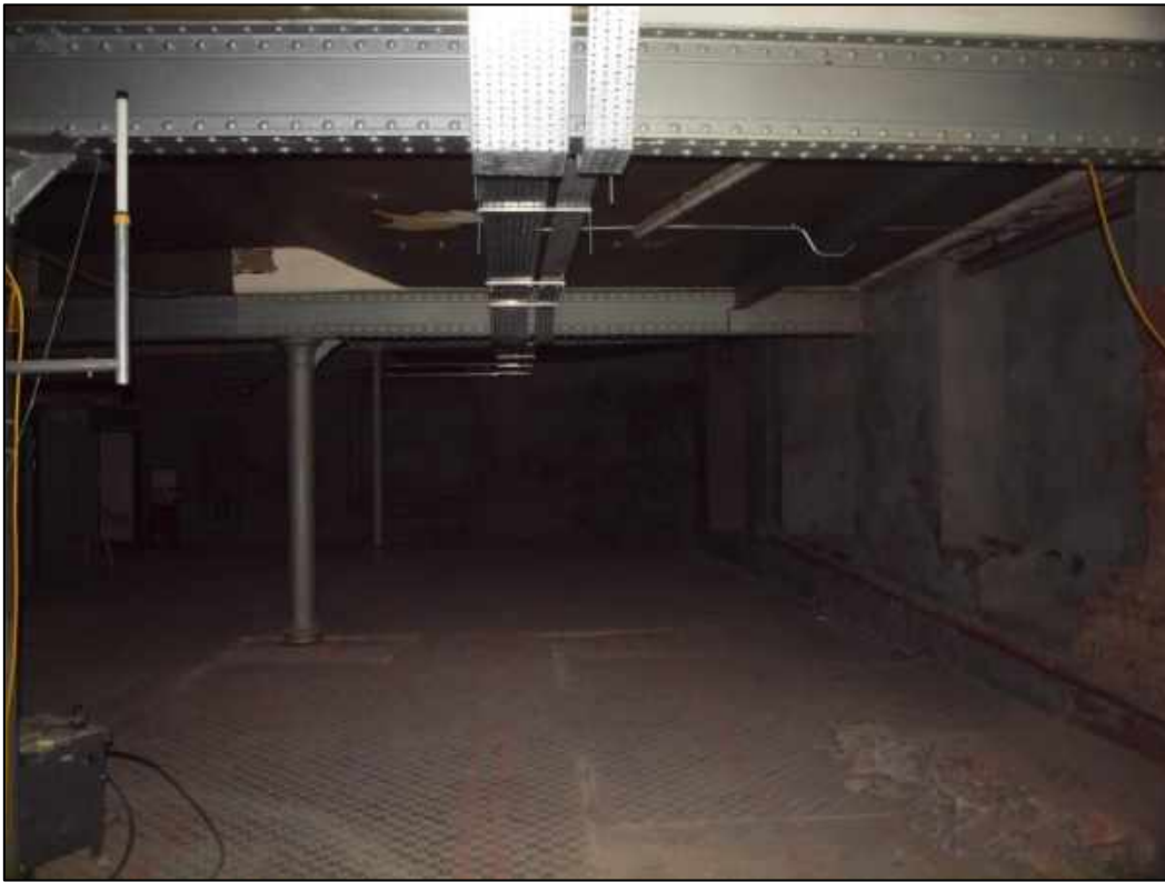
Plate 15: General shot of basement southern end
