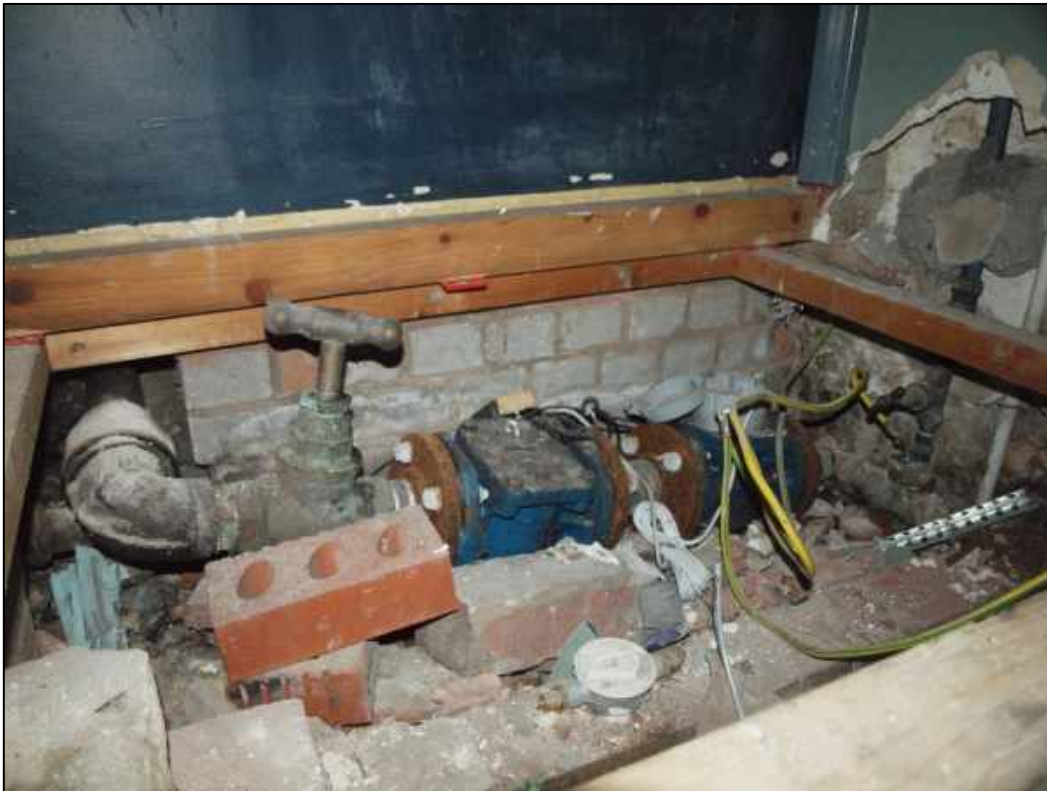
Plate 25: Lightwell showing location of mains water pipe
