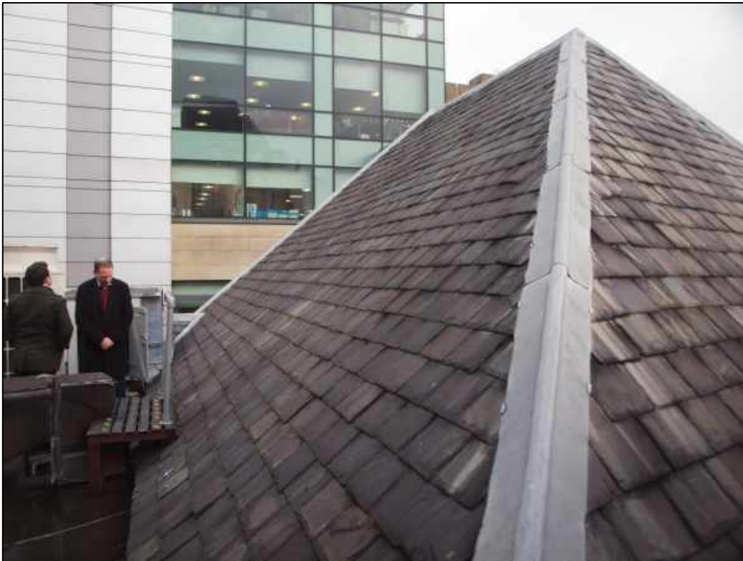
Plate 33: Detail of pitched roof
