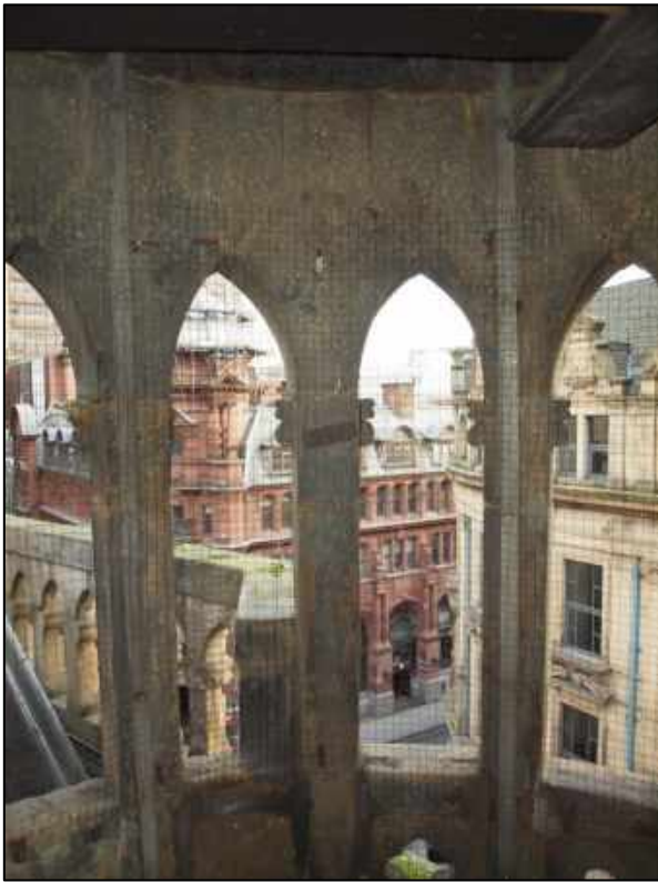
Plate 37: West turret as viewed from inside
