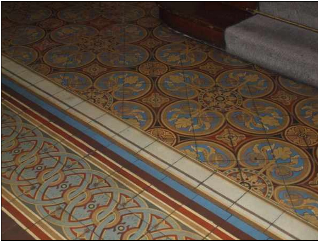
Plate 11: Detail of tiled floor
