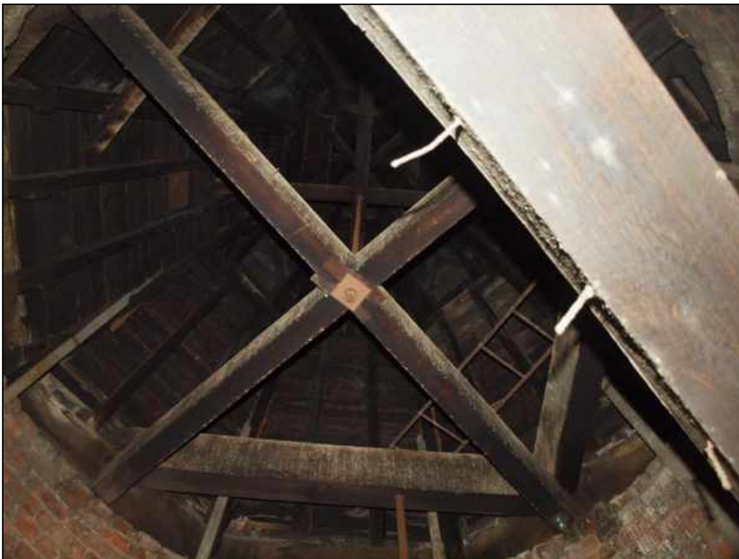
Plate 38: Detail of timber roof structure
