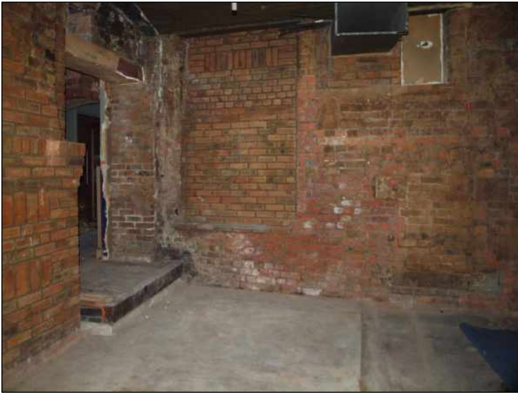
Plate 29: North wall of east room showing blocked window into yard
