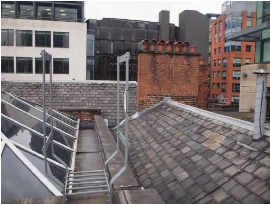
Plate 35: General shot of the roof showing partially rebuilt chimney stack
