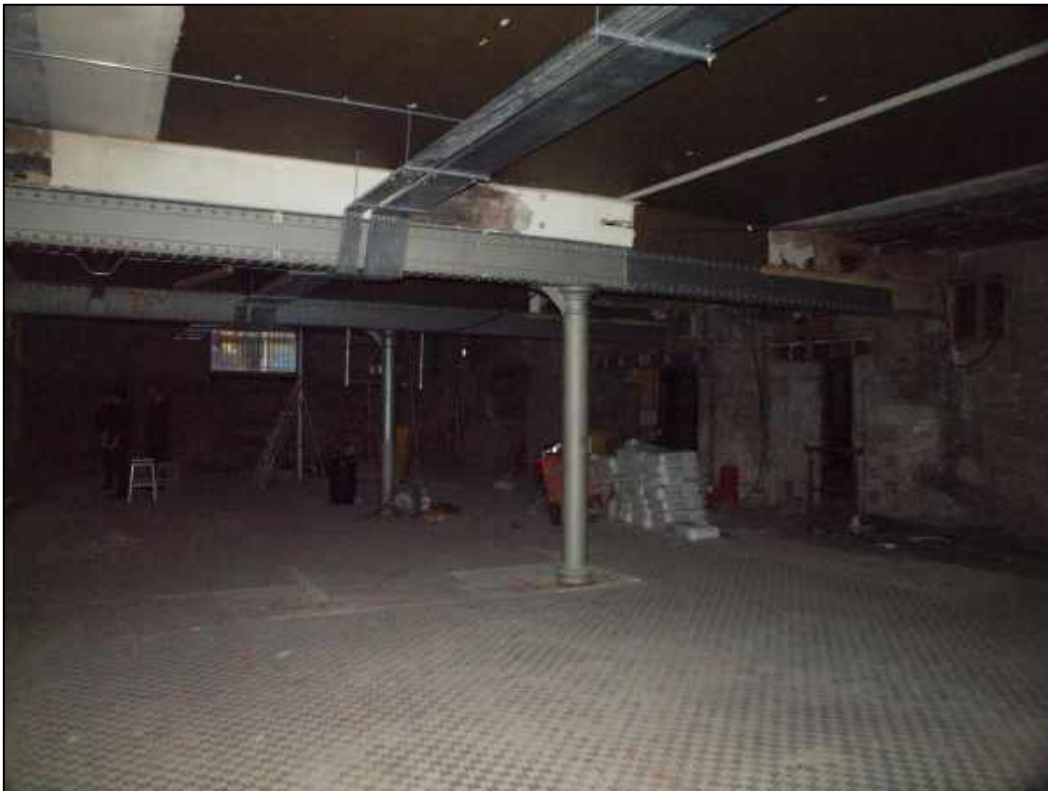
Plate 18: General shot of basement
