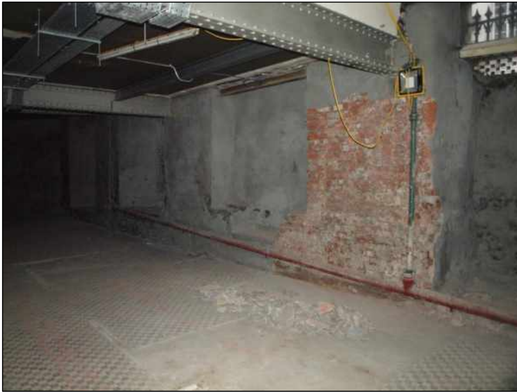
Plate 19: Section of removed render exposing brickwork
