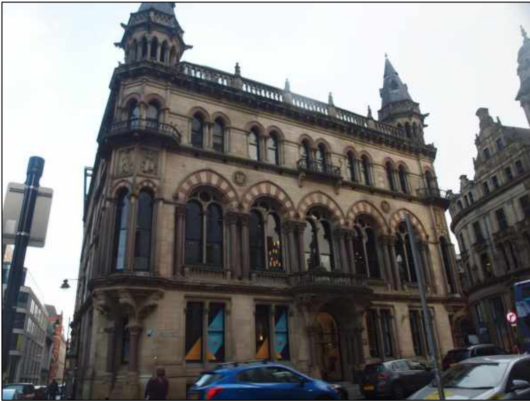
Plate 3: Detail of the King Street elevation
