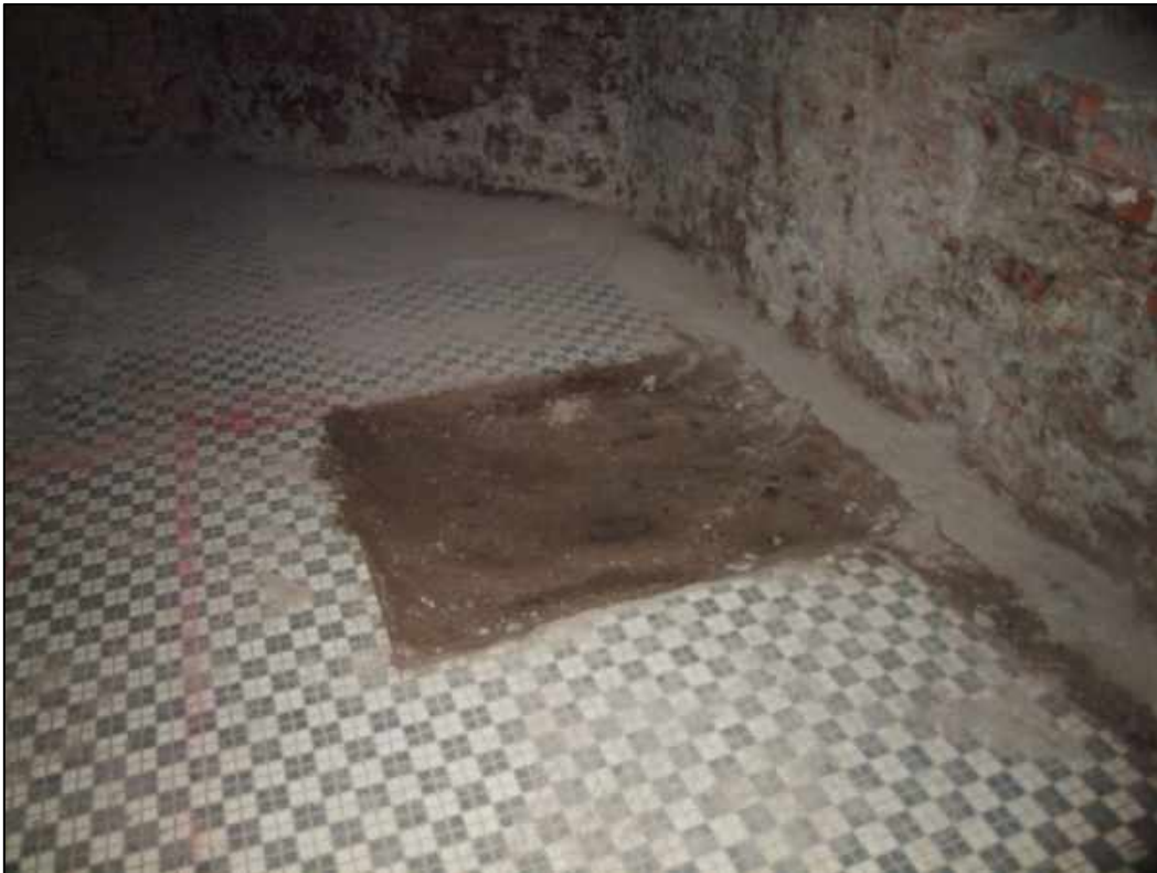
Plate 23: Detail of removed flooring revealing earth beneath
