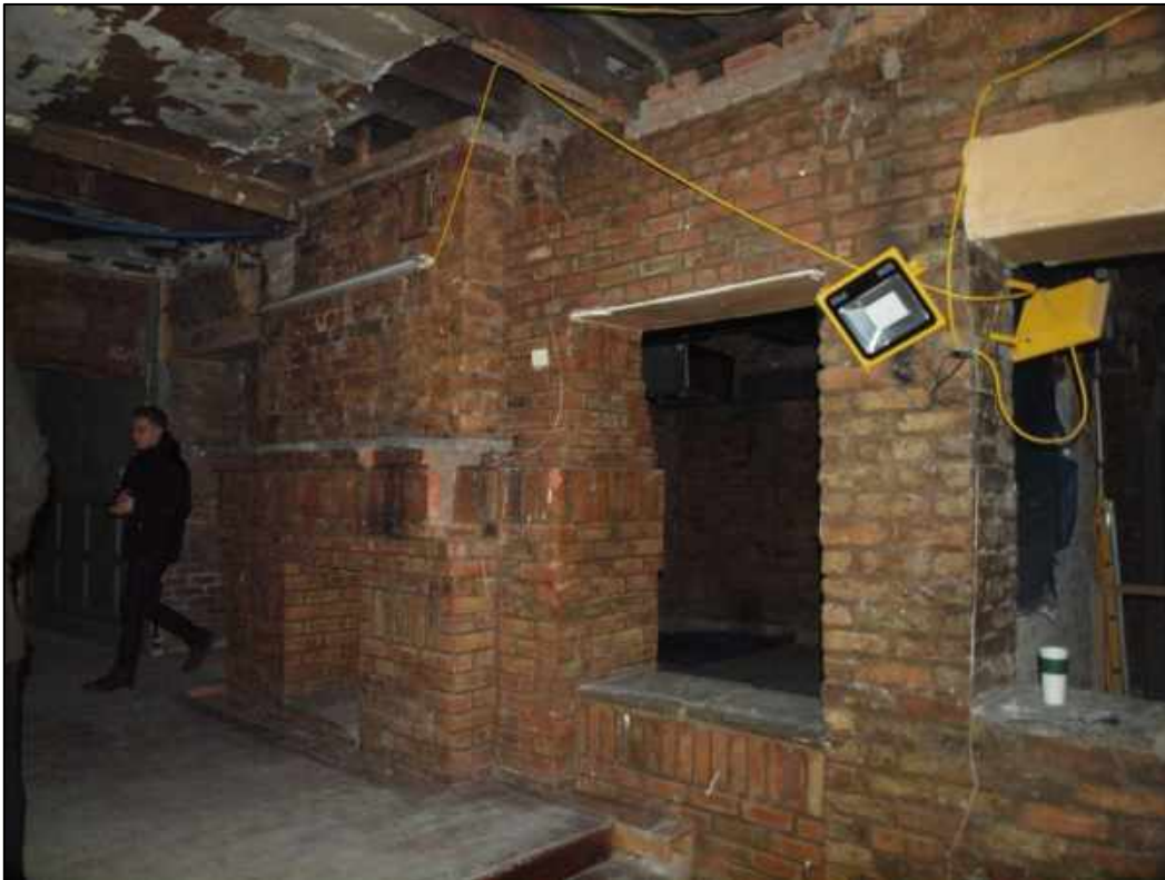
Plate 27: Inserted wall and fireplace dividing it from room to the east
