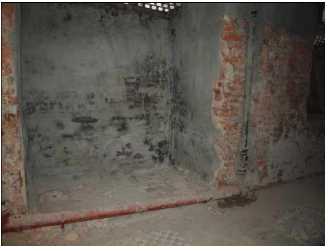
Plate 20: Detail of lightwell with base removed
