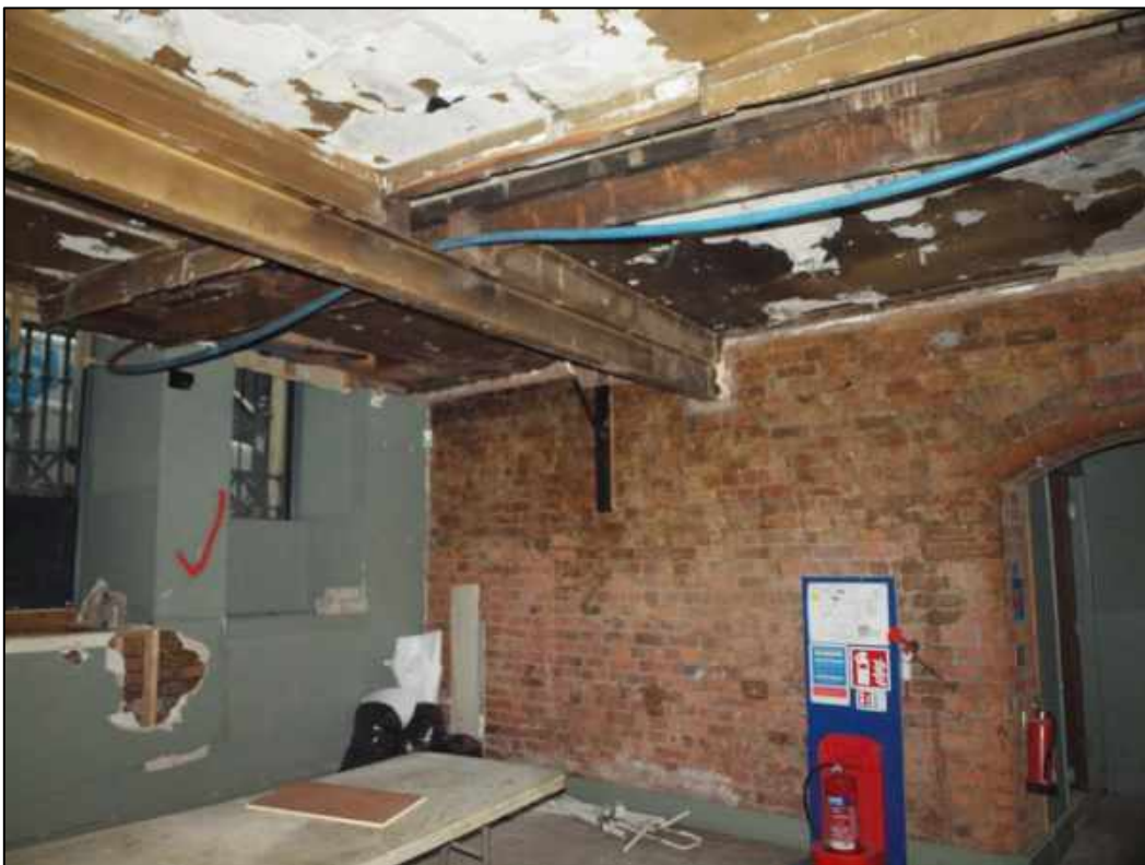
Plate 24: Northwest side of basement showing lightwells and temporary water pipe (blue)
