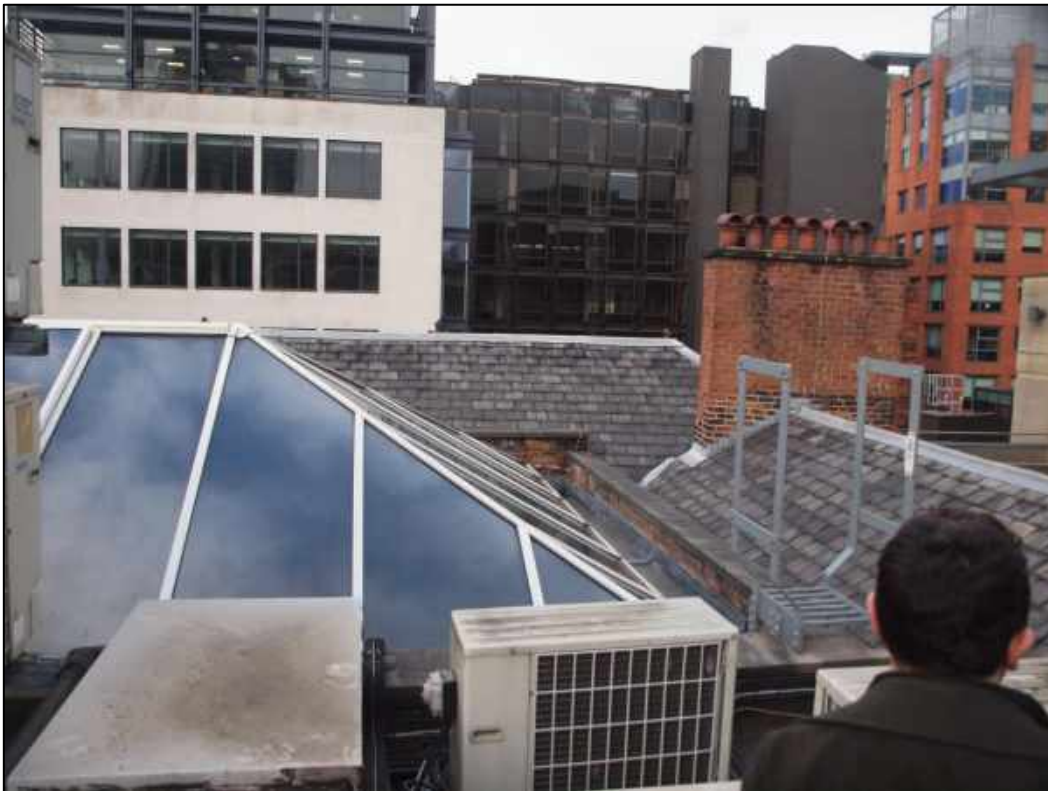
Plate 32: General view of the roof
