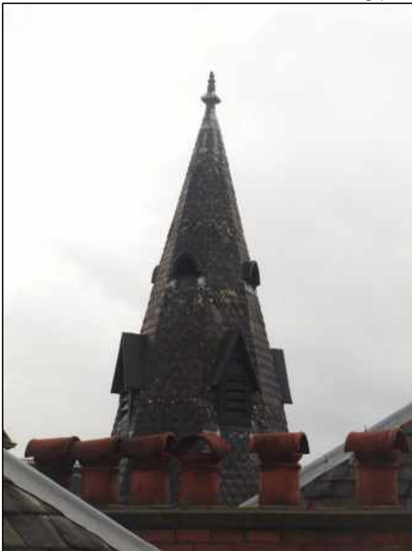
Plate 36: Shot of turret as viewed from the roof
