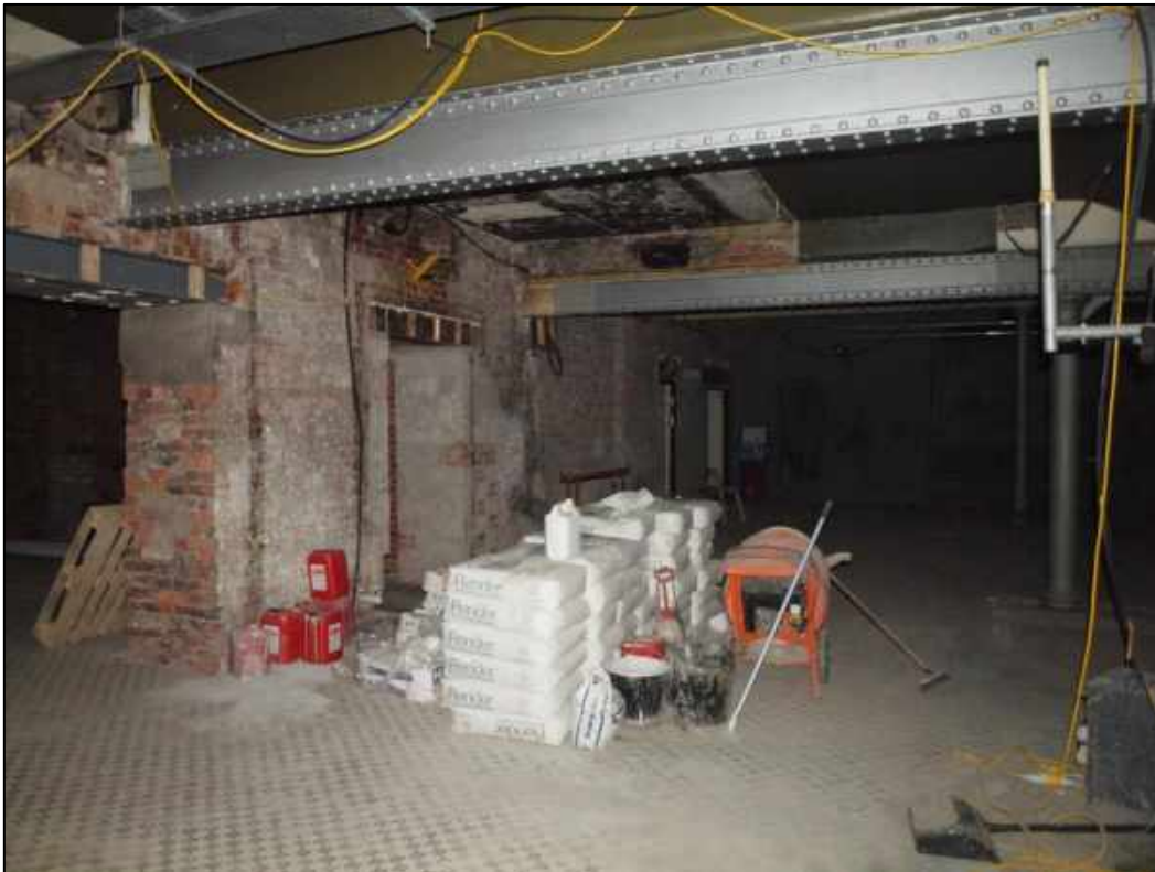
Plate 21: Inserted openings in north wall
