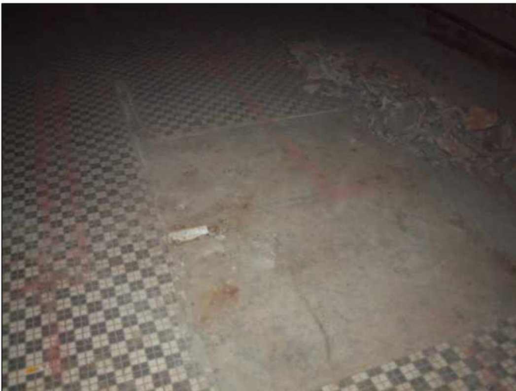
Plate 22: Modern flooring over concrete screed with modern pipe below
