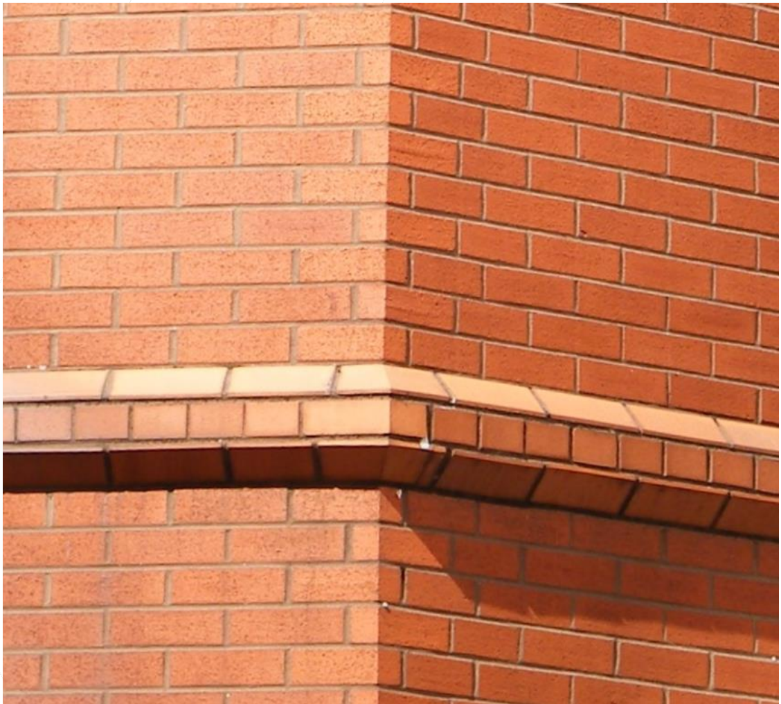
Fig.10: Angled brick band feature around the perimeter, HAD (2020).
