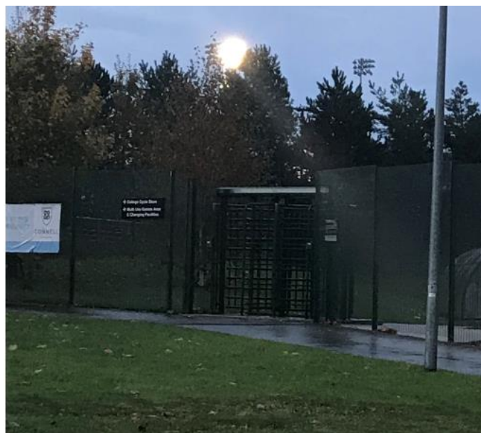
Access-controlled pedestrian turnstile - western aspect
