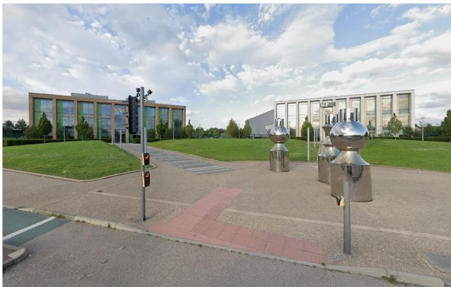
Connell Co-Op College (left) with MIHP building (right) with open area in foreground
