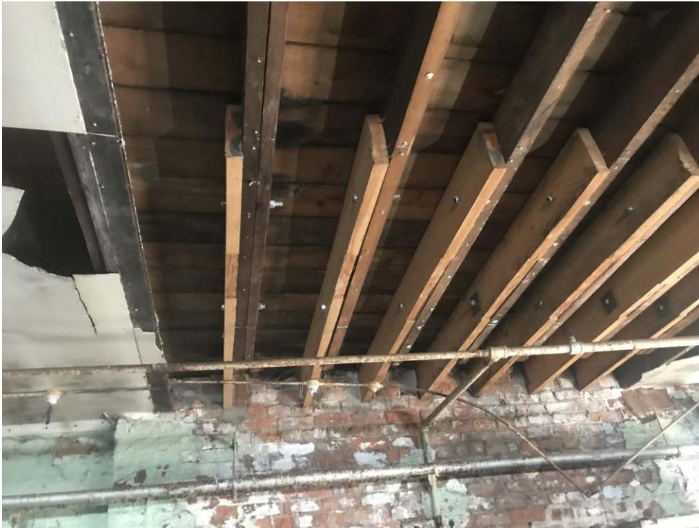
Photo 14 – Existing Splice Connection Detail to Roof
