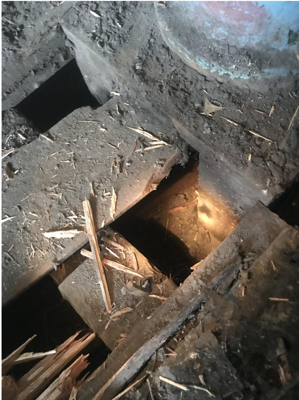
Photo 18 – Oblique Wrought Iron Member Bearing on Cast Iron Column at Second Floor
