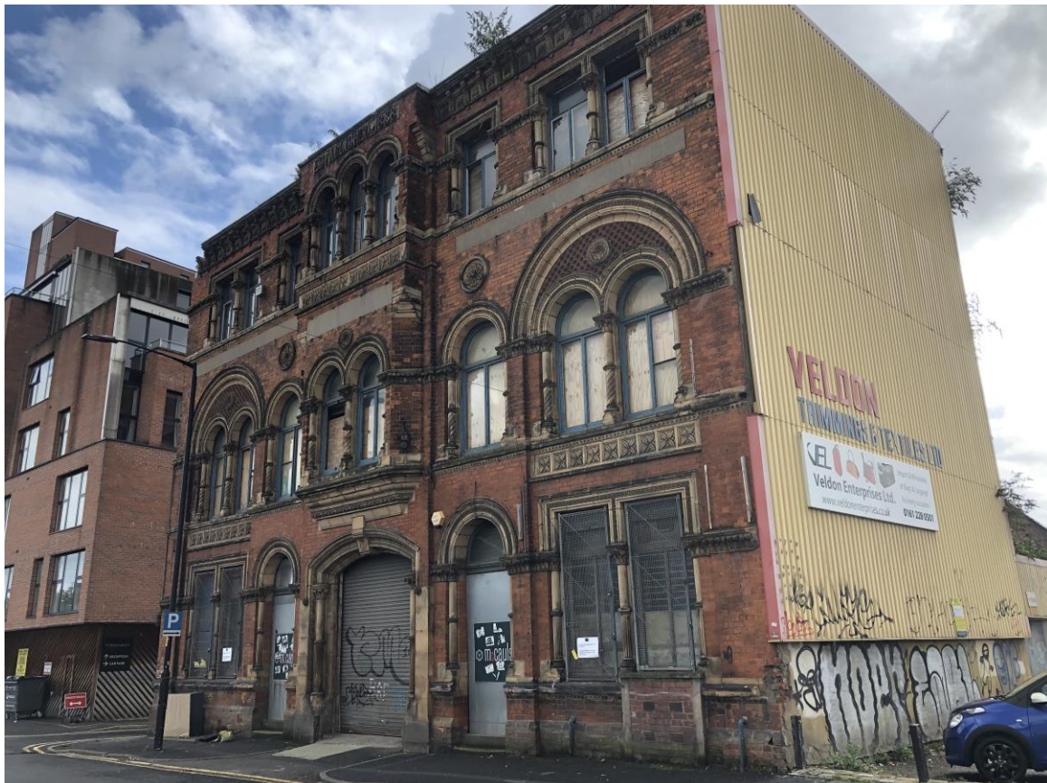
Photo 13 – Profiled Metal Cladding to Southwest Elevation
