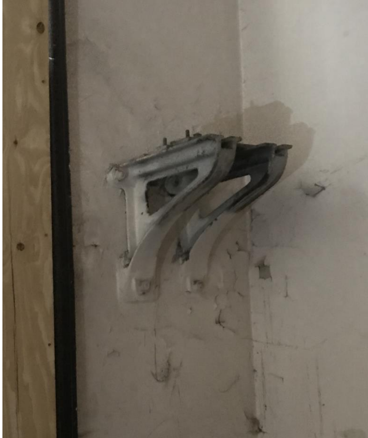
Photo 24 – Former Tank Stand in Northeast Building Corner
