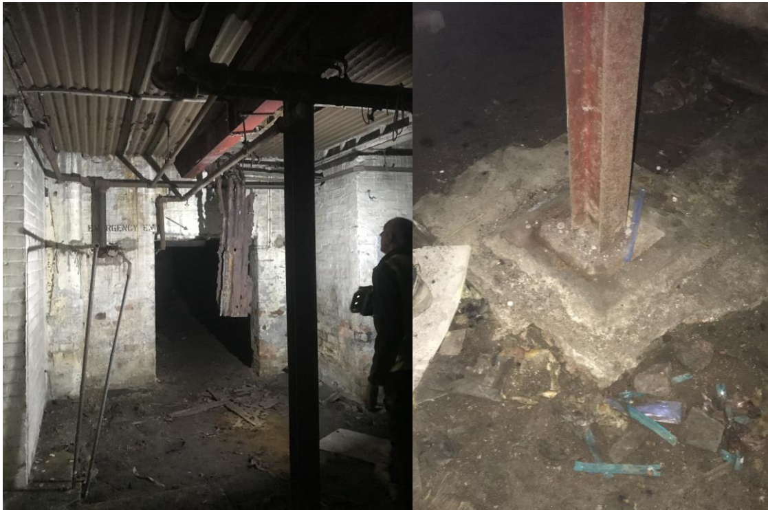
Photos 28 & 29 – Ground Floor Strengthening Works In Basement
