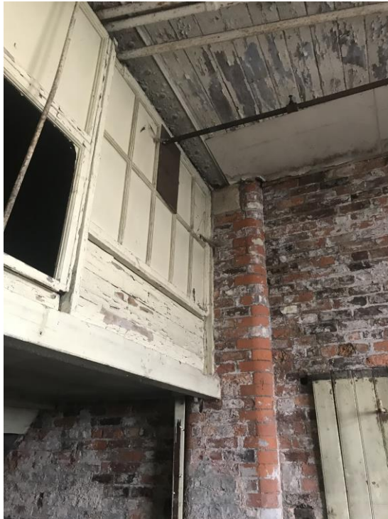
Photos 25 & 26 – Ground Floor Partial Mezzanine with Visible Riveted Beams
