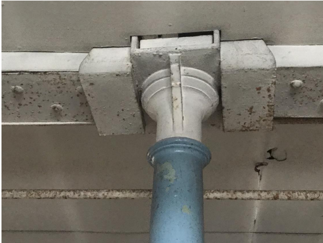
Photo 19 – Cast Support Brackets at Column Head Supporting Roof Members
