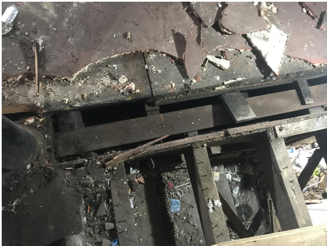
Photo 20 – Timber Infill to First Floor Stair Void and Original Trimmer Beam
