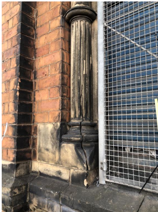
Photos 4 to 7 – Cracking to Terracotta Castings
