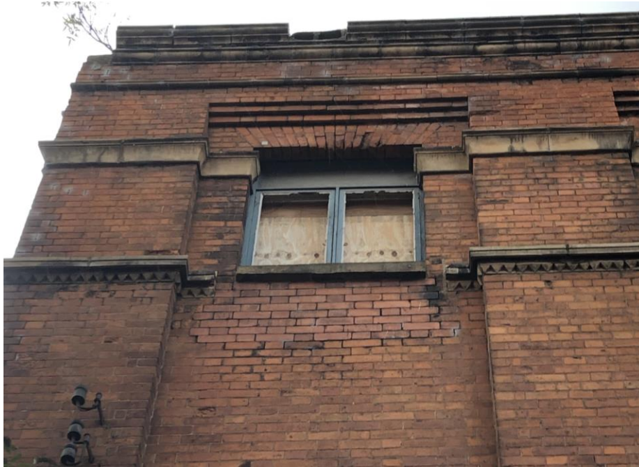
Photo 12 – Historic Loading Bay at Second Floor – Northeast Elevation
