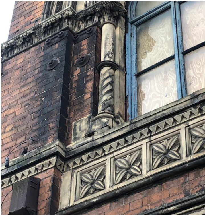
Photo 10 – External Spreader Plates on Northeast Building Corner
