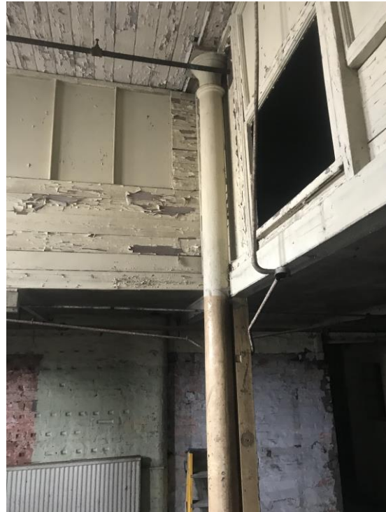
Photos 25 & 26 – Ground Floor Partial Mezzanine with Visible Riveted Beams
