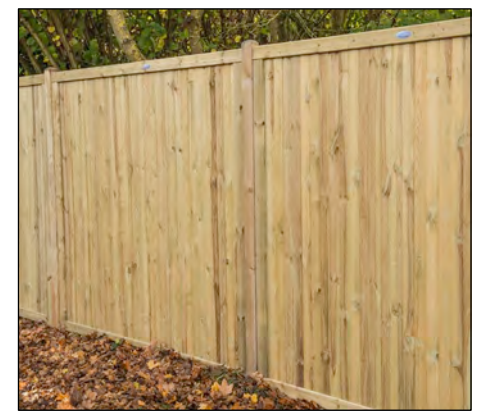
Close boarded timber acoustic fence to acousticians requirements. 3.0ms high.
