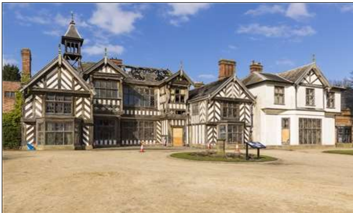
Figure 29 Wythenshawe Hall March 2016, after the fire.
