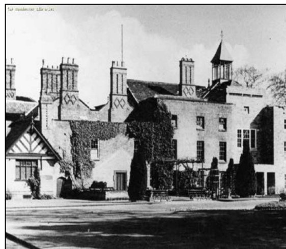
Figure 27 T Baddley, west of Wythenshawe Hall showing scarring (1952) © Manchester Libraries
