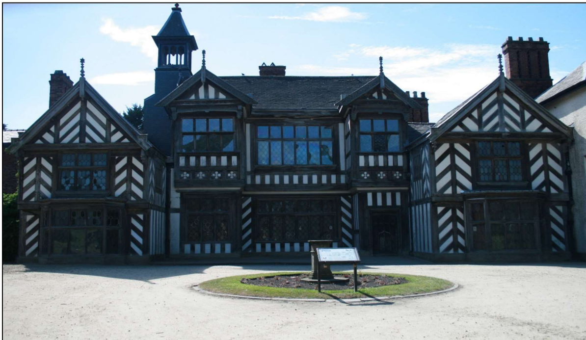
Figure 5 Hall Forecourt, before the fire, 2010.
