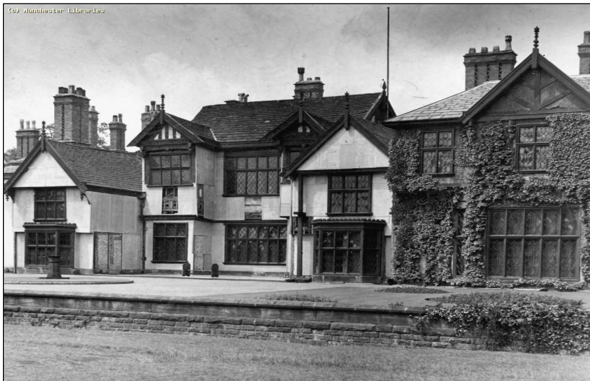
Figure 24 Wythenshawe Hall during repairs (1934) © Manchester Libraries
