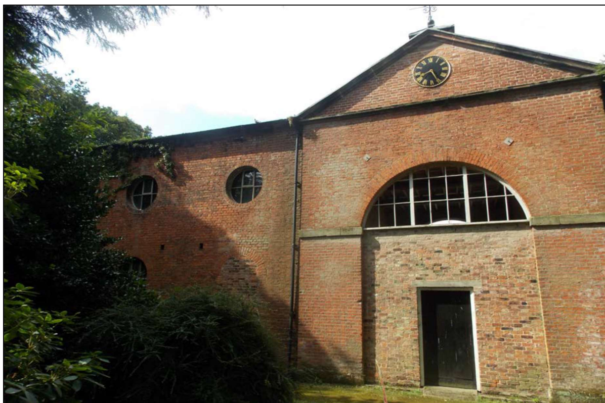
Figure 17 Former Stable Block, 2016.
