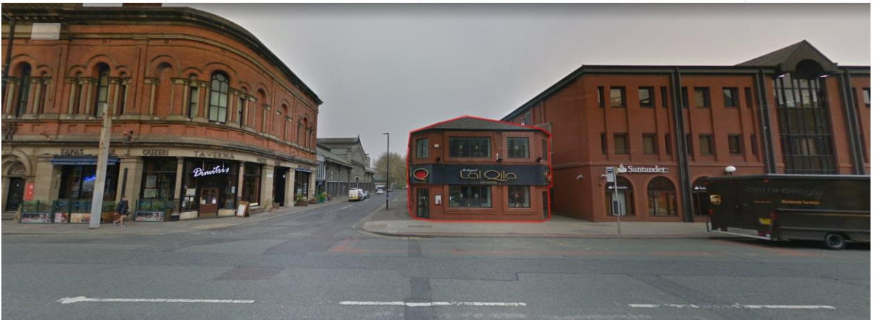
Deansgate view showing site, neighbouring buildings, and their various architectural styles. Site in red outline. Google Street (2019)
