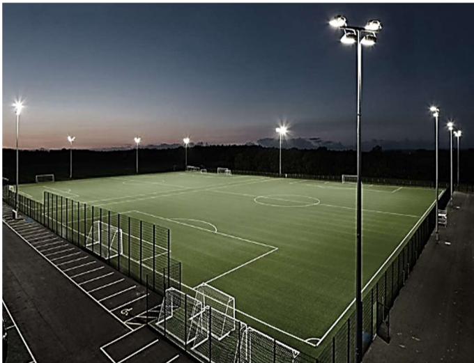
Typical 3G Artificial Grass Pitch (AGP) Installation
