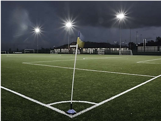
Typical 3G Artificial Grass Pitch (AGP) Installation
