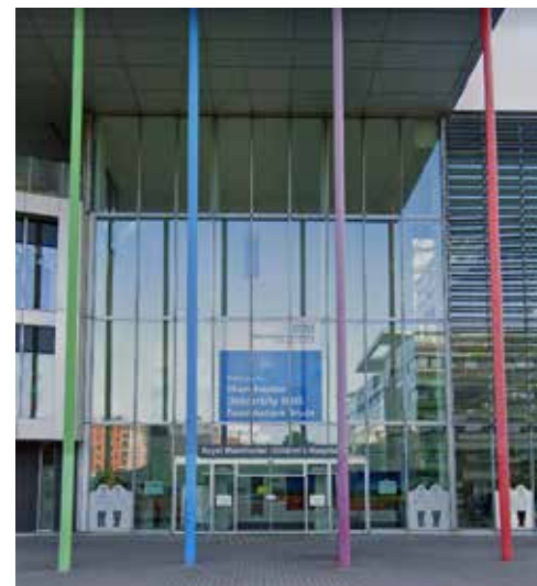
Children's Hospital Main Entrance
