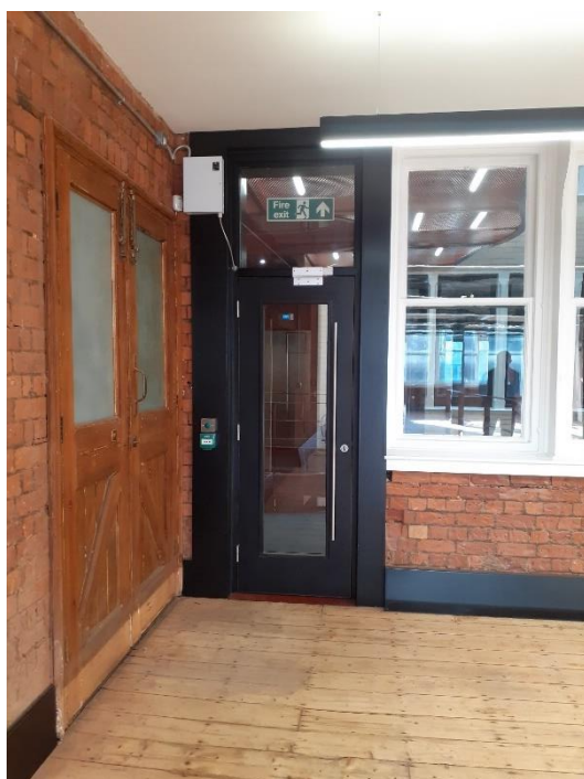
Image 7: Existing original timber doors, exposed brickwork, plasterboard ceiling and luminaries, modern partition and door
