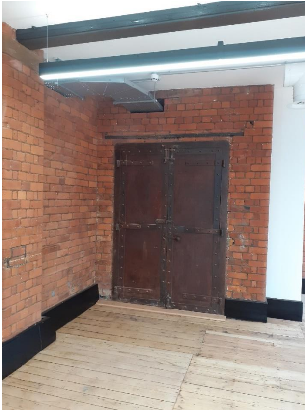
Image 8: Existing original brickwork, doors, beam and timber flooring, existing plasterboard ceiling, luminaire and mechanical services.
