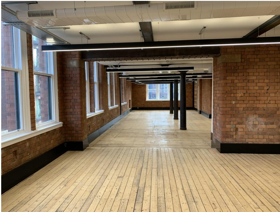
Image 10: Existing original brickwork, beams, columns and timber flooring, plasterboard ceiling, luminaires and mechanical services.
