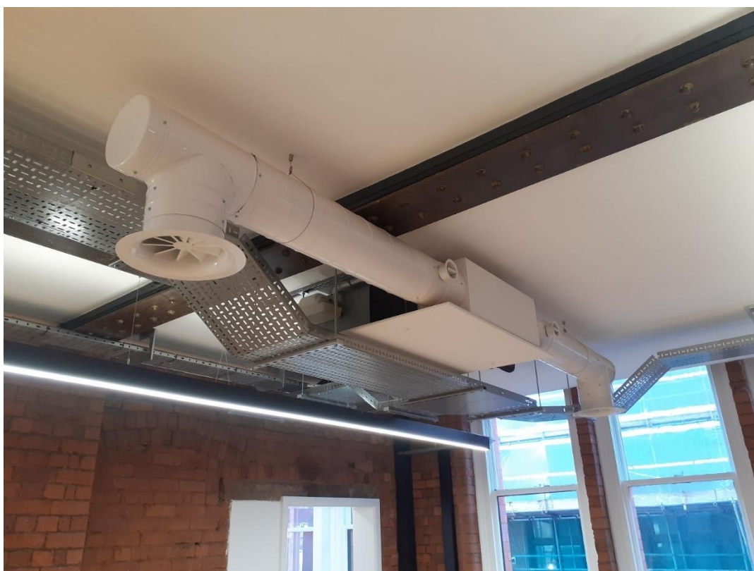
Image 6: Existing plasterboard ceiling, original beam, non-original mechanical services and luminaires.
