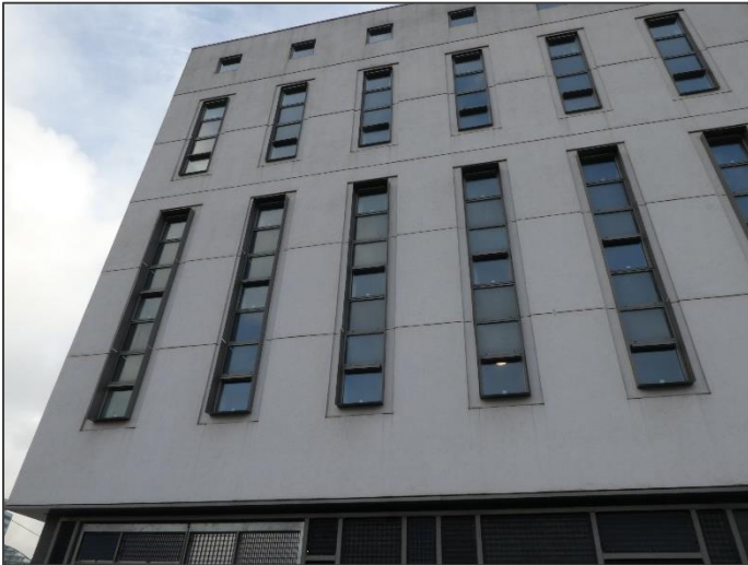
Photograph No. 1: Render system external view – North elevation
