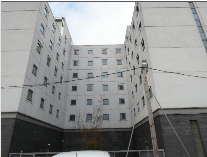
Photograph No. 2: Render system external view – South elevation
