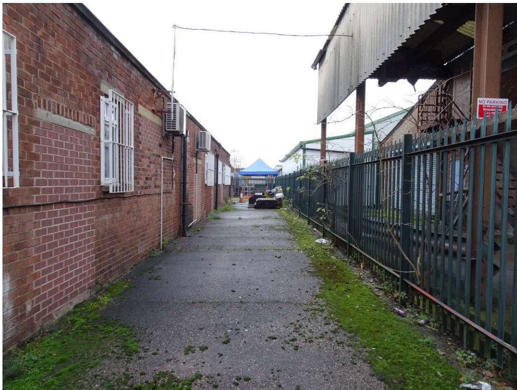
Photograph 4 – Side elevation (to be extended)
