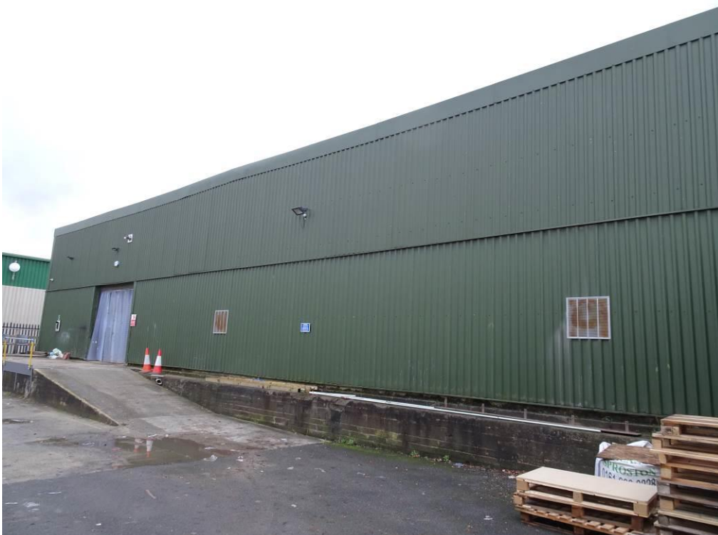
Photograph 2 – Side elevation and main vehicle access.
