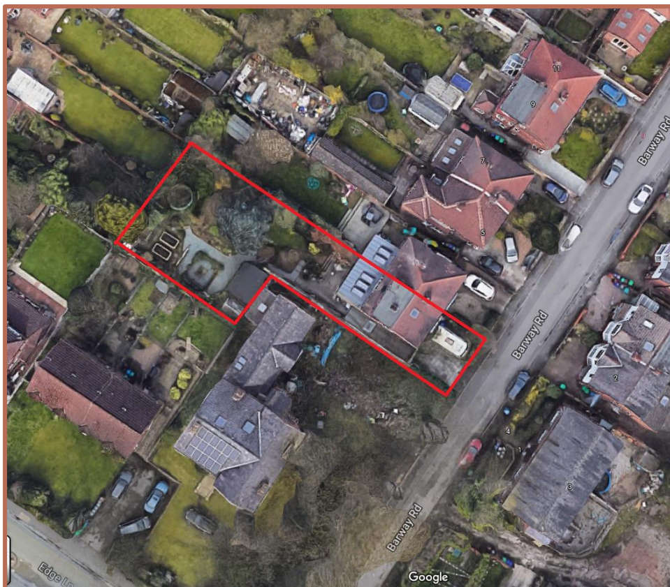
Figure 1: 1 Barway Road: Google Maps satellite imagery: Accessed March 2021
